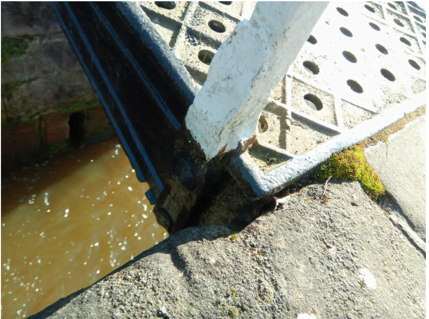
FIG 14A. A HEAVY HAMMER-WELD ON A LOCK-GATE BRIDGE LOCATED ON BOSLEY LOCK-FLIGHT. THE TOE IS CLEARLY DEFINED AND NO EFFORT HAS BEEN MADE TO BLEND IT. COPYRIGHTS BY ROWAN TAYLOR.
