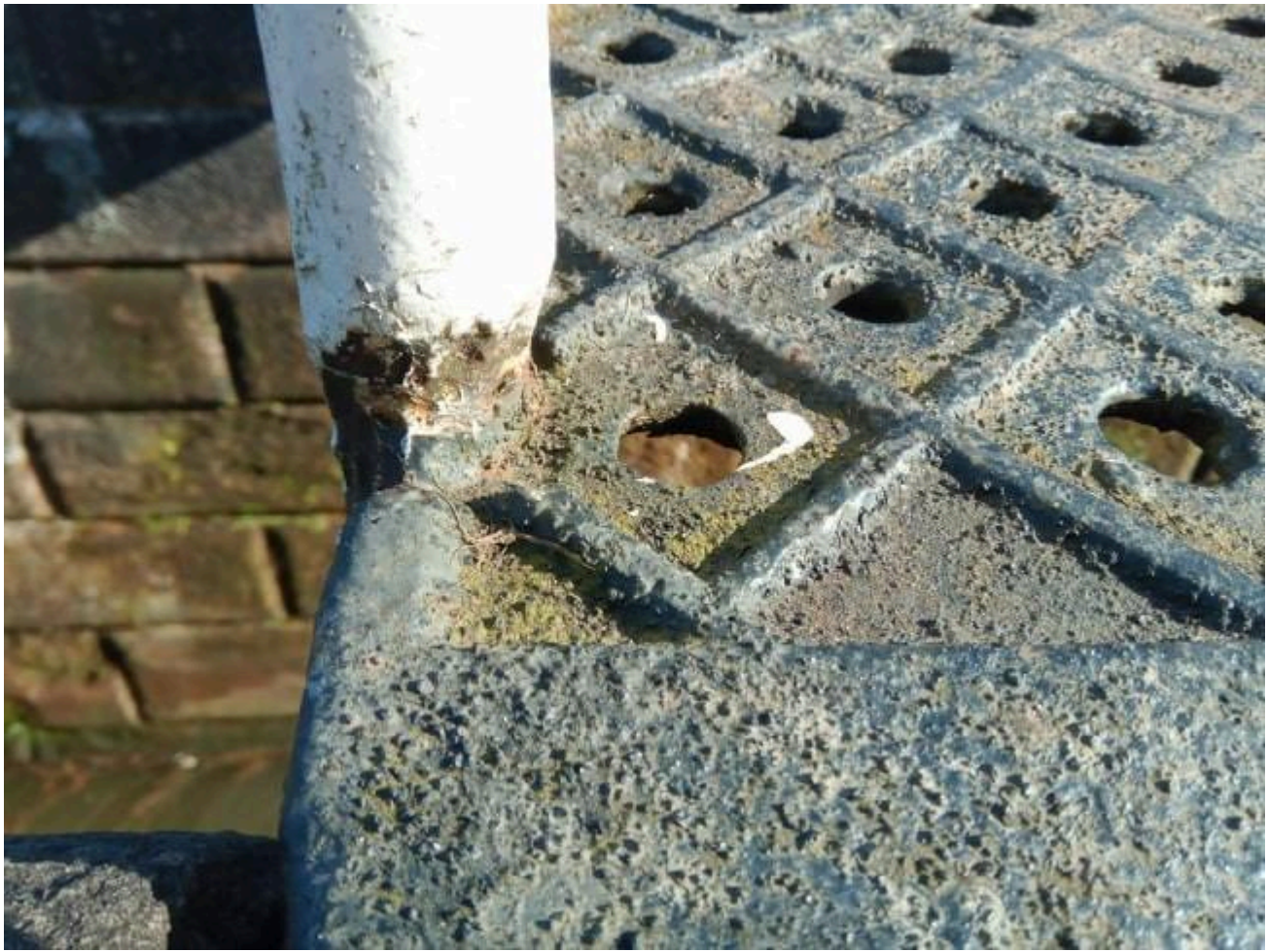
FIG 24B. EXAMPLES OF FOOTING CORROSION, SYMPTOMATIC OF AN ELECTROCHEMICAL IMBALANCE CAUSED BY THE PASSIVATION OF AN AREA OF IRONWORK. A - A WROUGHT IRON RIVET INCLUDED IN A CAST-IRON BALUSTER. THE BASE OF A HANDRAIL WHERE THE REAR OF THE FOOT IS BOLTED TO A CAST IRON BRIDGE. COPYRIGHTS BY ROWAN TAYLOR
