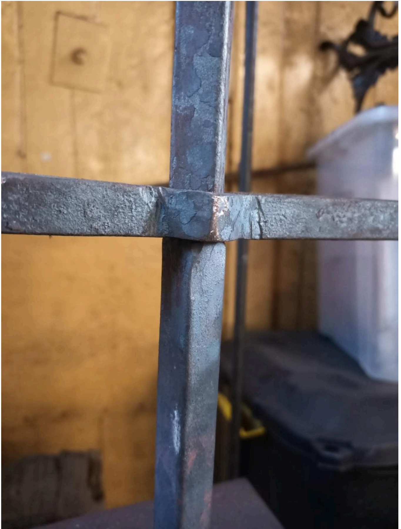
FIG 28A. PRACTICAL DEMONSTRATION OF A TWIST BEING USED TO FORM A STEP IN A SHAFT. THIS PRODUCES AN IMPEDANCE ON THE SHAFT SUFFICIENT TO THE RETENTION OF A PASS-THROUGH FIXING. ADDITIONALLY, THE SHAFT APPEARS EITHER BROADER ABOVE OR BELOW THE TWIST DEPENDING ON WHERE THE VIEWER STANDS. COPYRIGHTS BY ROWAN TAYLOR.
