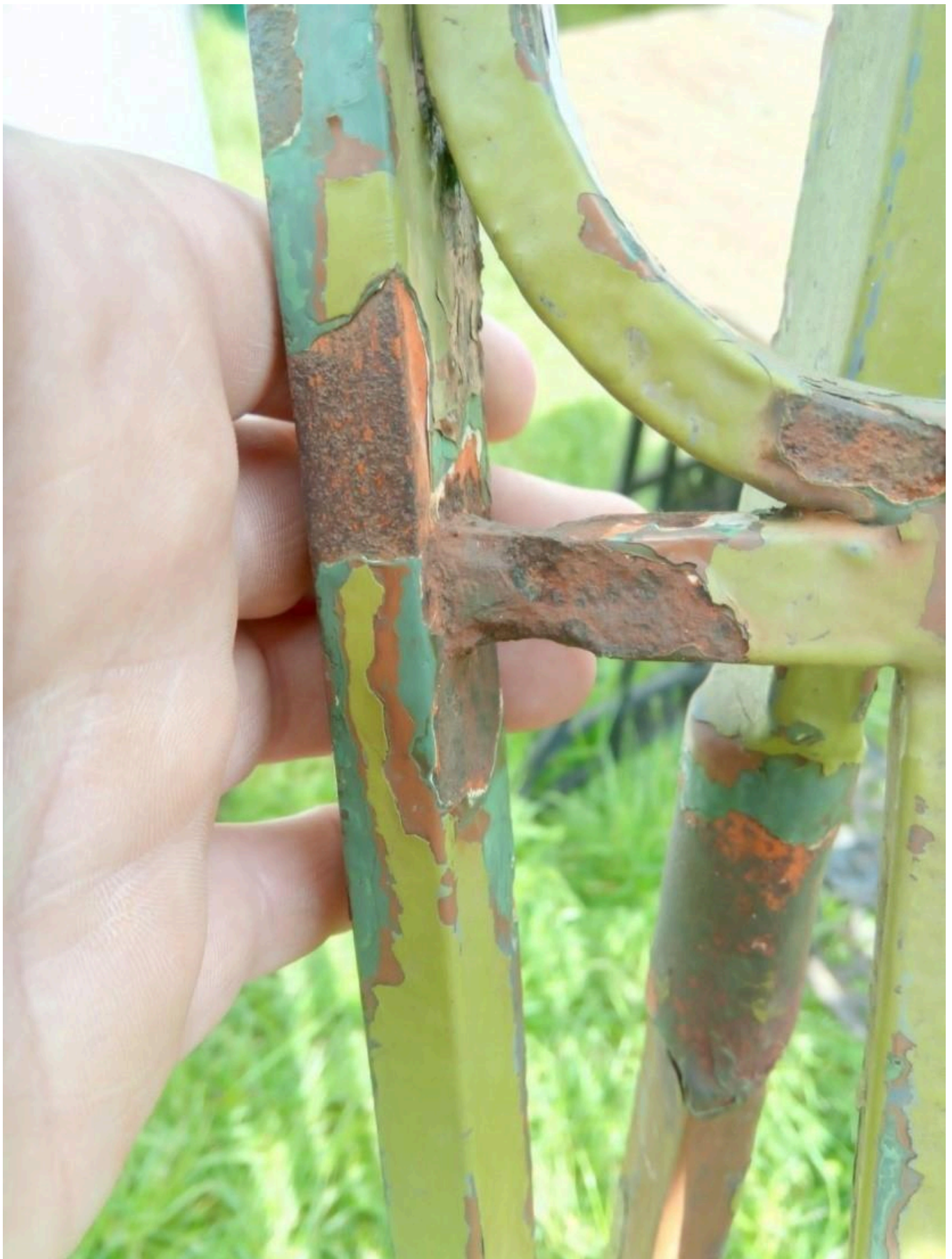
FIG 24E. EXAMPLES OF FOOTING CORROSION, SYMPTOMATIC OF AN ELECTROCHEMICAL IMBALANCE CAUSED BY THE PASSIVATION OF AN AREA OF IRONWORK. A - A WROUGHT IRON RIVET INCLUDED IN A CAST-IRON BALUSTER. SMALL GATE AT AN ANTIQUES FAIR, DEMONSTRATING FOOTING CORROSION ABOVE A MORTICE-AND-TENNON JOINT. WHILE THE FOOTING CORROSION IS HORIZONTAL IN THIS INSTANCE, THE GATE WAS LIKELY STORED ON ITS SIDE FOR AN EXTENDED PERIOD. COPYRIGHTS BY ROWAN TAYLOR
