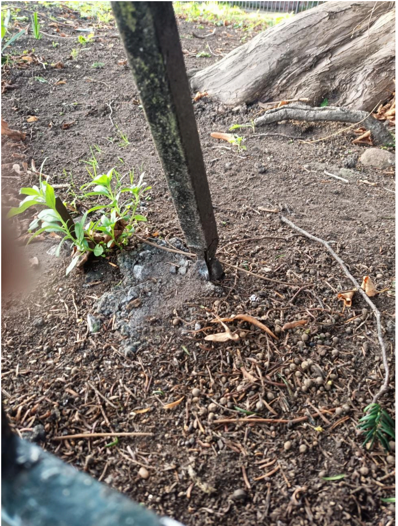
FIG 24C. EXAMPLES OF FOOTING CORROSION, SYMPTOMATIC OF AN ELECTROCHEMICAL IMBALANCE CAUSED BY THE PASSIVATION OF AN AREA OF IRONWORK. A - A WROUGHT IRON RIVET INCLUDED IN A CAST-IRON BALUSTER. STANCHION ON A CHURCH RAILING, FIXED INTO CONCRETE. COPYRIGHTS BY ROWAN TAYLOR
