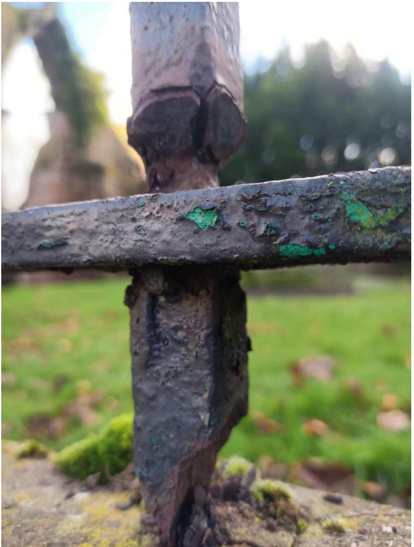
FIG 24D. EXAMPLES OF FOOTING CORROSION, SYMPTOMATIC OF AN ELECTROCHEMICAL IMBALANCE CAUSED BY THE PASSIVATION OF AN AREA OF IRONWORK. A - A WROUGHT IRON RIVET INCLUDED IN A CAST-IRON BALUSTER. UPRIGHT ON A CHURCH RAILING DEMONSTRATING FOOTING CORROSION BOTH ABOVE THE BASE AND ABOVE A PASS-THROUGH FIXING. COPYRIGHTS BY ROWAN TAYLOR
