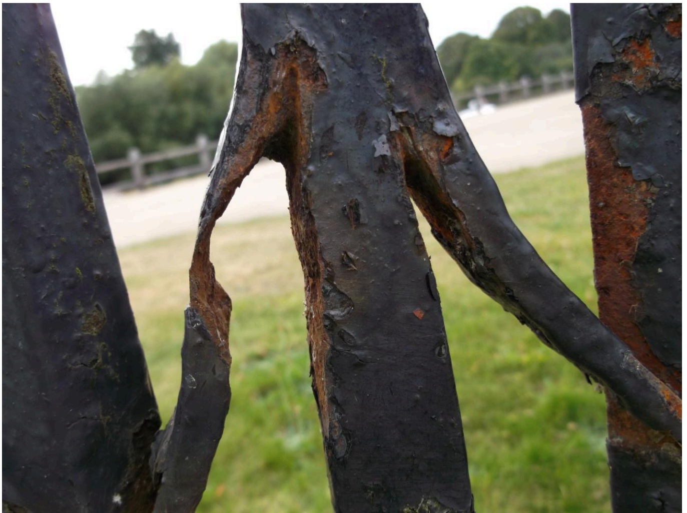
FIG 13B. THE SAME BRANCH-WELD AFTER REMOVAL OF THE CORROSION PRODUCT WHICH WAS CAUSING DAMAGE. GIVEN A PERIOD OF FIVE TO TEN YEARS, THE LOWER PART OF THE ELEMENT WOULD HAVE BECOME DETACHED, RESULTING IN A FORM SIMILAR TO THE POINT B SWELLING OF THE IRON STAND. IMAGE BY THE AUTHOR, SHARED COURTESY OF THE NHIG.
