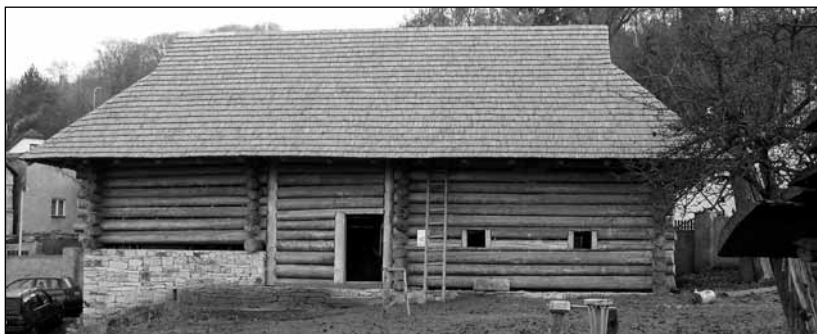
Fig. 27 Building of a three part house B1: view from the park grounds at the finished rough building with a shingle roof. ■
