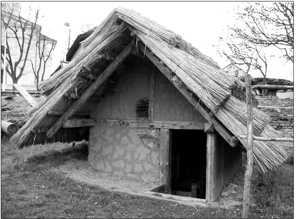
Fig. 19 Finished experimental construction of the structure B7. ■
