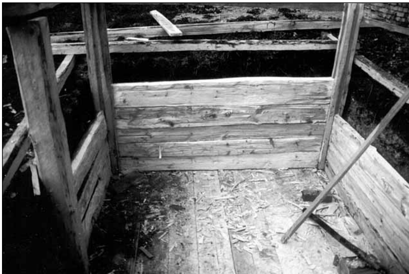
Fig. 11 Experimental building of structure B7: rebated construction in the subsurface part. ■
