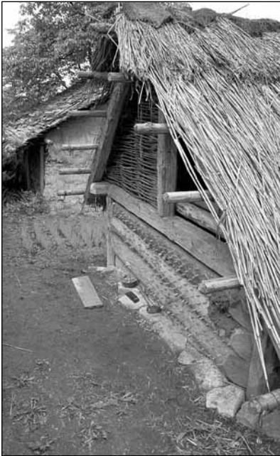
Fig. 16 Experimental building of structure B7: preparation of the rear wall for daubing. ■
