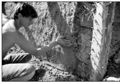
Fig. 18 Experimental building of structure B7: daubing. ■
