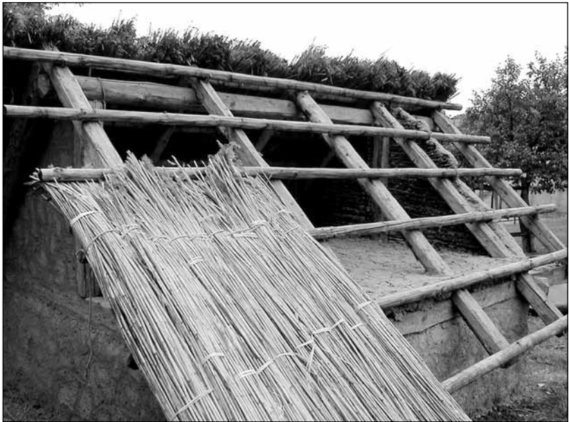
Fig. 15 Experimental building of structure B7: the daubed platform ceiling. ■
