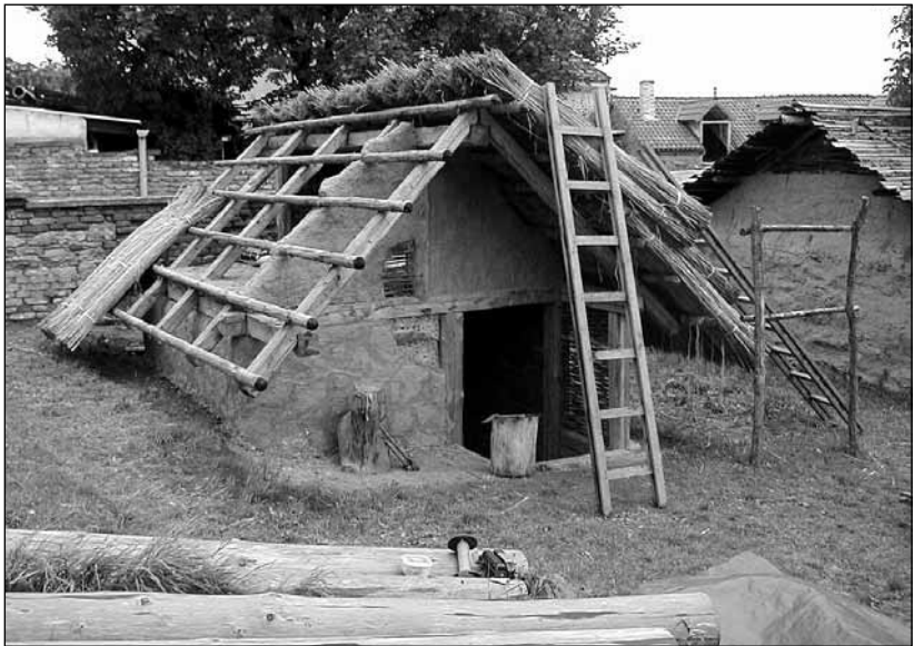
Fig. 13 Experimental building of structure B7 before finishing. ■
