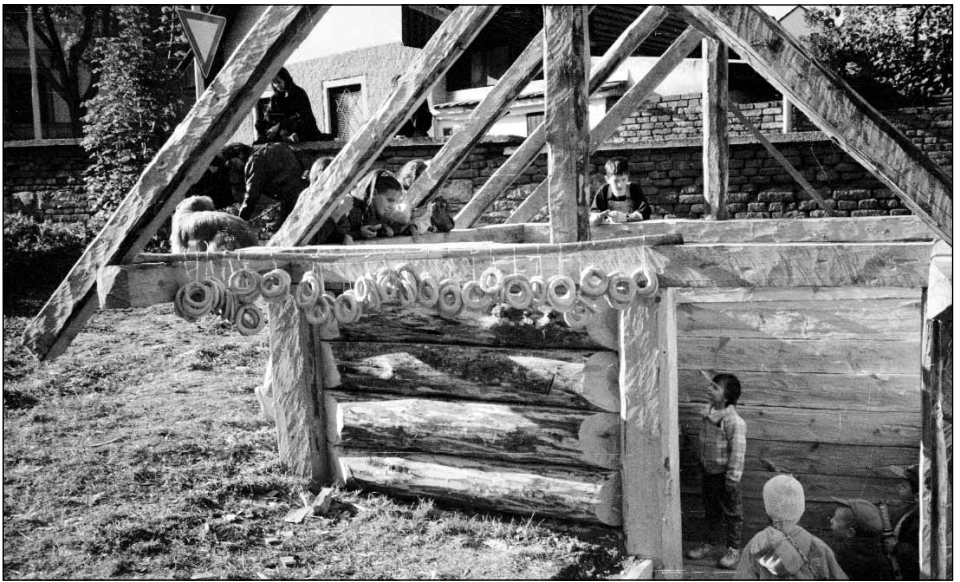
Fig. 12 Experimental building of structure B7: rough construction with a roof frame. ■
