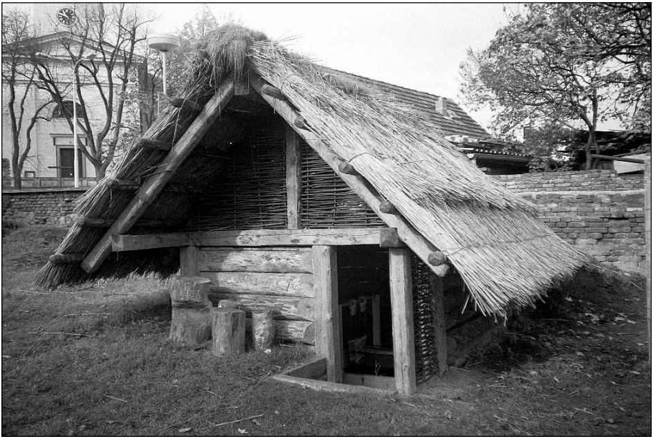
Fig. 14 Experimental building of structure B7: finished building before daubing. ■
