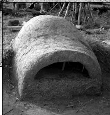
Fig. 11 Construction of a one-chamber kiln. ■
