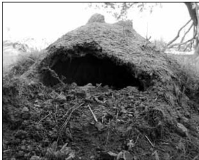
Fig. 37 (right) Destruction of the vault of the one-chamber kiln firebox; there is a visible difference between the fired and non-fired layers of daub in the section of the cover. ■ Fig. 43 (left) Weathered outer surface of the cover of the one-chamber kiln. ■
