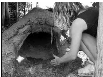
Fig. 30 Repair of the horizontal kiln. ■
