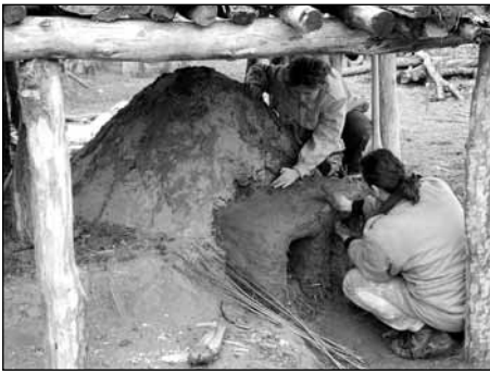
Fig. 31 Adaptation of the vertical two-chamber kiln to second version. ■
