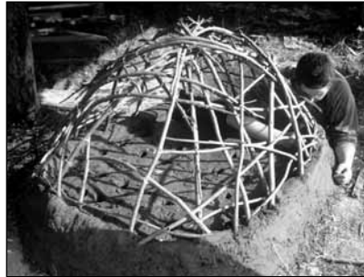
Fig. 29 Construction of the cover of the vertical two-chamber kiln. ■
