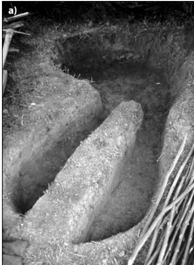
Fig. 28 Construction of channels of a grate and b vertical kiln. ■
