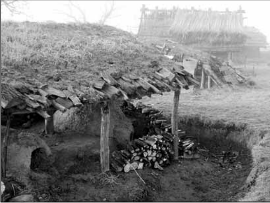
Fig. 42 Shelter over the kilns. ■
