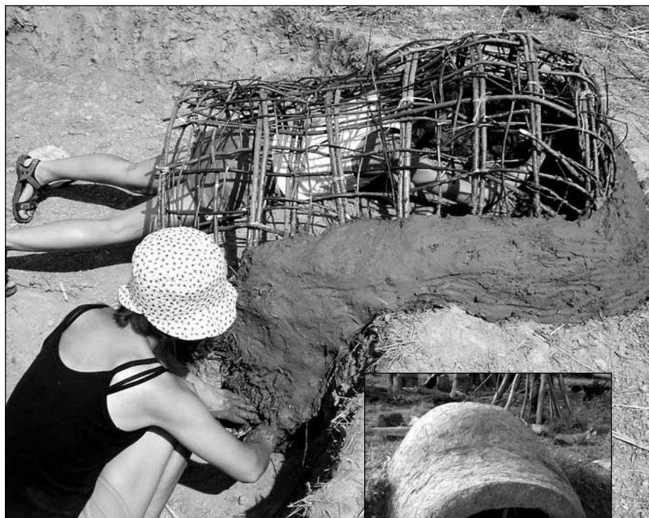
Fig. 12 Building of a one-chamber kiln. ■
