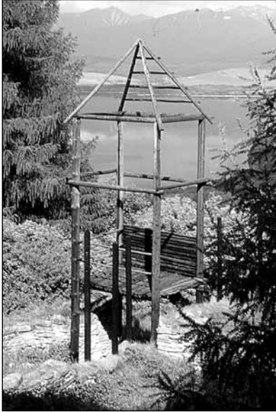
Fig. 1 Condition of the tower in 2000. ■
