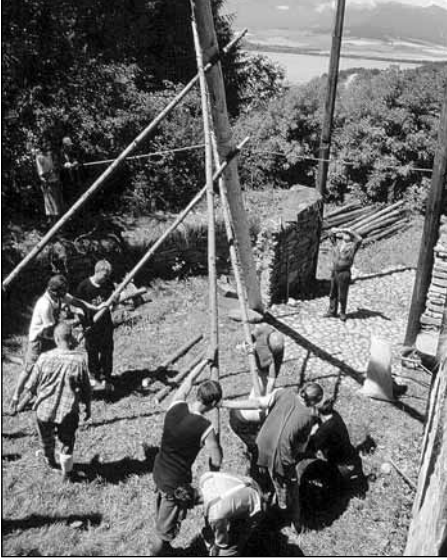
Fig. 7 Erecting a new post. ■
