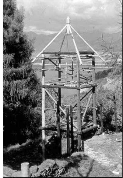
Fig. 3 Condition of the tower in autumn 2003. ■
