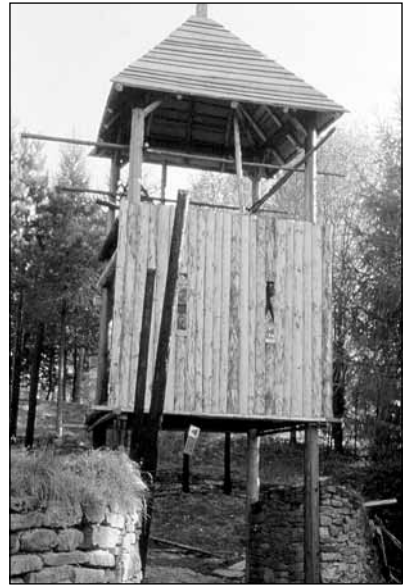
Fig. 10 Putting on the covering under supervision. ■
