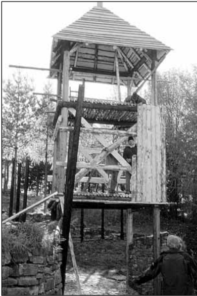
Fig. 8 Horizontal strengthening of the tower at floor level. ■
