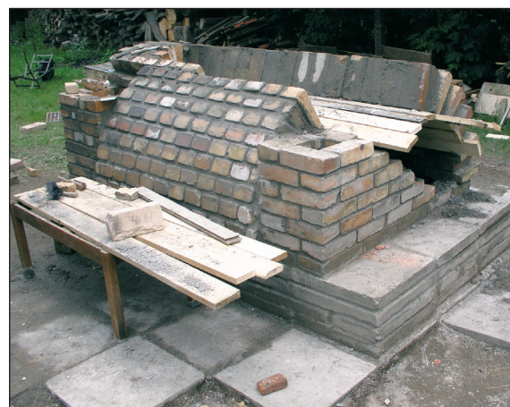
■ Fig. 11 Building of a kiln for baking of impure potash in the garden area of the Muzeum in Deštné v Orlických horách.
