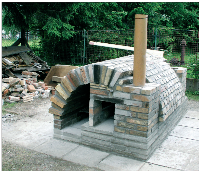
■ Fig. 12 Kiln for baking of potash. (all photo of production of potash J. Woitsch)
