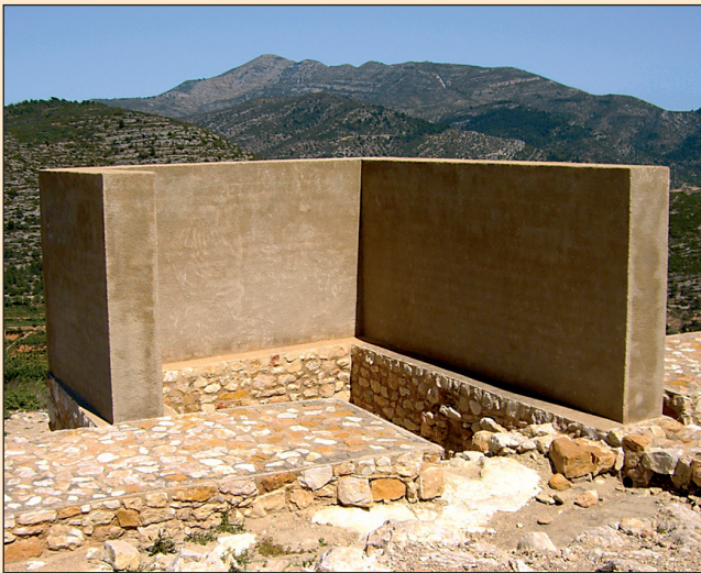
■ Fig. 6 Iberian village of Moleta del Remei (Alcanar, Tarragona), wall made by concrete above the original one.
