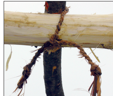
■ Fig. 9 Binding of the houses beam with lime bast.
