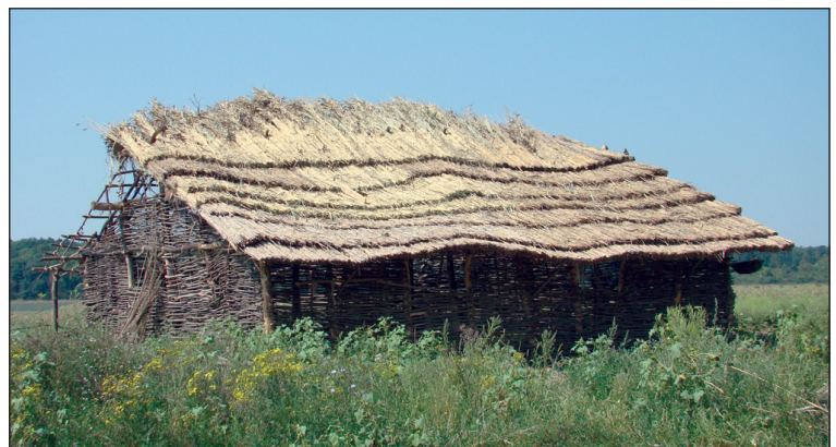
■ Fig. 22 Reed roof, general view.
