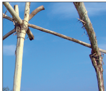
■ Fig. 17 Binding of construction elements with flaxen rope.
