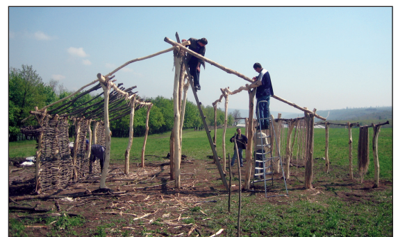
■ Fig. 11 Fix the lateral beams.
