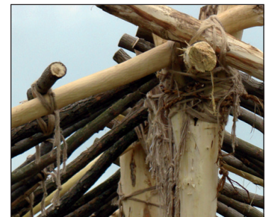
■ Fig. 18 Binding of construction elements with flaxen rope with lime bast.
