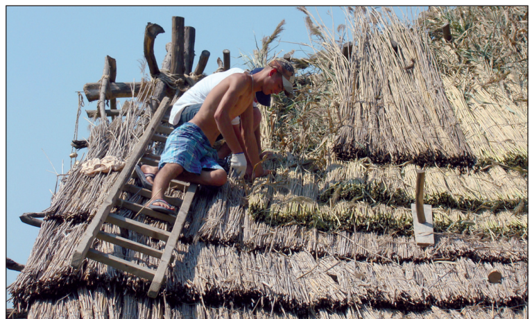
■ Fig. 20 Roof arrangement with reed.
