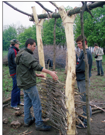
■ Fig. 14 Walls plaited with twigs.
