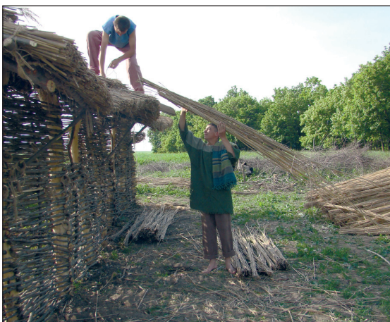
■ Fig. 21 Coverage of the house with reed.
