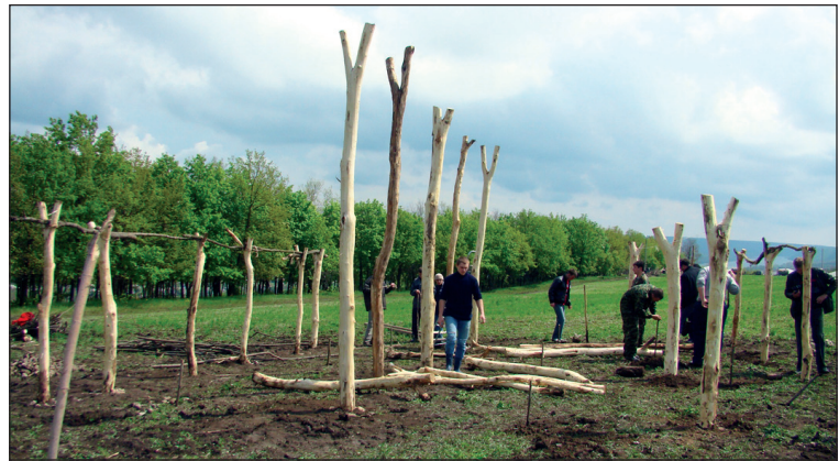
■ Fig. 4 Central trunks for roof strengthening.
