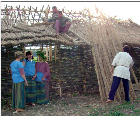
■ Fig. 19 Final aspect of the house's wooden construction, south view.
