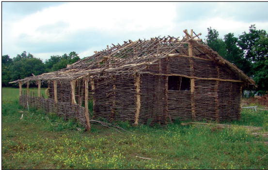
■ Fig. 16 Final aspect of the house's wooden construction, north-eastern view.
