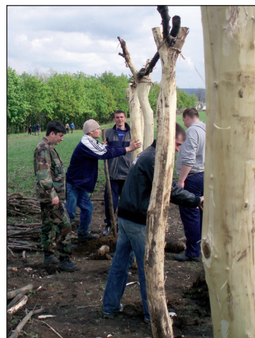
■ Fig. 7 Strengthening of external trunks of the house.
