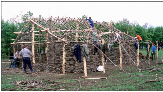
■ Fig. 13 Fix the roof's lateral trunks of the house and wall plait with branches.
