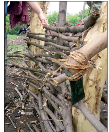
■ Fig. 15 Walls plaited with branches.
