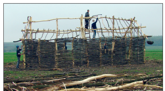
■ Fig. 12 Fix the roof's lateral trunks of the house.
