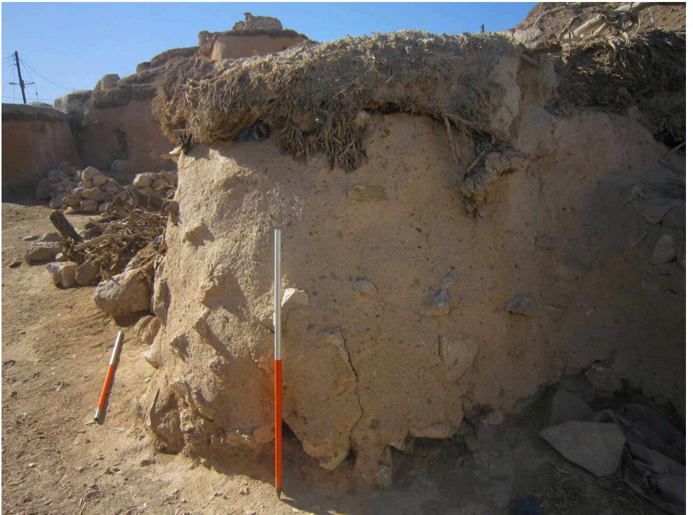
FIG 8. STONE MATERIALS AND THATCH. PHOTO BY TAHERE RAHIMKHANI.
