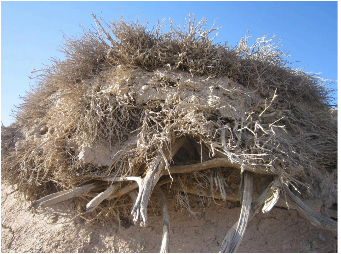
FIG 9A. WINDBLOWN THORNS TO PREVENT RAIN FROM PENETRATING THE ROOF. PHOTO BY TAHERE RAHIMKHANI.
