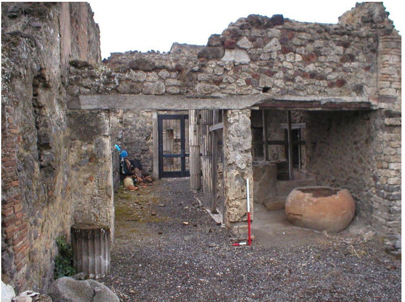
FIG 4. POMPEII, PROPERTY I VIII 19. THE ROOF IS MODERN REINFORCED CONCRETE THAT HAS BEEN POORLY MAINTAINED. PHOTO: ROB JANAWAY
