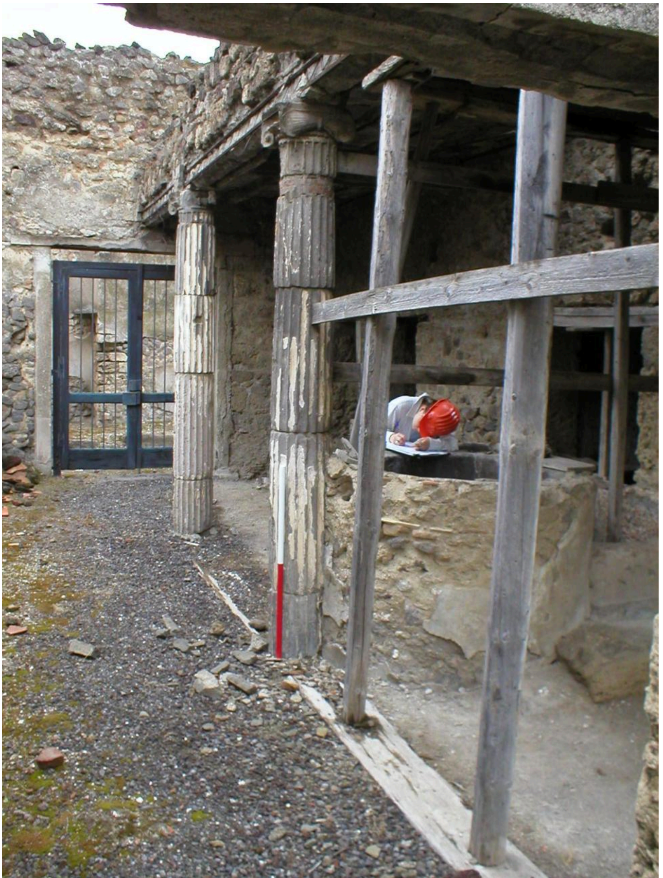
FIG 6. THE ORIGINAL REMAINS, AN UNKNOWN AMOUNT OF CONCRETE RESTORATION OF UNKNOWN AGE, PROPS FOR THE MODERN ROOF THAT IS COLLAPSING STRAIGHT ON TO THE ORIGINAL REMAINS. PHOTO: ROB JANAWAY
