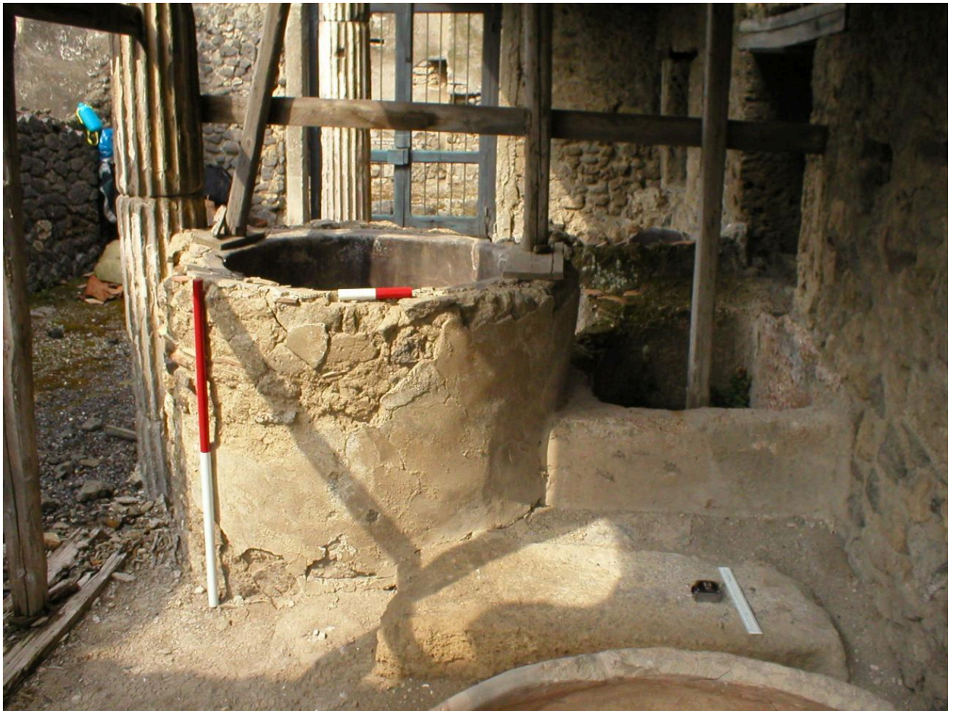
FIG 3. VAT 5, PROPERTY IVIII19, SHOWING PROPS SUPPORTING POORLY MAINTAINED RECONSTRUCTED ROOF RESTING ON ORIGINAL ROMAN APPARATUS, THEREBY DAMAGING IT. AS THE RECONSTRUCTION DECAYS IT IS NOT POSSIBLE TO DISCERN THE ORIGINAL AND MODERN.
