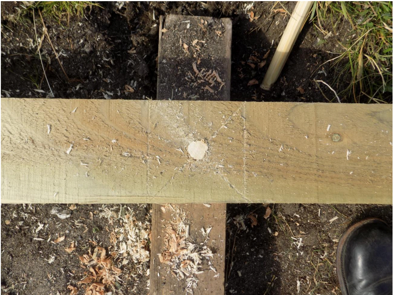
FIG 17. THE SECOND METHOD TO TRIM THE TRENAILS WAS USING AN ADZE. THIS LEFT MORE OF A STUMP; WAS LESS NEAT THAN A SAW; AND CREATED MORE WASTE MATERIAL. PHOTO BY ANTHONY DAWSON.
