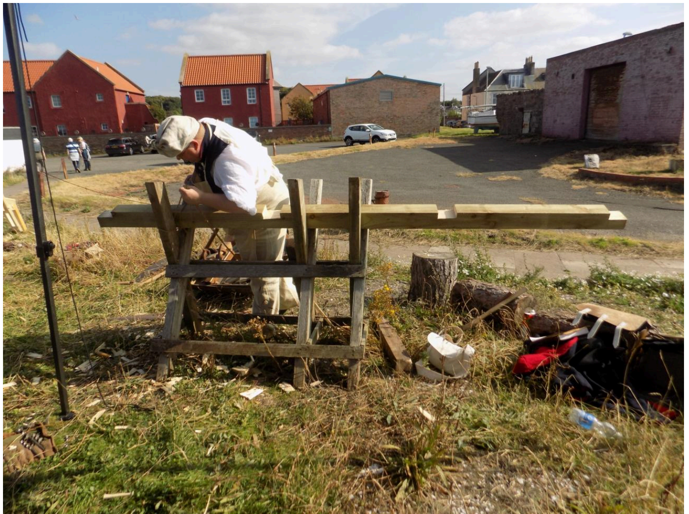
FIG 20. CUTTING HALF LAP JOINTS IN THE RAILS BY HAND. EACH JOINT TOOK ONE INDIVIDUAL 30 MINUTES TO CUT, A MORE EXPERIENCED JOINER MAY HAVE TAKEN LESS TIME. IT IS LIKELY RAILS WERE PREPARED OFF-SITE. PHOTO BY ANTHONY DAWSON.
