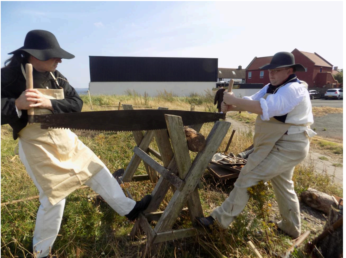
FIG 9. CUTTING ROUND WIND-FALL SLEEPERS TO LENGTH. SLEEPERS WERE CUT TO ONE AND A HALF TIMES THE GAUGE. PHOTO BY ANTHONY DAWSON.
