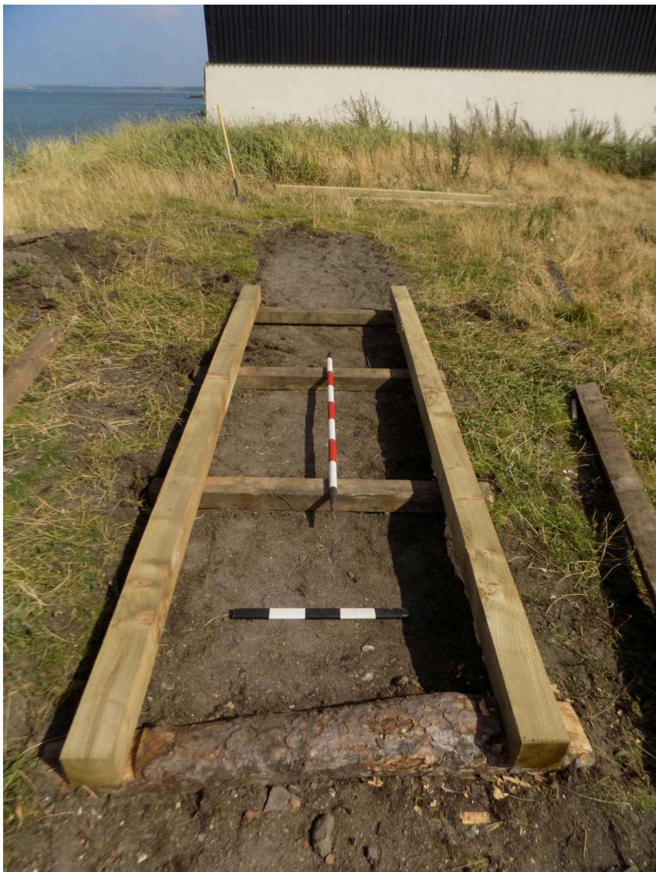
FIG 14. SLEEPERS AND RAILS IN SITU, PRIOR TO DRILLING OF HOLES FOR TRENAILS AND BALLASTING. BUILDING SUCH A RAILWAY REQUIRED THE MINIMAL AMOUNT OF TOOLS OR SKILLS. PHOTO BY ANTHONY DAWSON.
