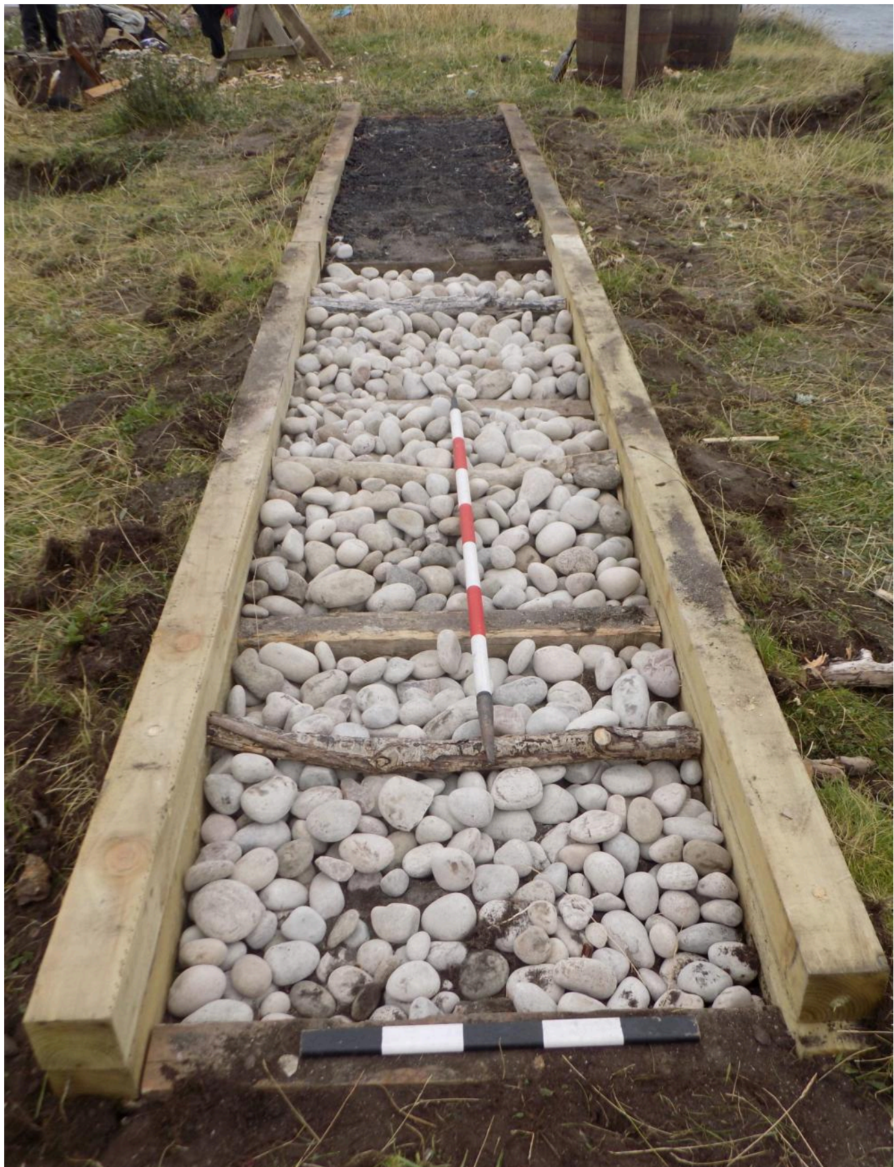
FIG 23. THE UPPER OR RUNNING RAILS SECURED IN POSITION, AND BALLASTED WITH BROKEN STONE AND COBBLES. ALSO EVIDENT ARE THE INTERMEDIATE SLEEPERS SUGGESTED BY THE ARCHAEOLOGY. PHOTO BY ANTHONY DAWSON.
