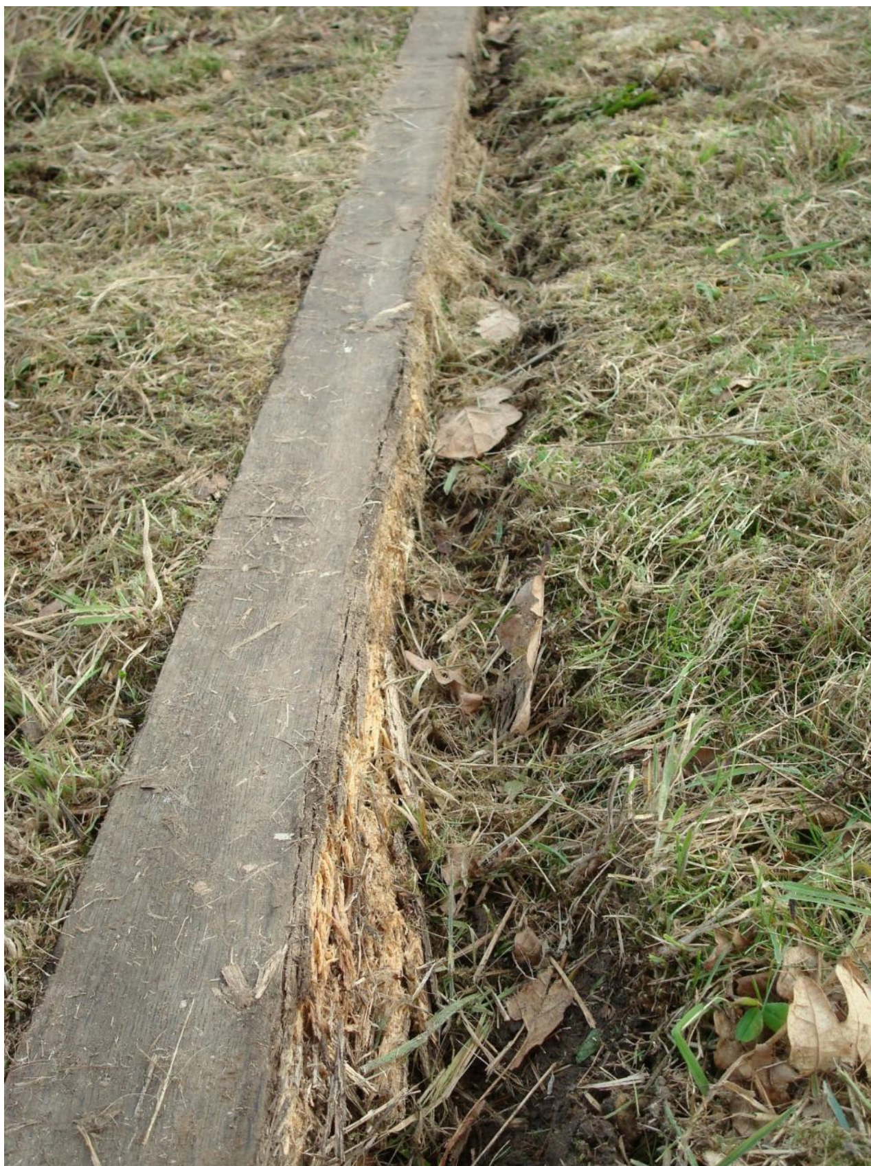
FIG 8. THE WHEEL AND IN PARTICULARLY THE FLANGE OF THE IRON WHEELS DAMAGED THE INSIDE FACE OF THE RAILS. THE RAILS WERE CRUSHED BY THE WEIGHT AND SHAPE OF THE WHEELS, AND THE FLANGE RUBBING AGAINST THE INSIDE FACE OF THE RAIL CAUSE CONSIDERABLE DAMAGE. THIS SUGGESTS LATER 18TH CENTURY WROUGHT-IRON STRIPS ON TOP OF THE RAIL WERE PERHAPS EITHER IN THE WRONG PLACE, OR REINFORCED THE EDGE, RAISING THE WHEEL SUFFICIENTLY SO THAT THE CONED TREAD RAN MORE HAPPILY ON THE STRIP OF IRON AND ALSO RAISED THE FLANGE SO THAT IT DIDN'T DAMAGE THE INSIDE OF THE RAIL. PHOTO BY PAUL JARMAN, BEAMISH MUSEUM.
