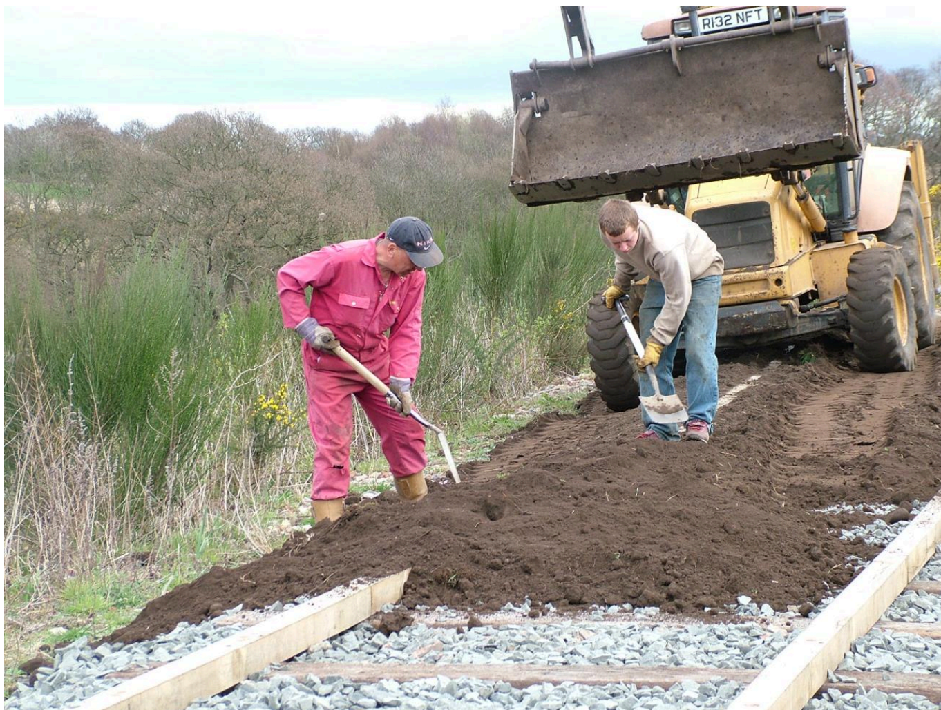
FIG 6. THE BEAMISH REPLICA WAS BALLASTED BY MACHINE. IN ORDER TO RESPECT THE LANDOWNERS WISHES NO DITCHES WERE DUG BUT IT WAS SECURELY FENCED OFF. PHOTO BY PAUL JARMAN, BEAMISH MUSEUM.
