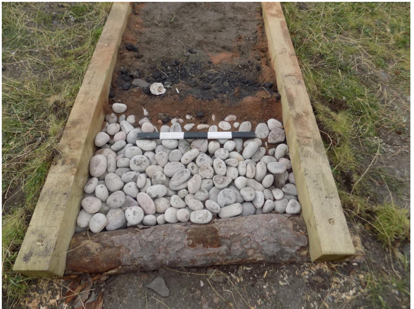
FIG 19. SMALL COAL, ASHES, CLINKER AND SPOIL FROM THE DITCHES WAS USED TO CREATE THE WALKING SURFACE OF THE HORSE TRACK. THIS WAS TRAMPLED UNDER FOOT AND RAMMED USING TIMBER POSTS TO MAKE THE FINAL SURFACE. PHOTO BY ANTHONY DAWSON.
