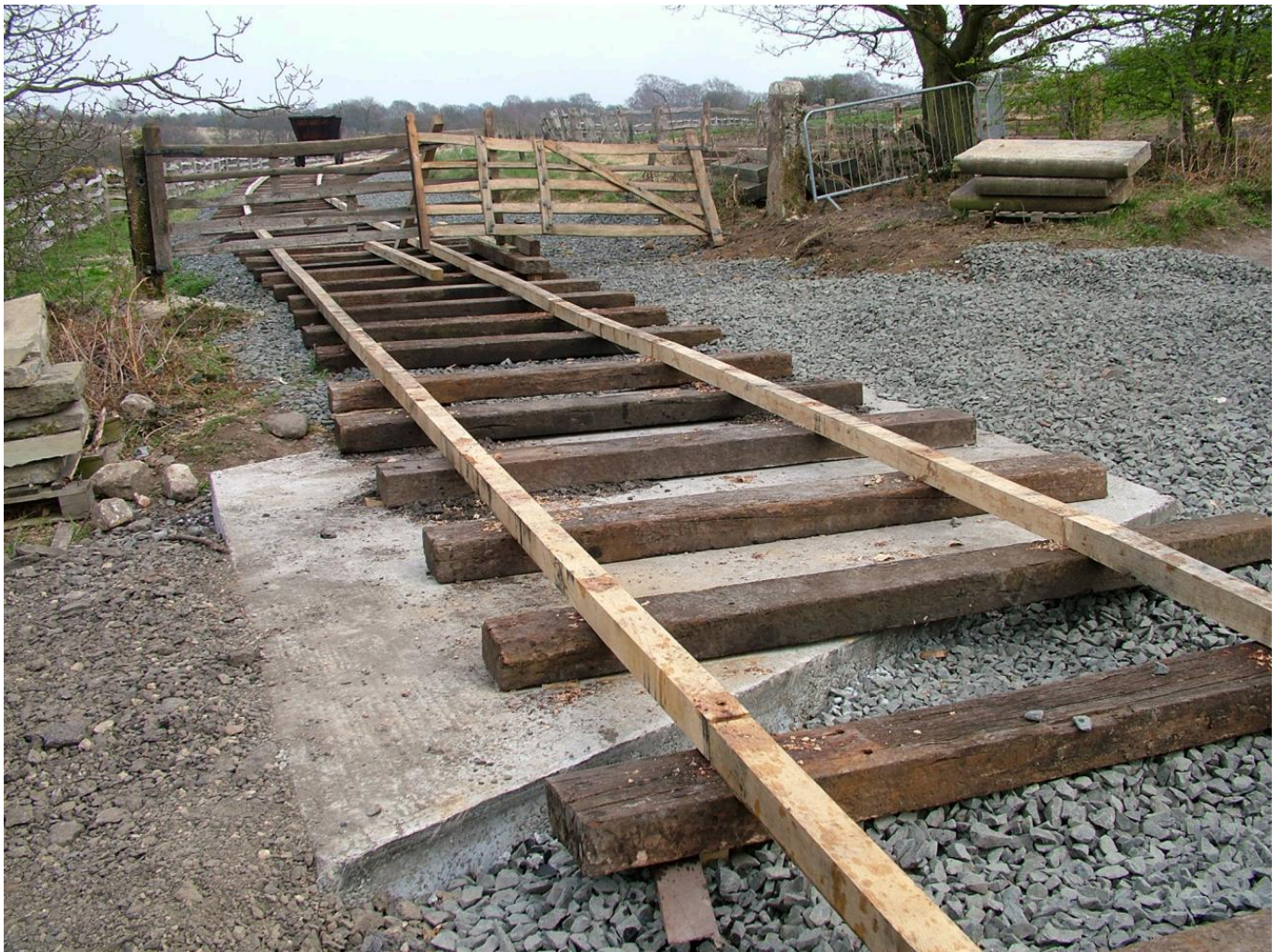
FIG 5. CONSTRUCTION OF THE REPLICA WOODEN WAGGONWAY AT BEAMISH WHICH USED A MIXTURE OF MODERN MATERIALS (SUCH AS SLEEPERS AND PRE-SAWN OAK TIMBER) BUT ALSO TRADITIONAL METHODS SUCH AS DRILLING TRENAIL HOLES BY HAND. PHOTO BY PAUL JARMAN, BEAMISH MUSEUM.
