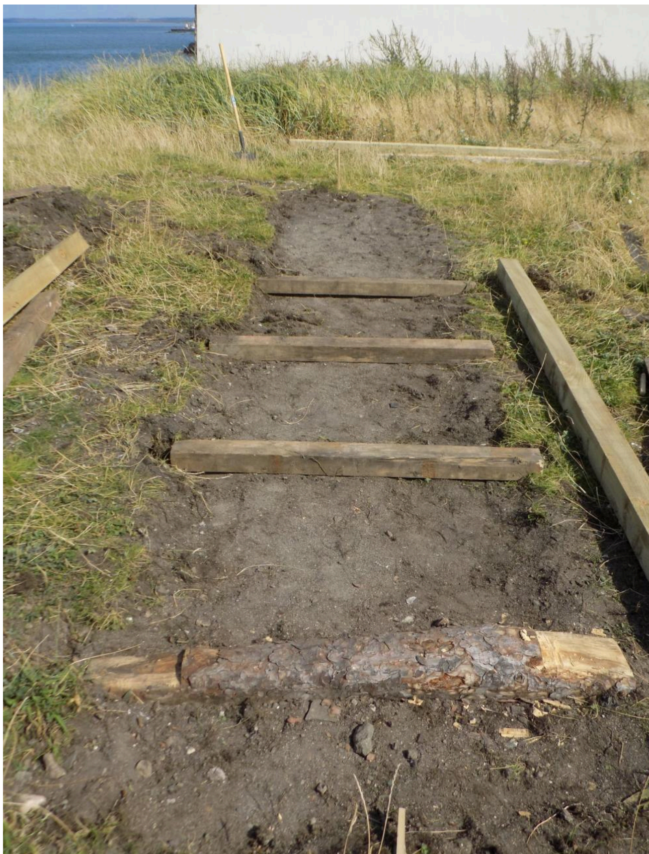
FIG 13. ROUND TIMBER SLEEPER HALF BURIED AND LEVELLED IN THE EARTH WITH FOUR MACHINE-FINISHED SLEEPERS ROUGHLY IN SITU. PHOTO BY ANTHONY DAWSON.
