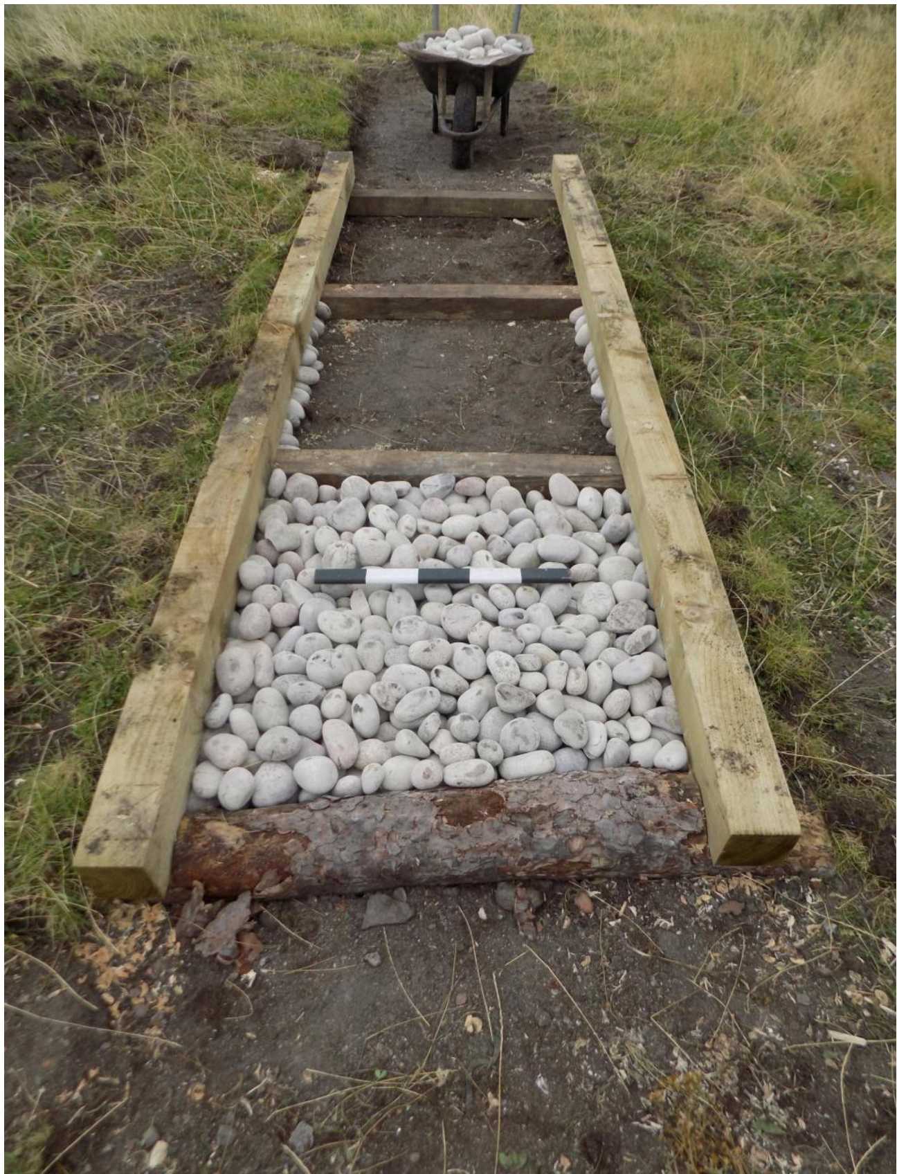
FIG 18. EACH 'COMPARTMENT' FORMED BY THE RAIL AND SLEEPER REQUIRED TWO MODERN BARROW LOADS OR APPROXIMATELY 180LITRES OF COBBLES AND BROKEN STONE TO FILL IT. THIS WAS THEN RAMMED AND PACKED WITH SPOIL TO CREATE A SOLID FOUNDATION. PHOTO BY ANTHONY DAWSON.
