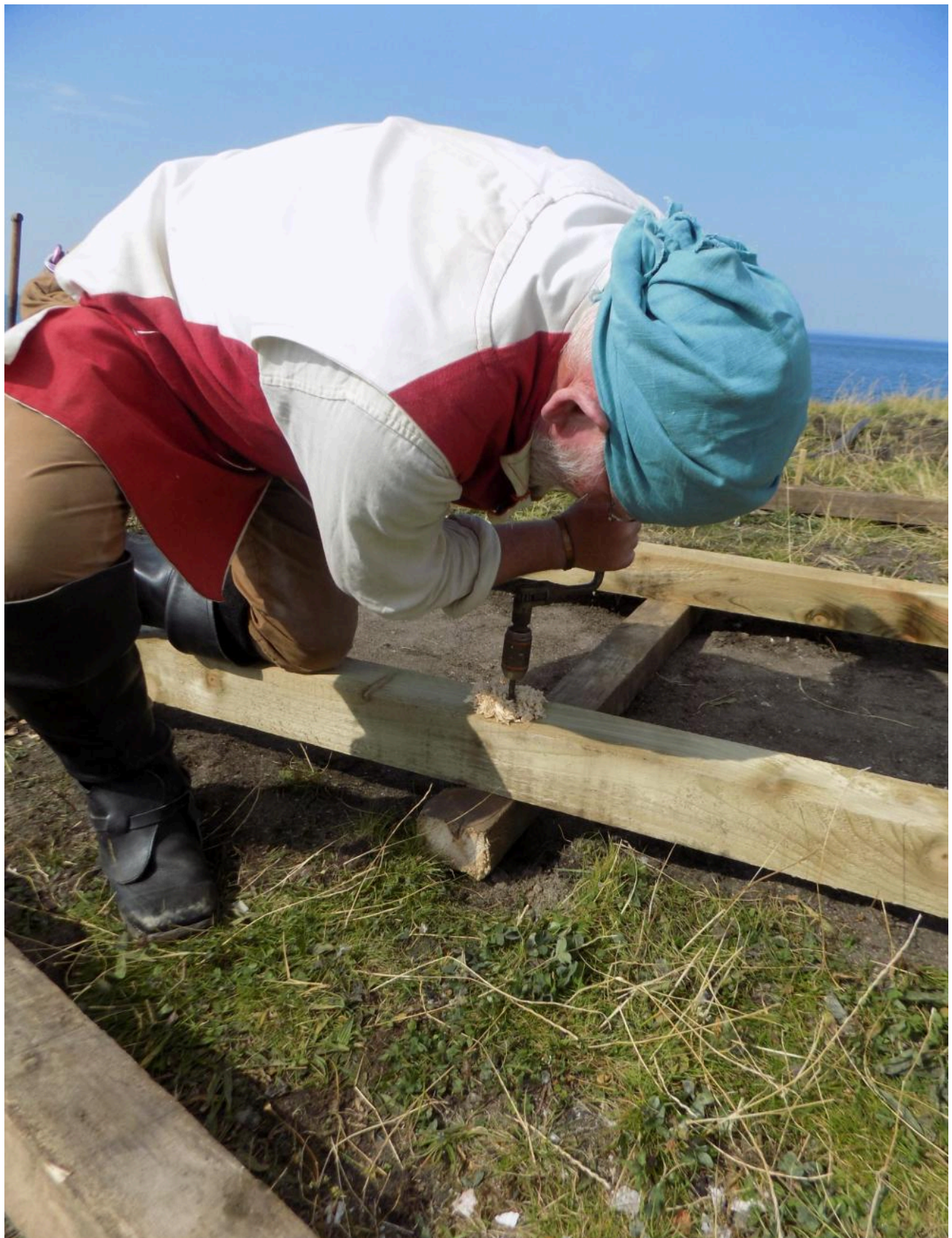
FIG 15. DRILLING HOLES FOR TRENAILS BY HAND THROUGH THE RAIL AND THE FULL THICKNESS OF THE SLEEPER. THIS PROCESS TOOK APPROXIMATELY 1MINUTE USING A CARPENTER'S BRACE. PHOTO BY ANTHONY DAWSON.
