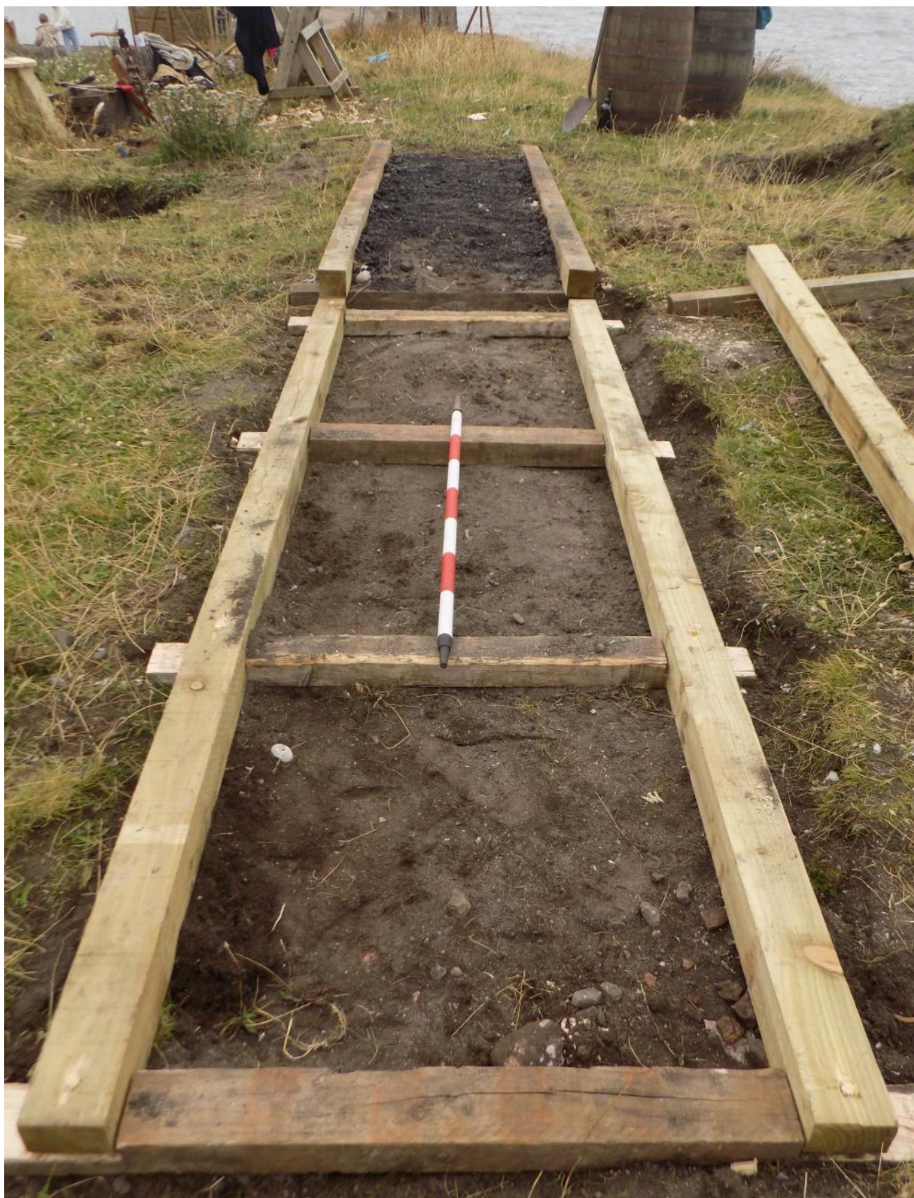
FIG 22. THE LOWER SET OF RAILS SECURED IN POSITION WITH TRENAILS. THE MORE ROBUST CONSTRUCTION COMPARED TO THE SINGLE-PHASE WHERE RAILS WERE SIMPLY MATED ONTO ROUGHLY PREPARED SLEEPERS IS EVIDENT. AGAIN, HOWEVER, THE SKILL REQUIRED TO PRODUCE SUCH A WAGGONWAY WAS RELATIVELY LOW. PHOTO BY ANTHONY DAWSON.
