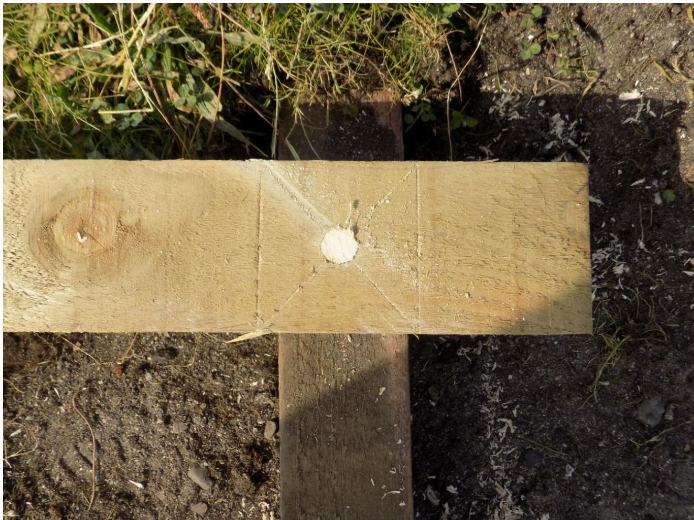
FIG 16. TRENNAILS WERE TRIMMED USING A SAW (HERE) AND ADZE. THE SAW LEFT THE NEATEST RESULT AND CREATED THE LEAST AMOUNT OF WASTE. IT ALSO LEFT A TELL-TALE SAW MARK AS A RESULT OF THE SAWING PROCESS. PHOTO BY ANTHONY DAWSON.
