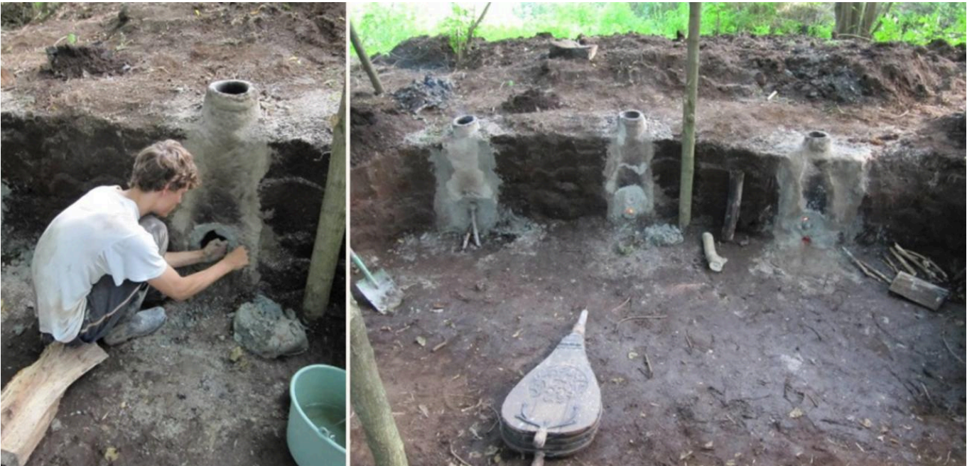
FIG 4. BUILDING FURNACES.
