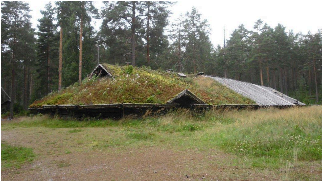
Fig. 2. The longhouse from SE. The reconstruction is 40 m long, 9 m wide, have birch-bark roof and walls of braided twigs sealed with clay. The building is supported by heavy poles. Photo Carl L. Thunberg (2012-08-21).
