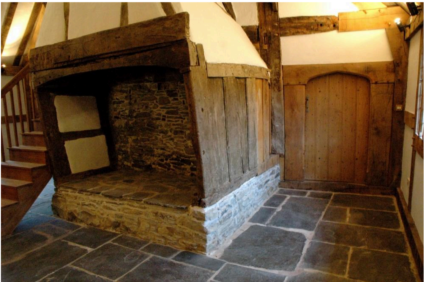
FIG 3. TIMBER SMOKE HOOD CIRCA 1635.
