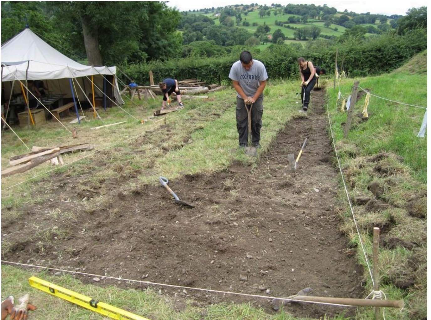
FIG 6. INTERNATIONAL VOLUNTEERS DIGGING A TERRACE FOR TIMBER FRAMED BUILDING RECONSTRUCTION AT TY MAWR MEDIEVAL HALL.
