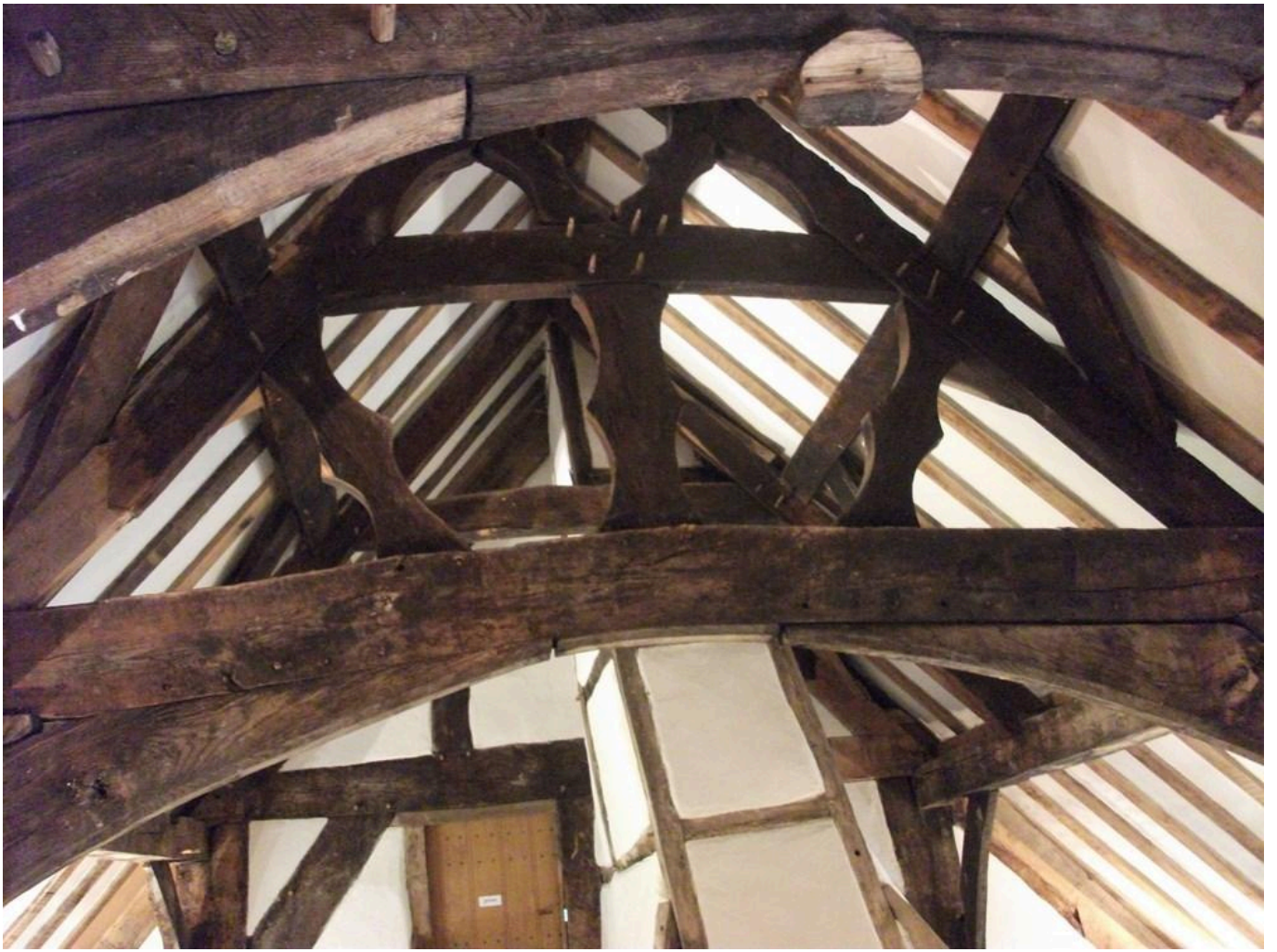
FIG 2. CENTRAL CRUCK TRUSS CIRCA 1460.
