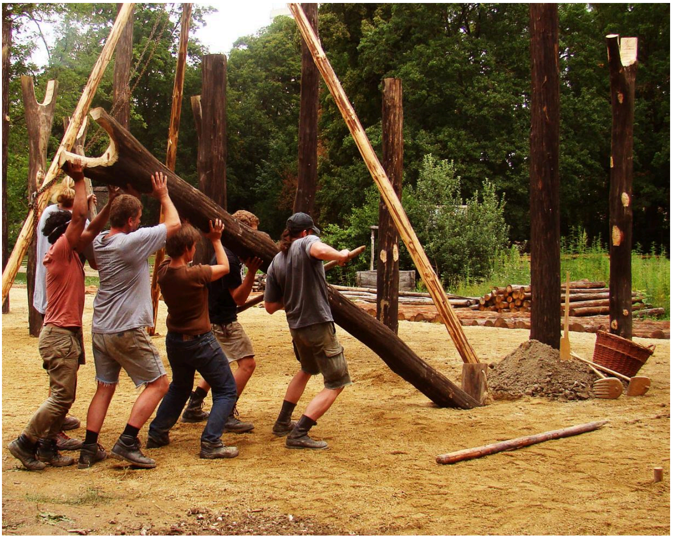
FIG 8. A FORKED POST IS PLACED IN A POST HOLE AND SET UPRIGHT; A VERTICAL PLANK IN THE HOLE PREVENTS THE TIMBER PULLING SOIL FROM THE PIT WALL DOWN WITH IT.
