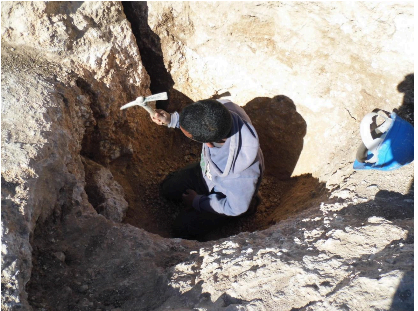
FIG 6. CAREFUL CHISELLING WITH A SMALL PICK-AXE GIVES A ROUNDED SHAPE TO THE SHAFT (COURTESY OF THE IAA)
