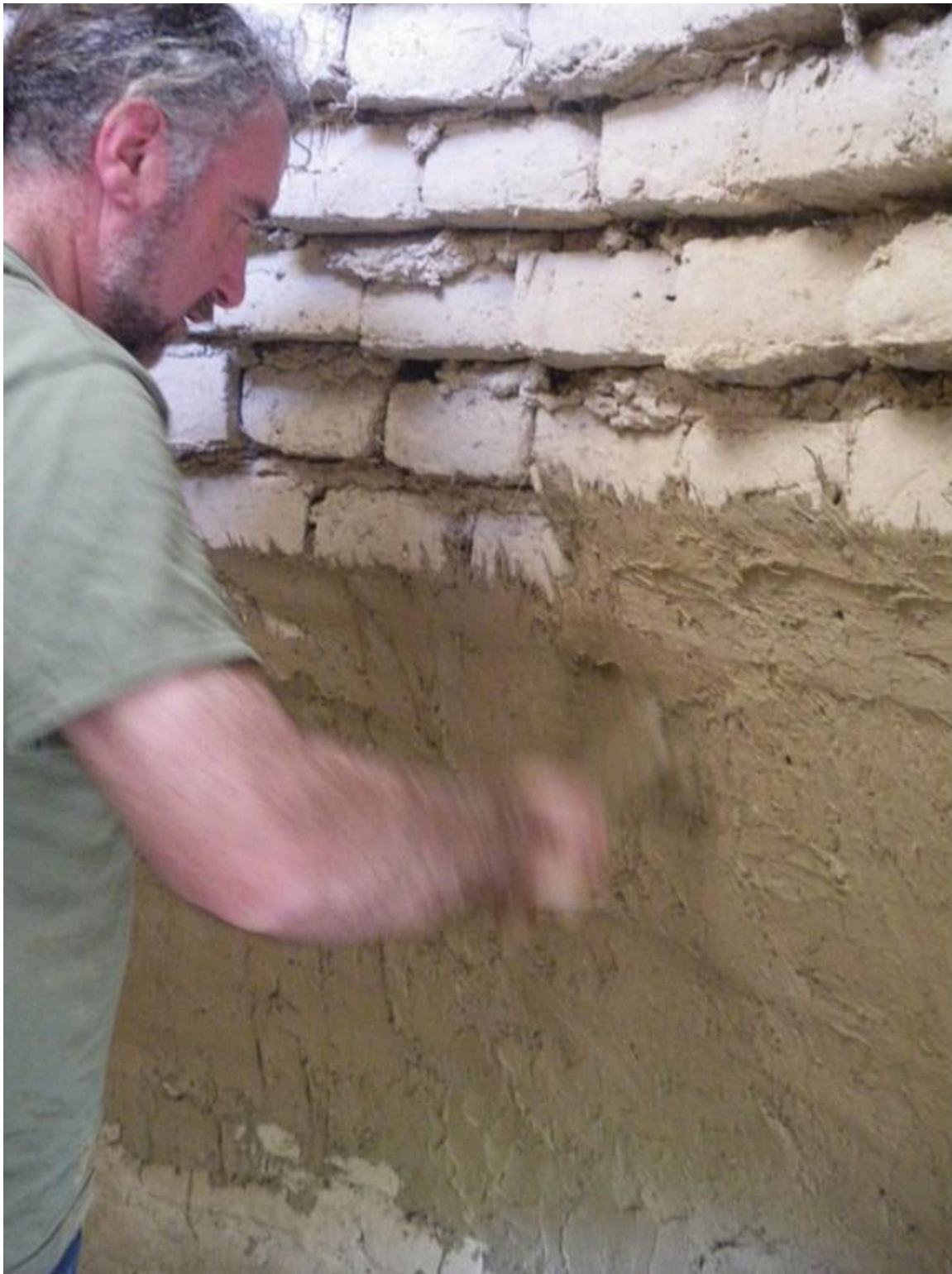
FIG 15. PLASTERING OF THE INTERIOR OF THE FIRING CHAMBER OF THE EXPERIMENTAL KILN OF VERDÚ.
