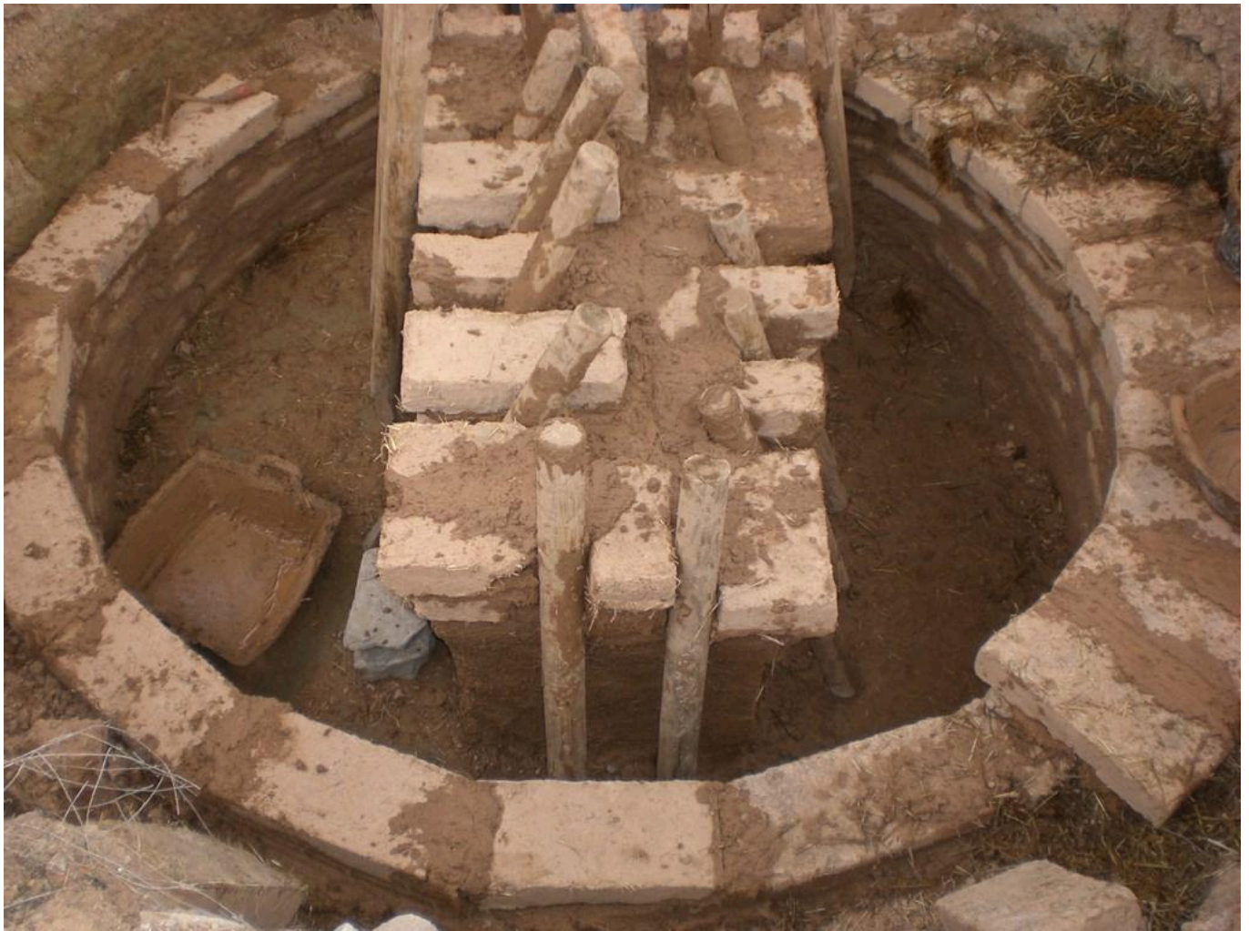
FIG 9. VIEW OF THE CENTRAL PILLAR AND THE BOUGHS PLACED TO SUPPORT THE GRATE DURING CONSTRUCTION OF THE EXPERIMENTAL KILN OF VERDÚ.
