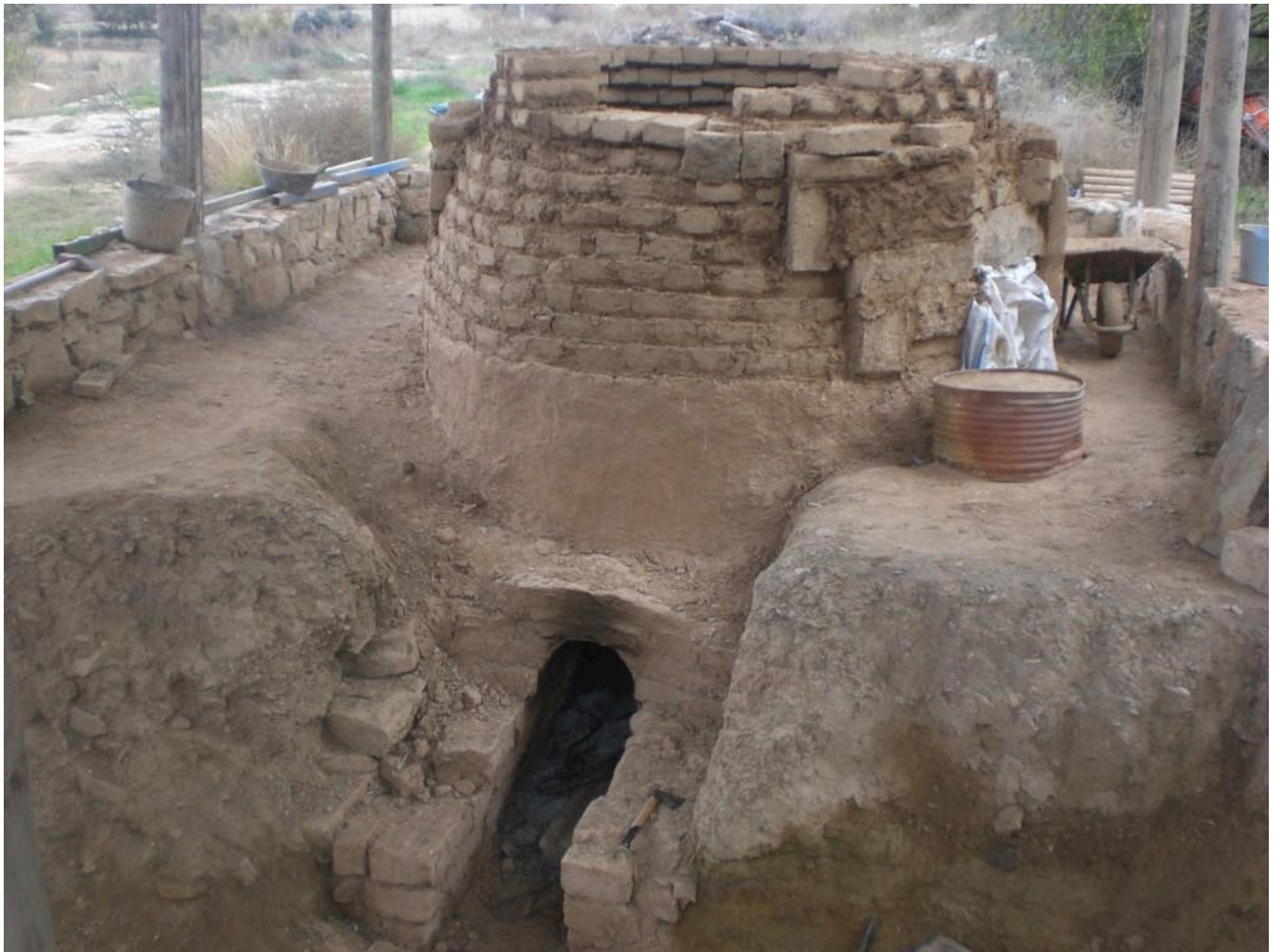
FIG 14. VIEW OF THE BRICK-BUILT FIRING CHAMBER OF THE EXPERIMENTAL KILN OF VERDÚ.
