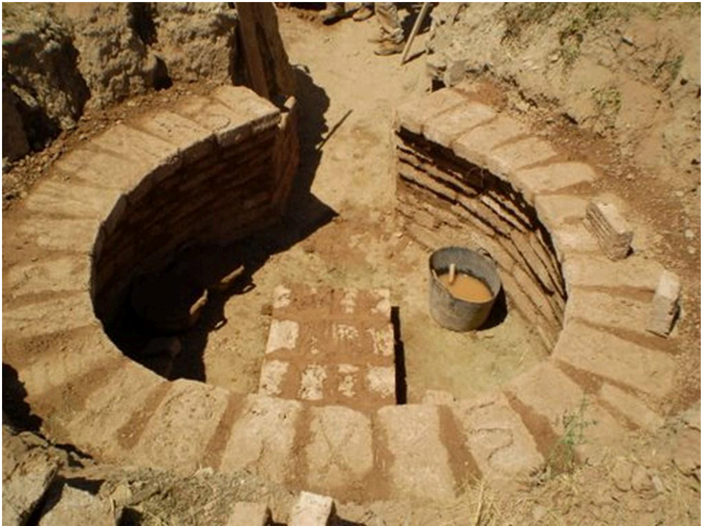
FIG 8. CONSTRUCTION OF THE COMBUSTION CHAMBER AND THE CENTRAL PILLAR OF THE EXPERIMENTAL KILN OF VERDÚ.
