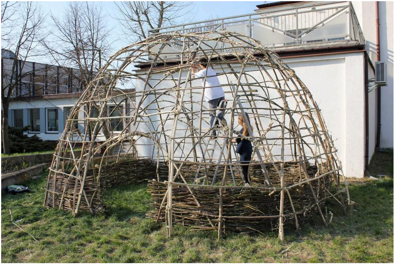
FIG 2C. CONSTRUCTION OF THE MESOLITHIC SHELTER - STAGES OF WORK.
