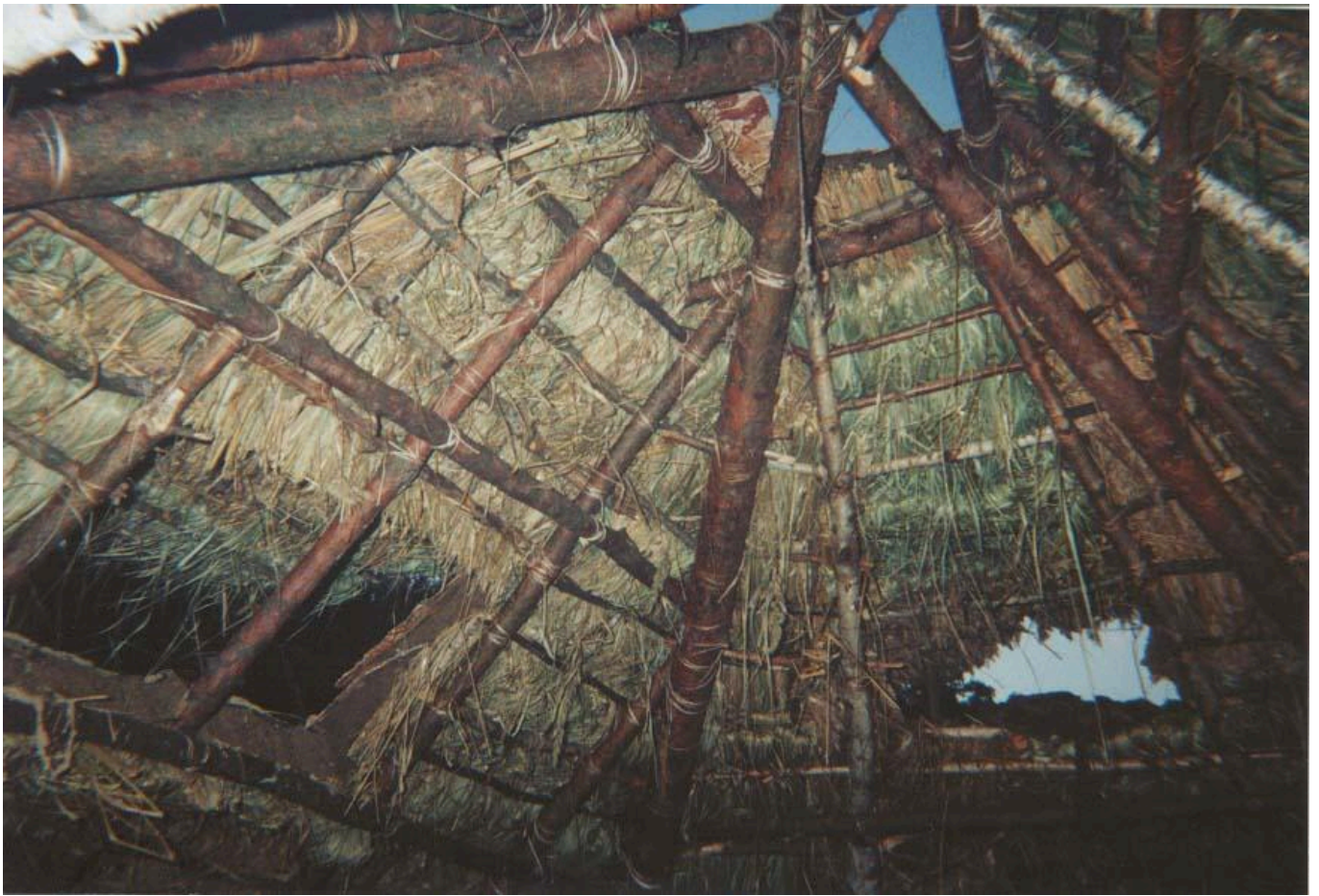
FIG 1G. CONSTRUCTION OF THE STONE AGES SHALLOW PIT-HOUSE – STAGES OF WORK.
