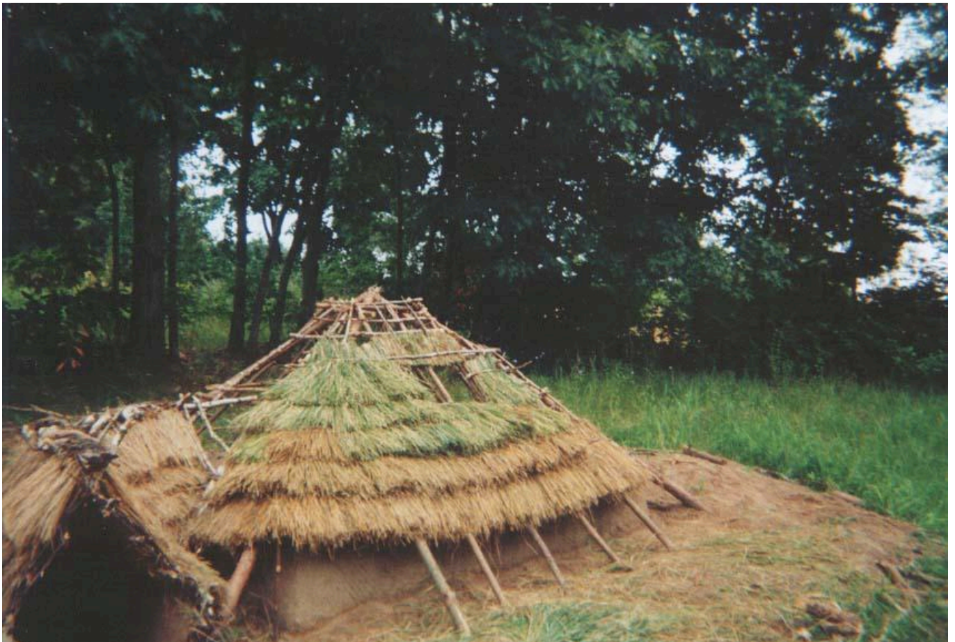
FIG 1F. CONSTRUCTION OF THE STONE AGES SHALLOW PIT-HOUSE – STAGES OF WORK.
