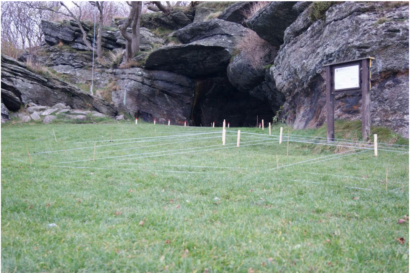
FIG 3. HERE WE SEE THE CREW USING WIRES ON TWO DIFFERENT LEVELS TO CHECK HOW THE PATH CAN BE ELEVATED WITHOUT INTERRUPTING THE MAIN LANDSCAPE LINES. A HIGHER BUILD-UP RESULTS IN A LESS STEEP INCLINE AND BETTER DESIGN SOLUTION, BUT ALSO INCREASED LANDSCAPE INTERVENTION.
