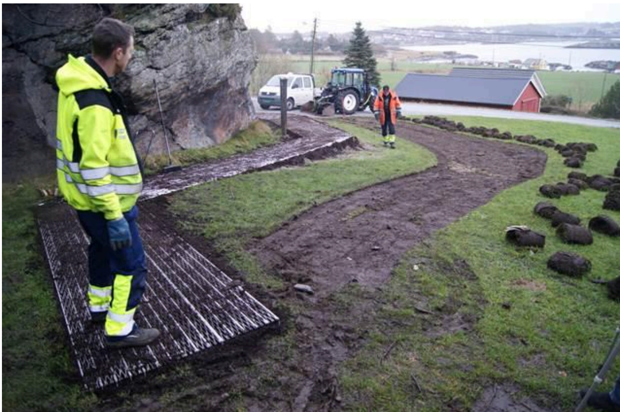
FIG 7. THE GRASS IS PEELED BACK BEFORE FILLING OVER WITH SAND AND SOIL TO ADAPT THE RAISED PATH TO THE LANDSCAPE. THE PEELED-OFF AREA SHOWS THE EXTENT OF LANDSCAPING REQUIRED TO ADAPT THE 120 CM WIDE PATH TO THE LANDSCAPE.
