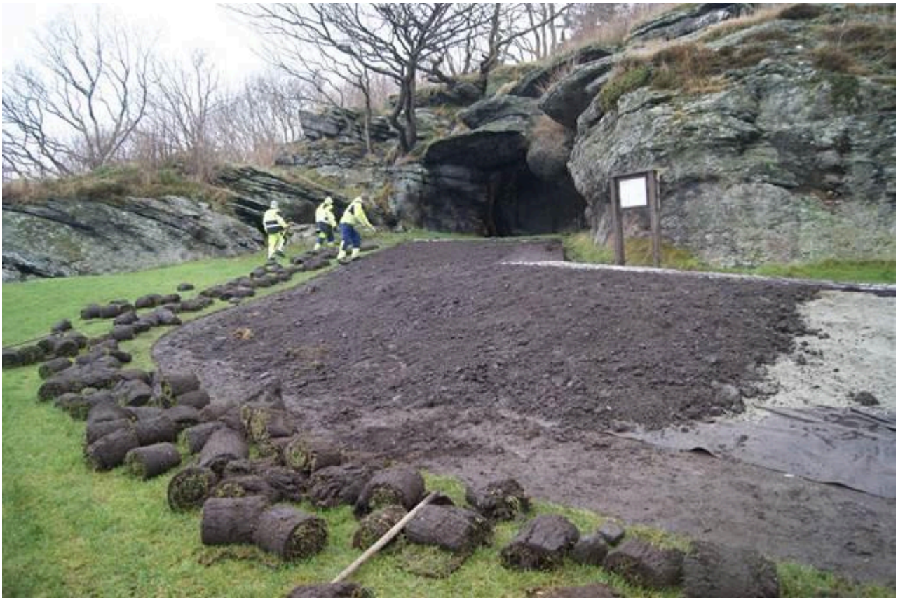
FIG 8. THE LANDSCAPING MEASURES ARE WELL UNDERWAY. NOTE THE FABRIC ON THE GROUND. ALSO NOTE THAT A GOOD DEAL OF SAND IS NEEDED AT THE FAR END OF THE LANDSCAPED AREA TO KEEP THE PATH IN PLACE.
