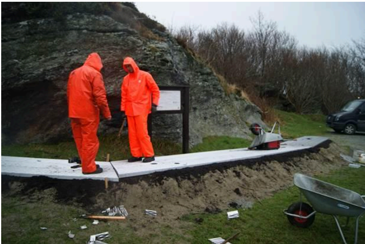
FIG 6. THE GRATES BEING INSTALLED. NOTE THE SOIL LAYER ON TOP OF THE GRAVEL. THIS PROVIDES THE GRASS WITH SOMEWHERE TO TAKE HOLD. NOTE ALSO HOW MUCH THE PATH IS RAISED.
