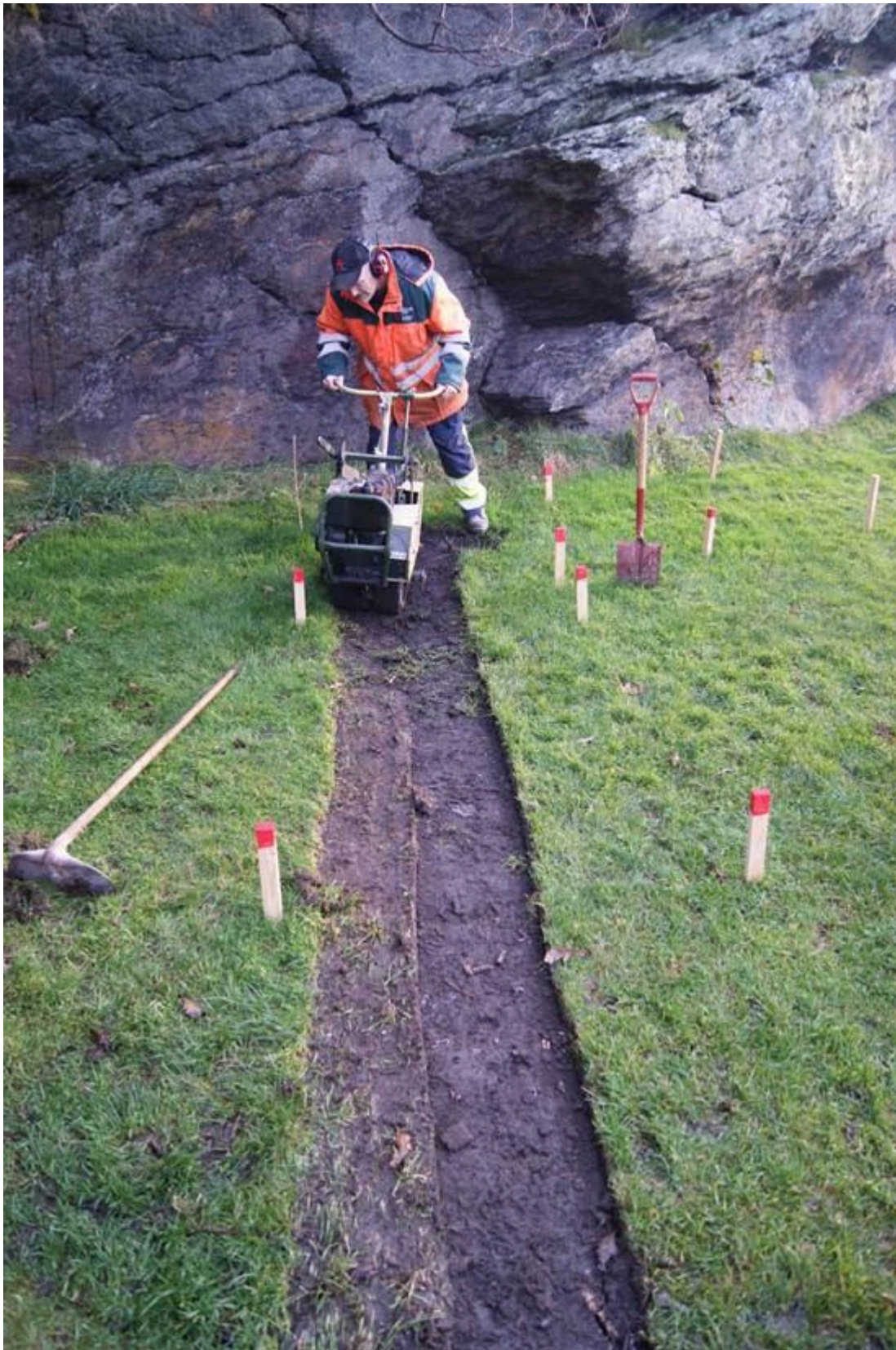
FIG 5. PEELING BACK 5–7 CM OF TURF DIRECTLY IN FRONT OF THE CAVE TO INSTALL THE GRATING AT THE CURRENT GROUND LEVEL. THE ENTIRE PROCESS WAS MONITORED BY ARCHAEOLOGISTS; NO DISCOVERIES WERE MADE.
