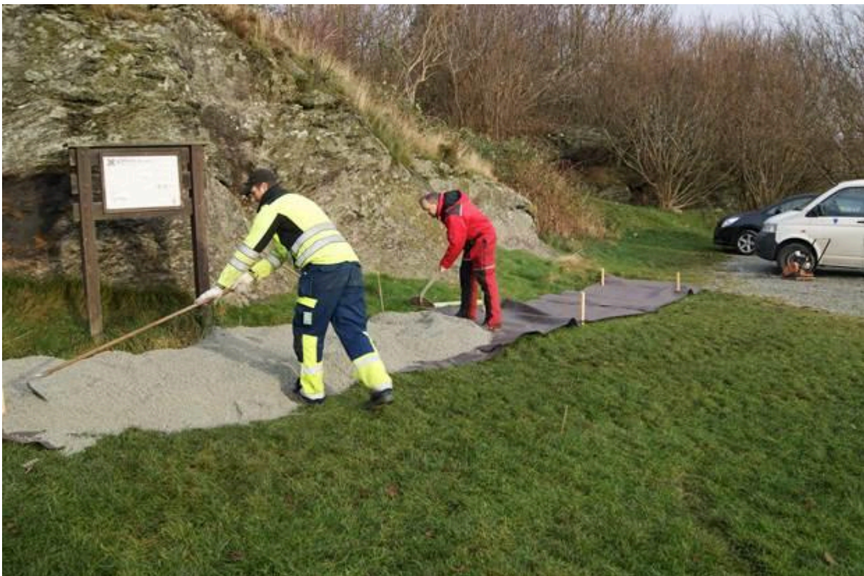
FIG 4. PHYSICAL EXECUTION. FILLING IN GRAVEL TO PROVIDE A SOUND FOUNDATION FOR THE GRATING. EVERYTHING IS REVERSIBLE TO AVOID DAMAGING THE ORIGINAL SURFACE.
