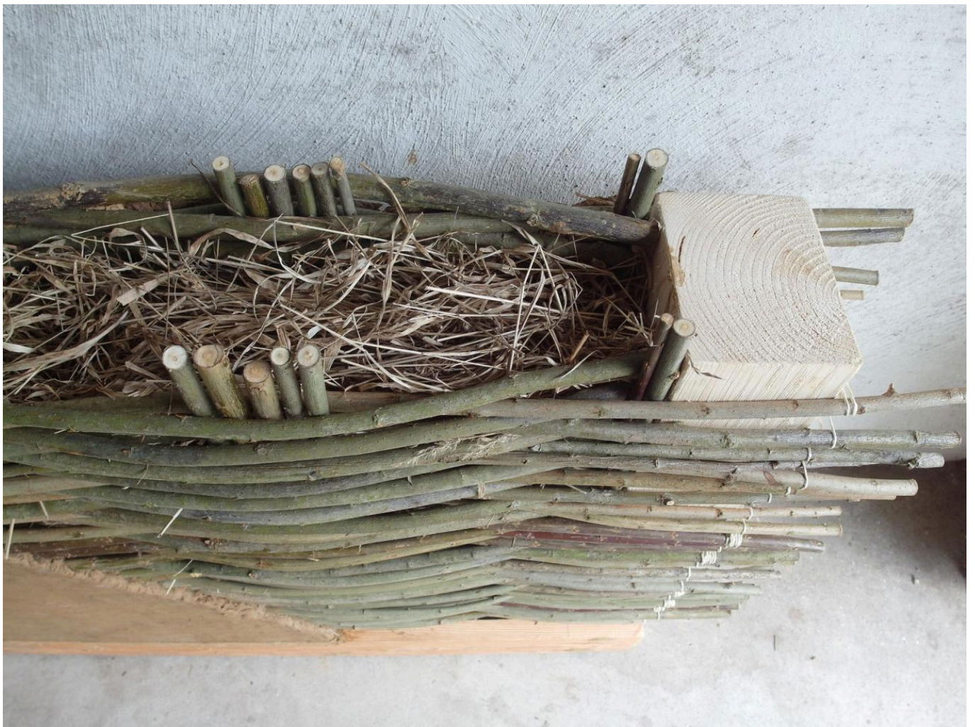
FIG 2. VIEW FROM ABOVE ONTO THE WALL WITH BEAM, TWO WATTLES AND GRASS FILLING.
