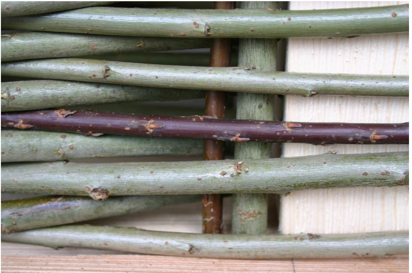
FIG 13. RECONSTRUCTION: RODS LED ALONG THE OUTSIDE OF A BEAM CONNECT THE WATTLE WITH THE SUPPORTING CONSTRUCTION.
