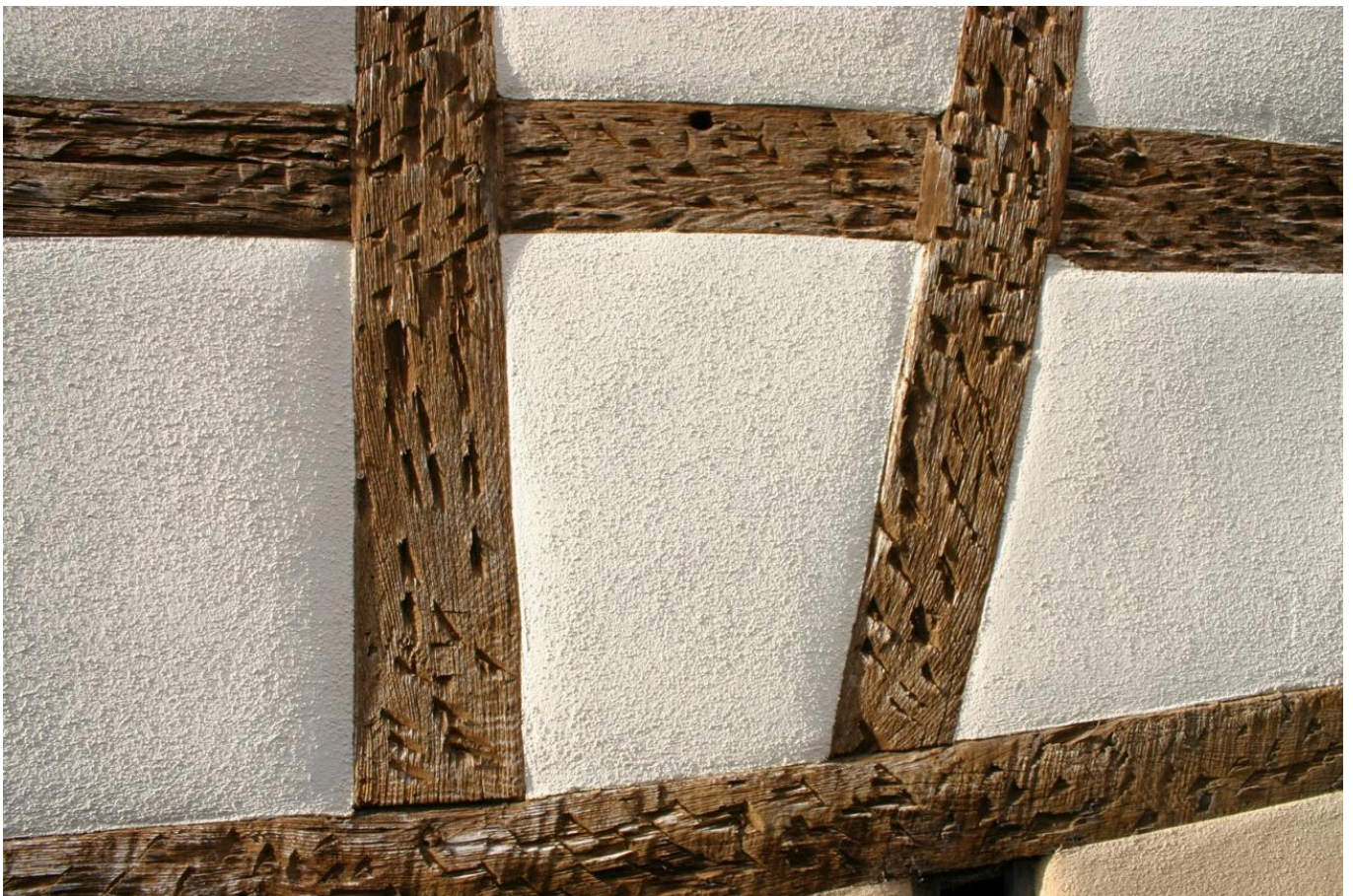
FIG 16. BLOWS/CUTS FROM AN AXE ROUGHENED THE SURFACE OF THE BEAMS TO ENSURE THE PLASTER WOULD STAY ON THE WOOD. OLD TIMBER FRAMED HOUSE IN GELNHAUSEN (HESSIA).
