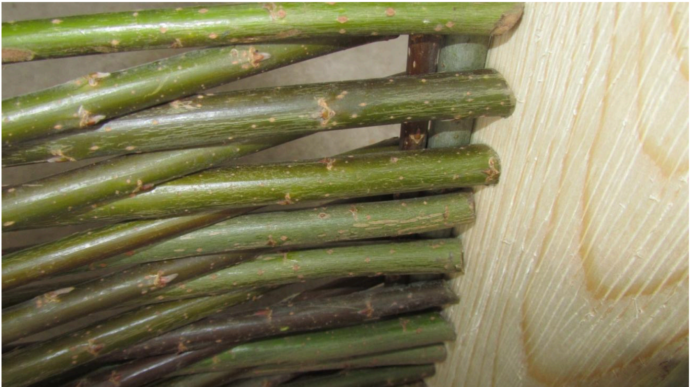
FIG 14. RECONSTRUCTION: RODS THAT STAY INSIDE ARE CLAMPED BEHIND THE POLES NEXT TO THE BEAM.
