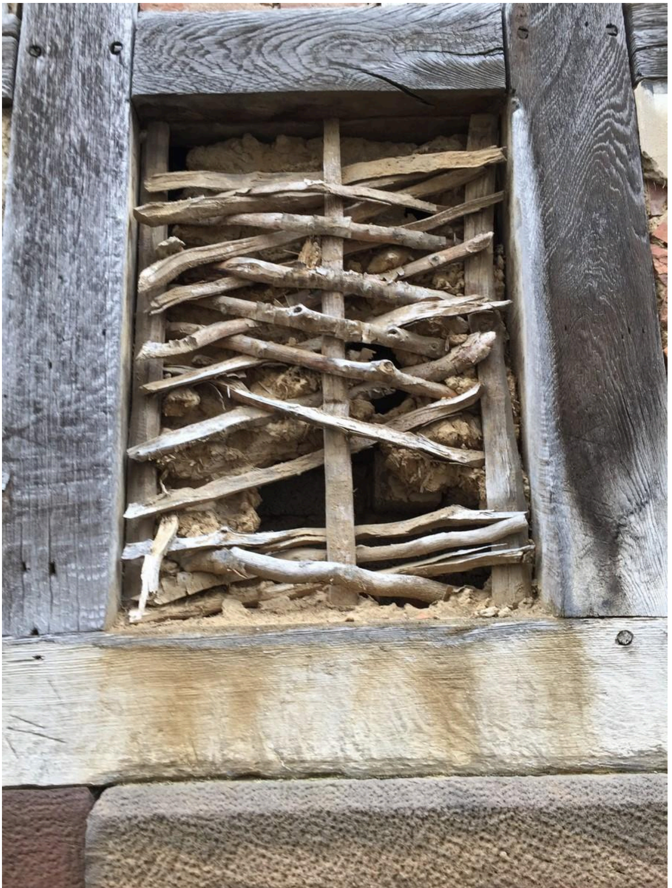
FIG 12. WATTLE OF A BARN IN RAUISCHHOLZHAUSEN (HESSIA). TWO POLES ARE SIDE BY SIDE NEXT TO THE VERTICAL BEAMS. BOTH POLE ENDS ARE CLAMPED IN A GROOVE IN THE UPPER AND LOWER BEAM. THE RODS ARE CLAMPED BEFORE AND BEHIND THESE POLES.
