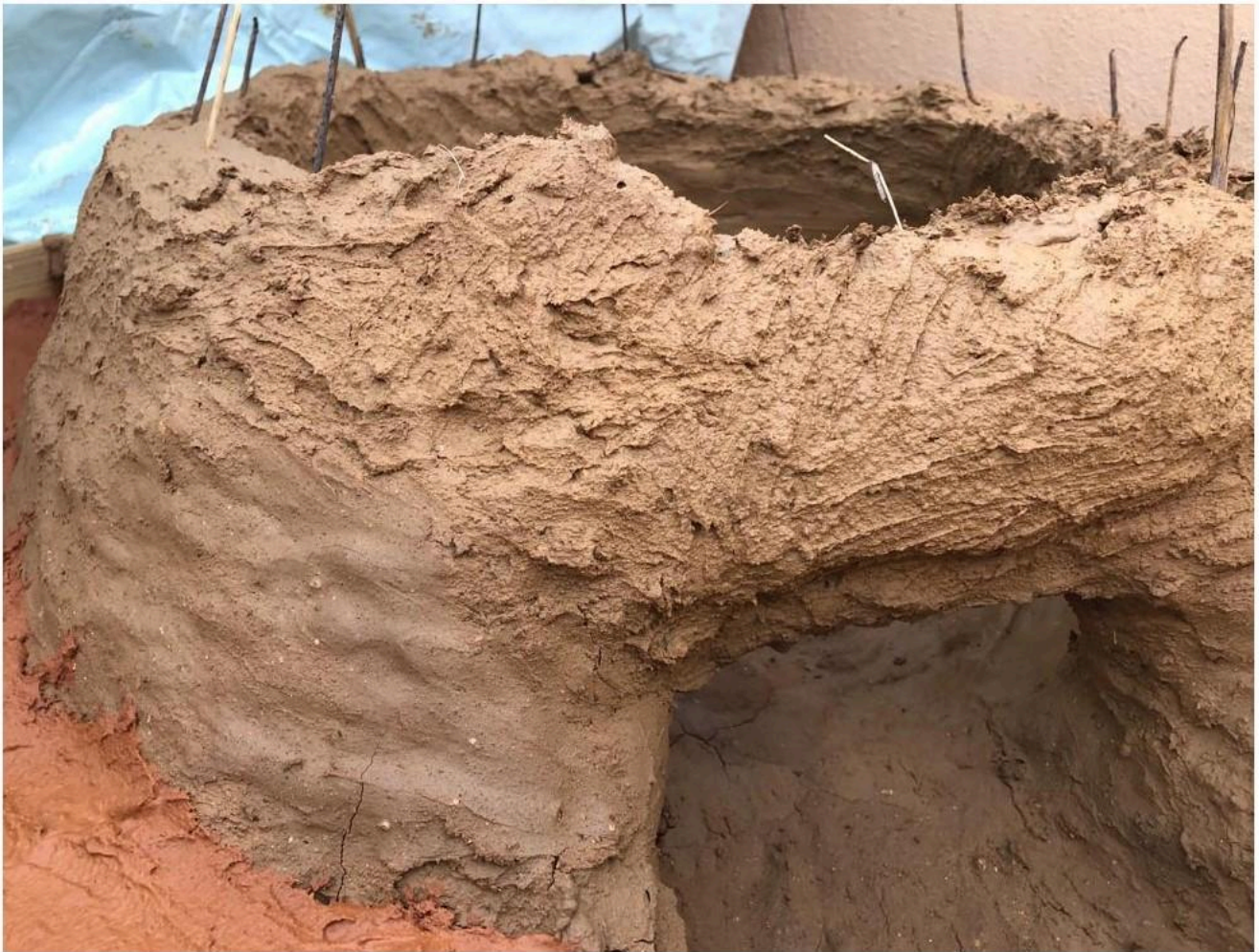
FIG 4. PROCESS OF ELABORATION OF THE FIXED TANNŪR. PHOTO BY CARMEN RAMÍREZ CAÑAS ET AL
