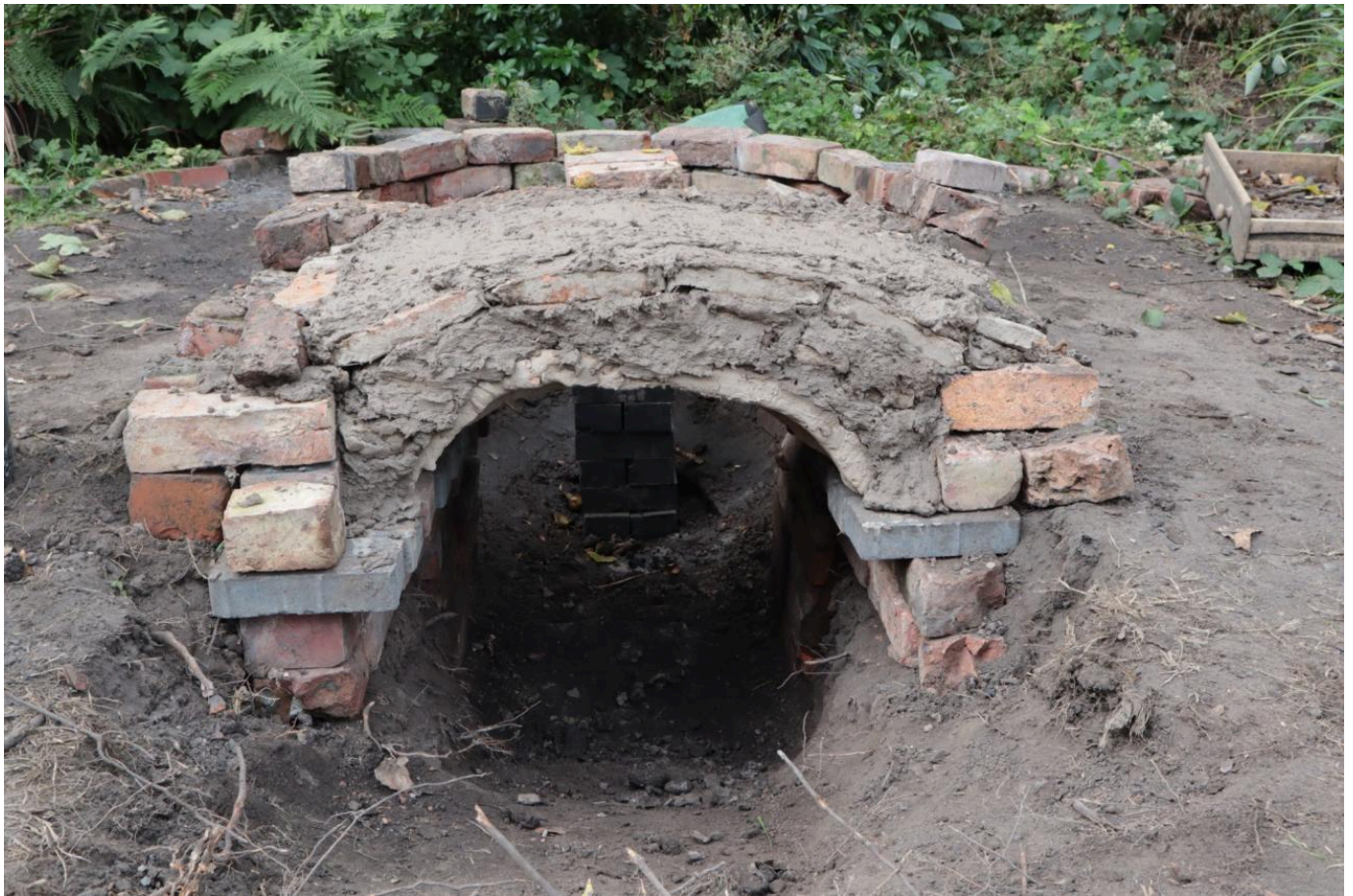
FIG 18. THE STOKING CHANNEL COMPLETED WITH TWO LAYERS OF ADOBE BRICKS AND CLAY CEMENT (TOMEI AND JIMÉNEZ RIVERO)
