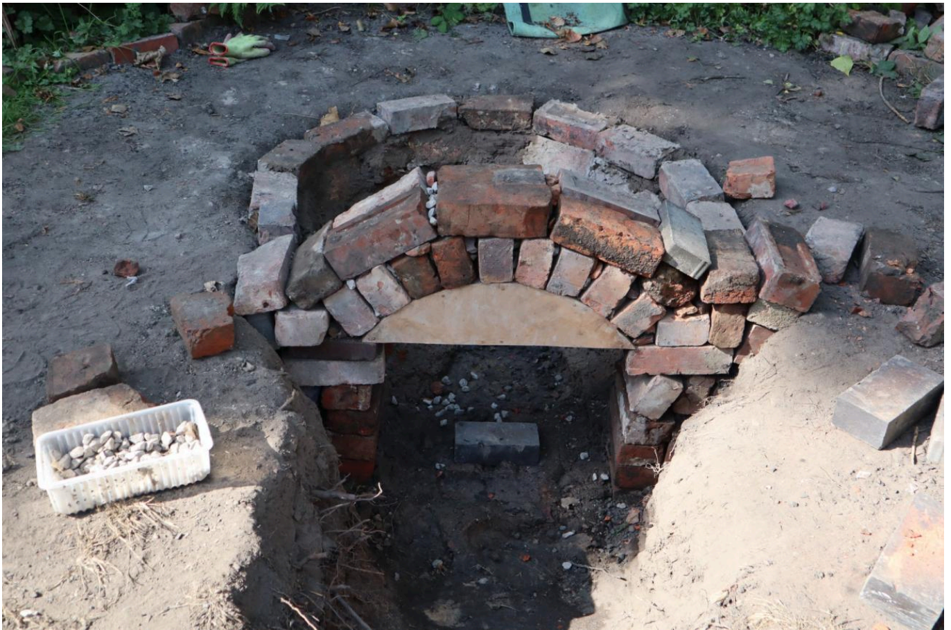
FIG 12. BUILDING THE ARCH WITH A WOODEN ARCH-SHAPED FRAME (TOMEI AND JIMÉNEZ RIVERO)
