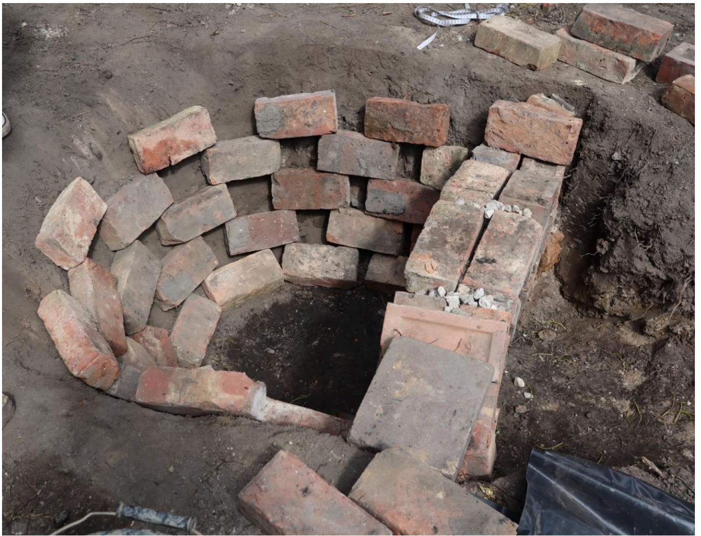
FIG 14. THE WALLS OF THE COMBUSTION CHAMBER REINFORCED WITH A FRAME OF VICTORIAN BRICKS (TOMEI AND JIMÉNEZ RIVERO)
