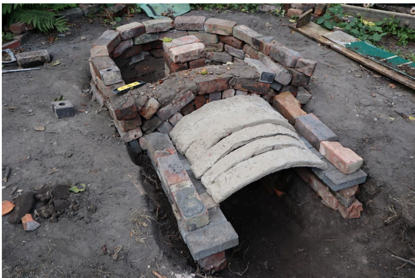
FIG 17. MAKING THE STOKING CHANNEL WITH CLAY COILS (TOMEI AND JIMÉNEZ RIVERO)
