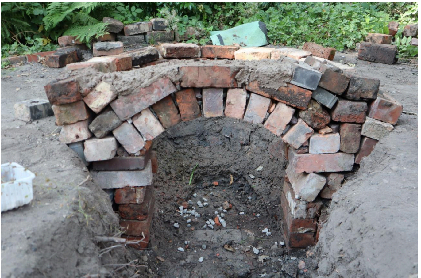
FIG 13. THE ARCH STANDS ON ITS OWN WEIGHT AT THE ENTRANCE OF THE COMBUSTION CHAMBER (TOMEI AND JIMÉNEZ RIVERO)
