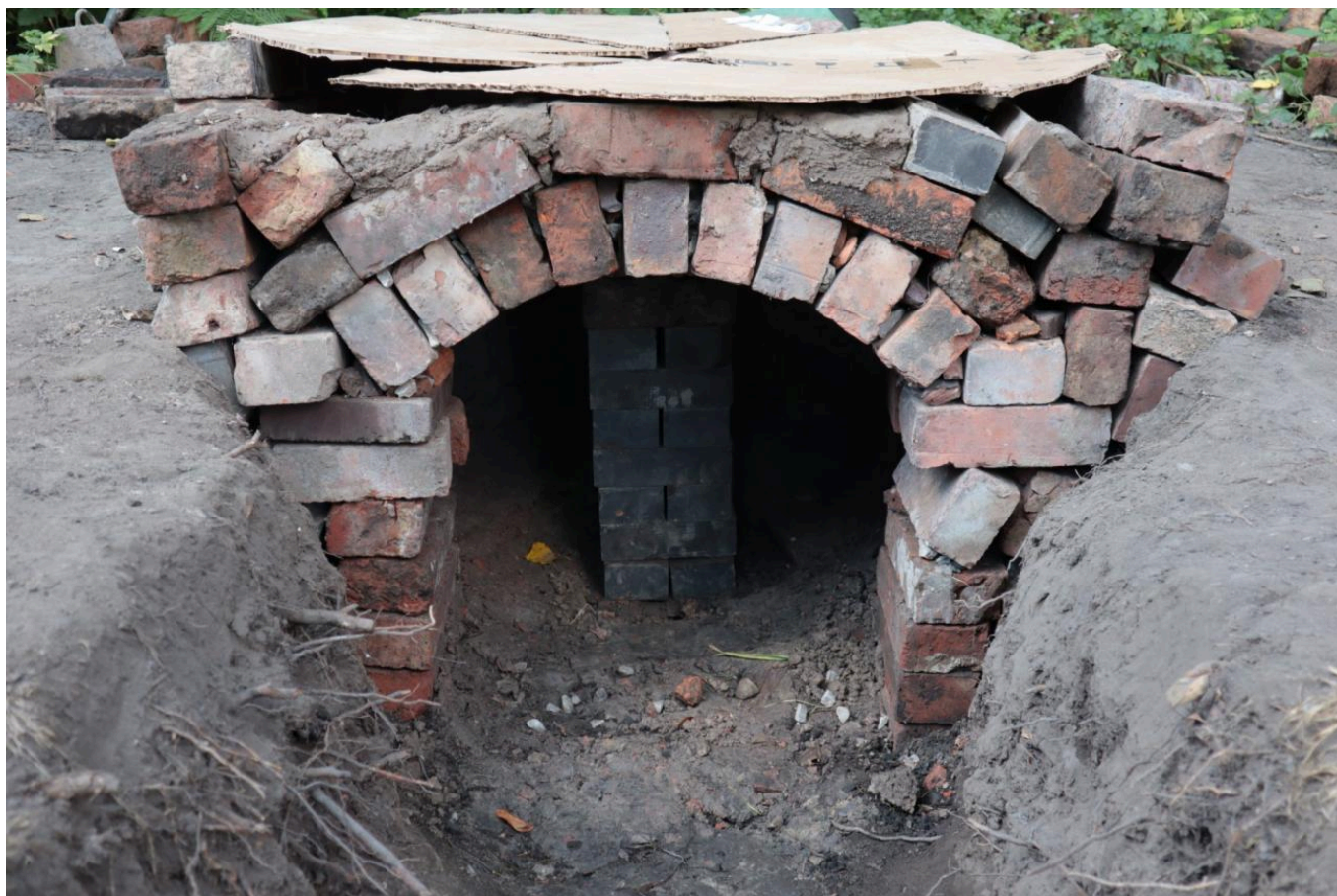
FIG 16. FINDING THE RIGHT POSITION OF THE CENTRAL PILLAR USING CARDBOARD PIECES TRACING THE PERFORATED FLOOR'S PORTIONS (TOMEI AND JIMÉNEZ RIVERO)
