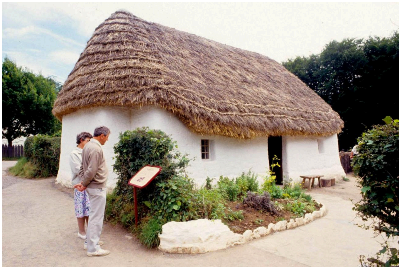
FIG 7. THE NANTWALLTER COTTAGE AT ST FAGANS. THIS BUILDING HAS BEEN OPEN ON THE SITE FOR OVER TWENTY YEARS AND REMAINS IN EXCELLENT CONDITION. THE CLOM WALLS ARE REGULARLY WHITEWASHED,
