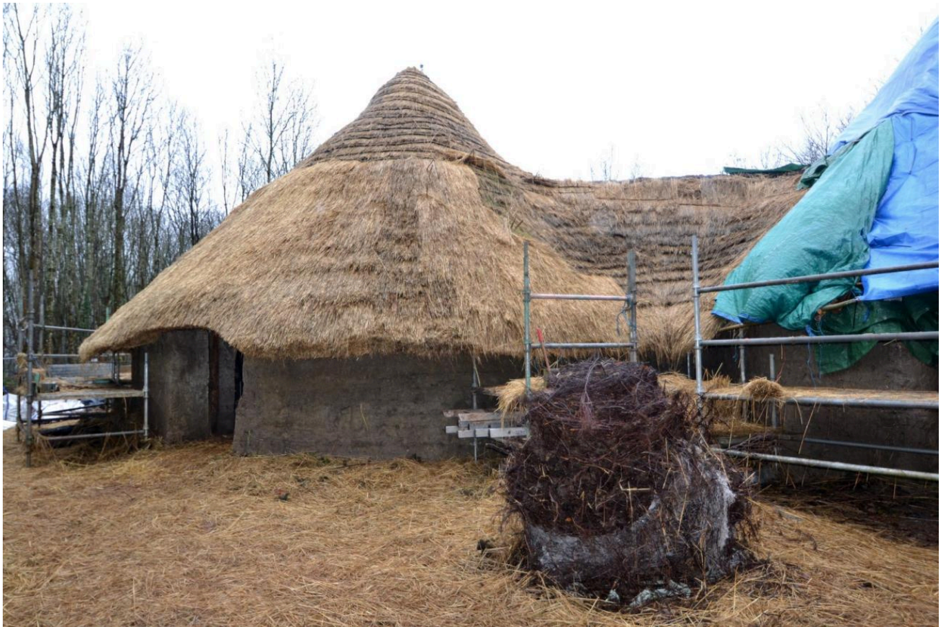
FIG 12. THE THATCHING OF THE ROOFS OF THE IRON AGE FARMSTEAD. THE SHAGGY APPEARANCE OF THE ROOFS IS A PRODUCT OF THE STUFF THATCHING TECHNIQUE USED THROUGHOUT.
