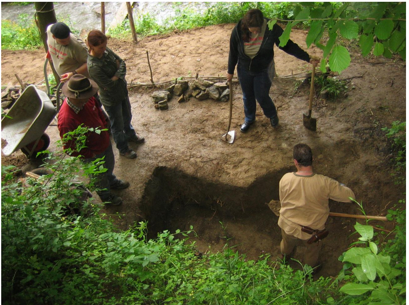
FIG 3. EXCAVATION OF A KEYHOLE-SHAPED FOUNDATION
