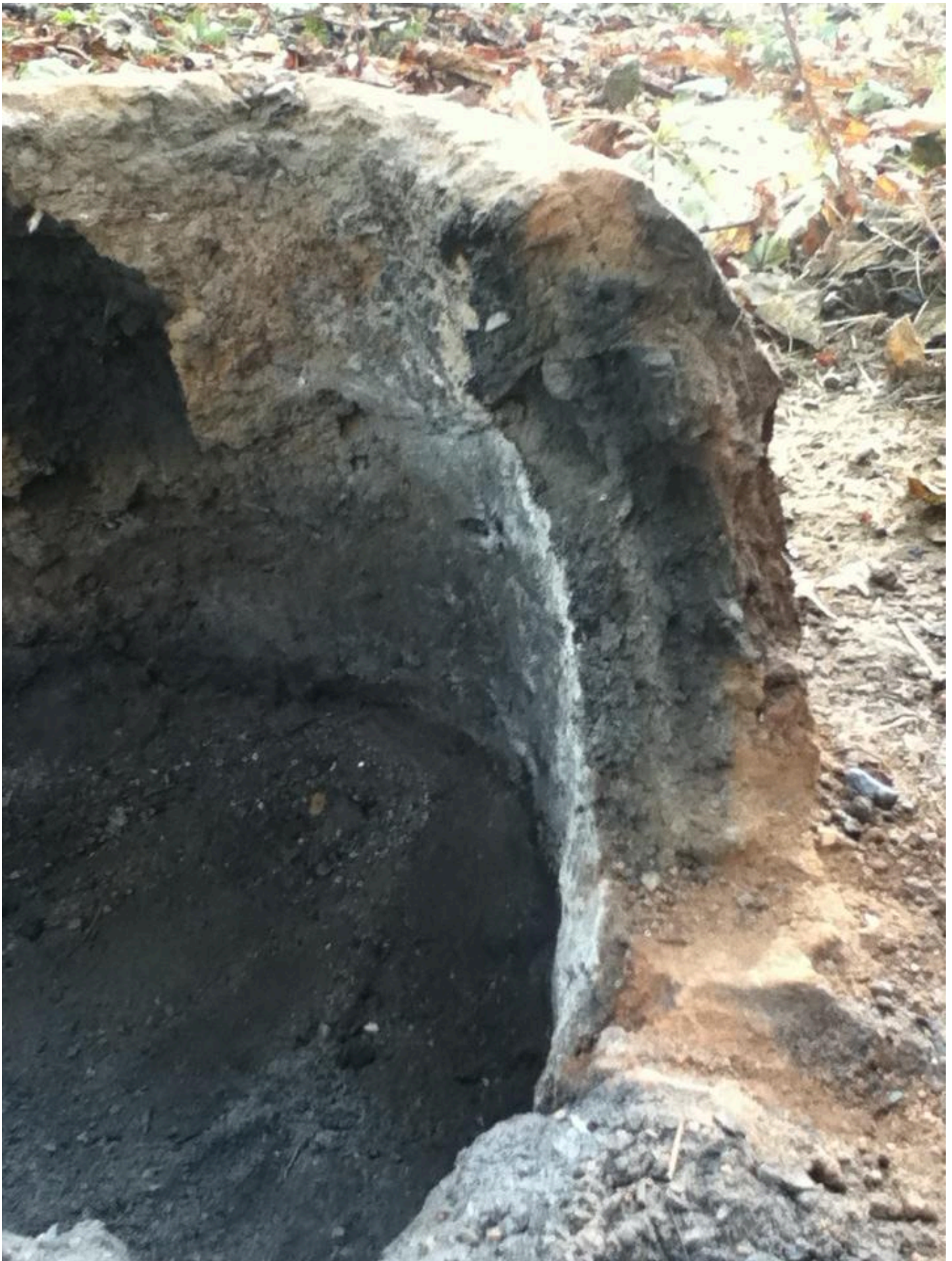
FIG 6. SECTION THROUGH FURNACE WALL, WHICH SHOWS THE REDUCING CORE EXTENDING TO TOP OF STRUCTURE. PHOTO BY Y. A. MARKS
