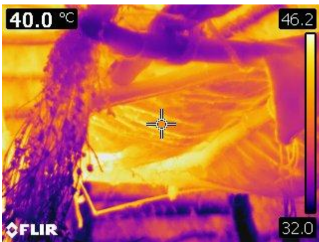
FIG 6A. THERMIC IMAGE IN THE HOUSE. PHOTO BY KAI-ERIK BALLAK
