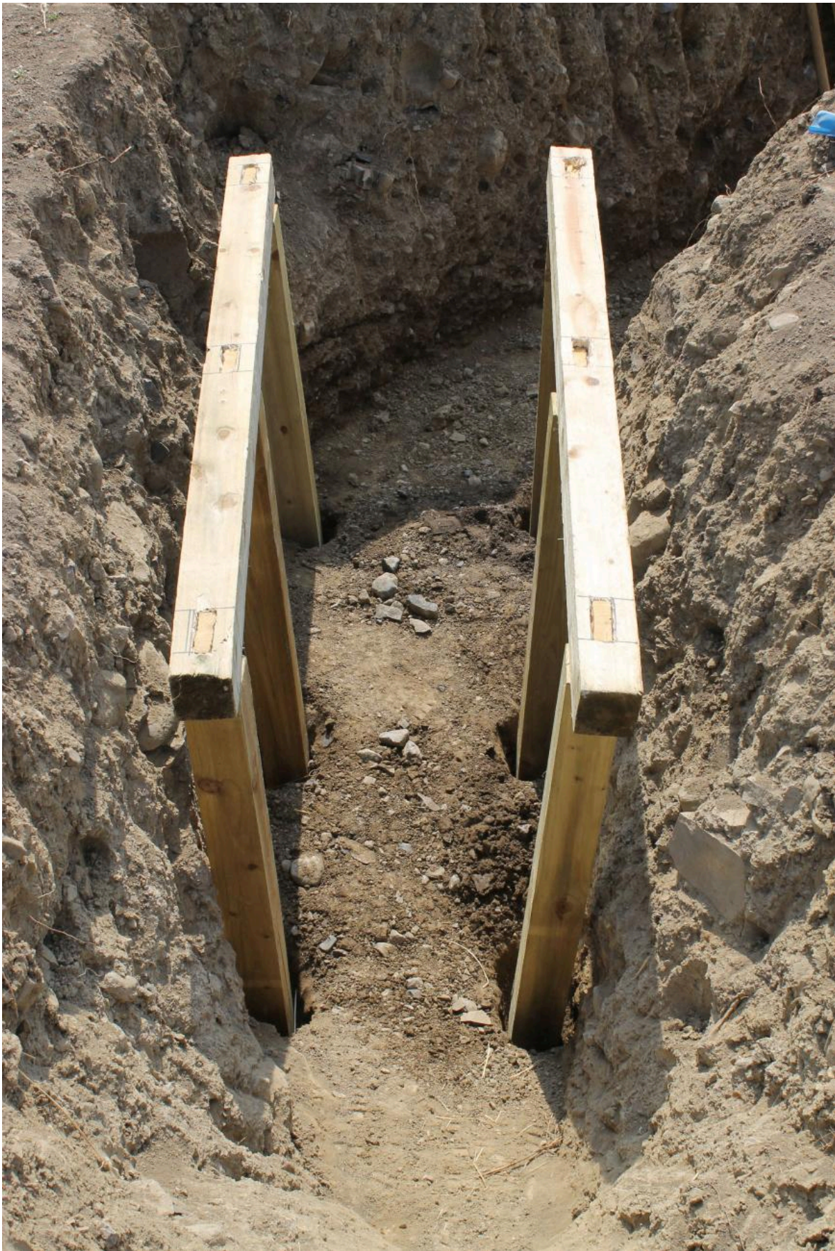
FIG 7. ADDING POSTS AND ROOFING BEAMS TO BUILD THE FRAME OF THE SOUTERRAIN. PHOTO BY TOM MEHARG
