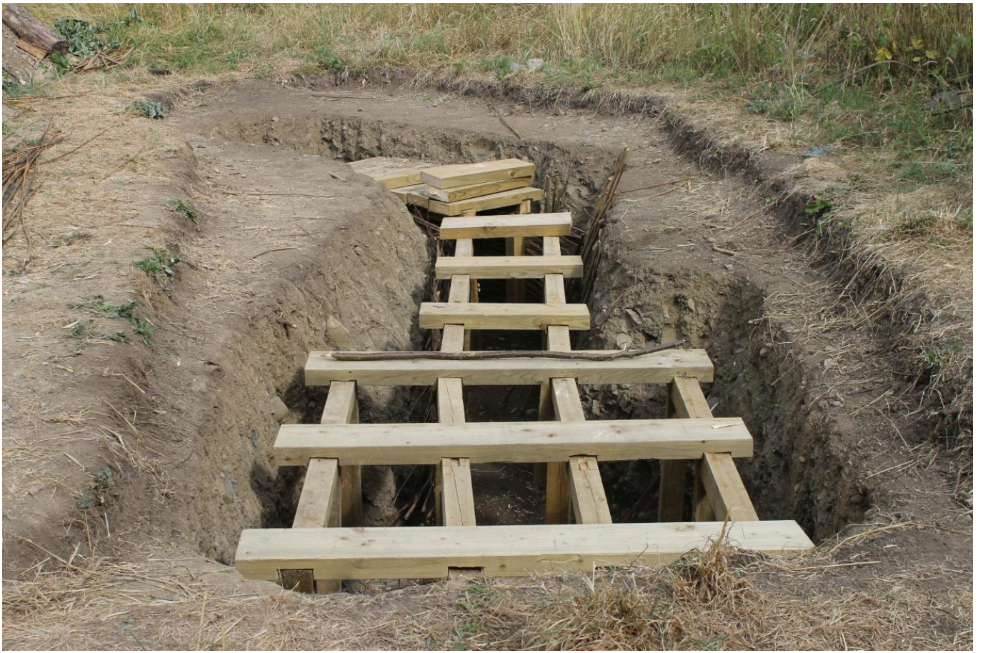
FIG 7. ADDING POSTS AND ROOFING BEAMS TO BUILD THE FRAME OF THE SOUTERRAIN. PHOTO BY TOM MEHARG
