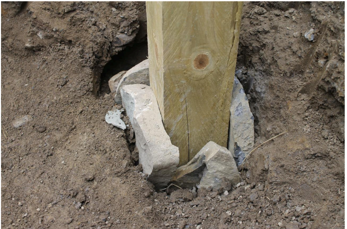
FIG 6. SECURING POSTS IN POSTHOLES WITH PACKING STONES. PHOTO BY TOM MEHARG
