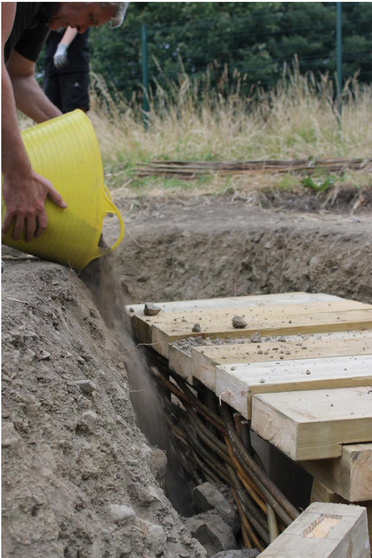
FIG 10. POURING THE LOOSE BOULDER CLAY INTO THE CAVITY BETWEEN THE WATTLE AND THE TRENCH WALL. PHOTO BY TOM MEHARG
