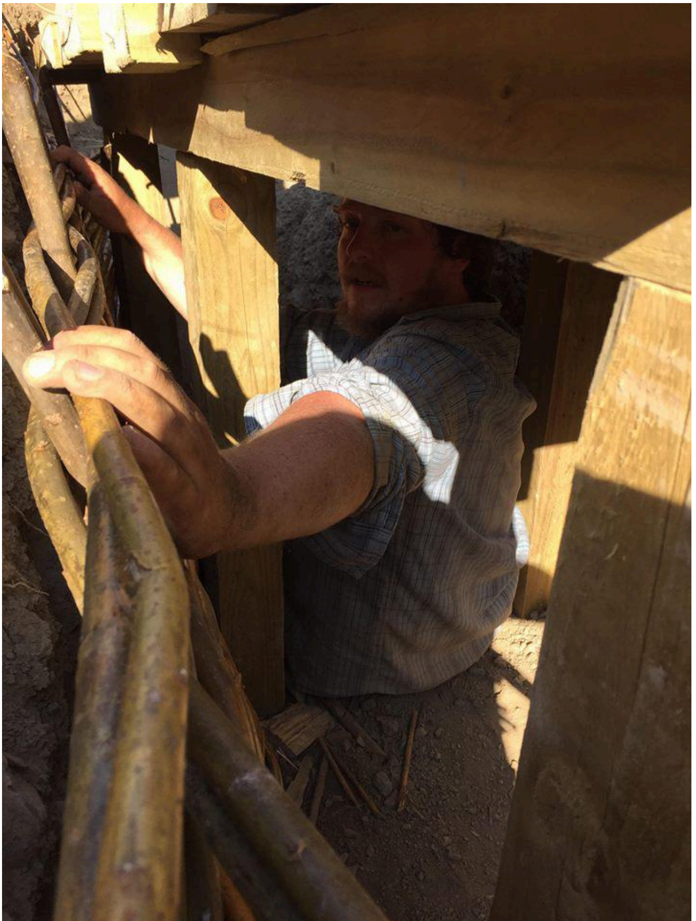
FIG 9. WEAVING THE WILLOW WATTLE RETAINING WALL BETWEEN THE FRAME AND THE TRENCH WALL. PHOTO BY TERRY RUNNER
