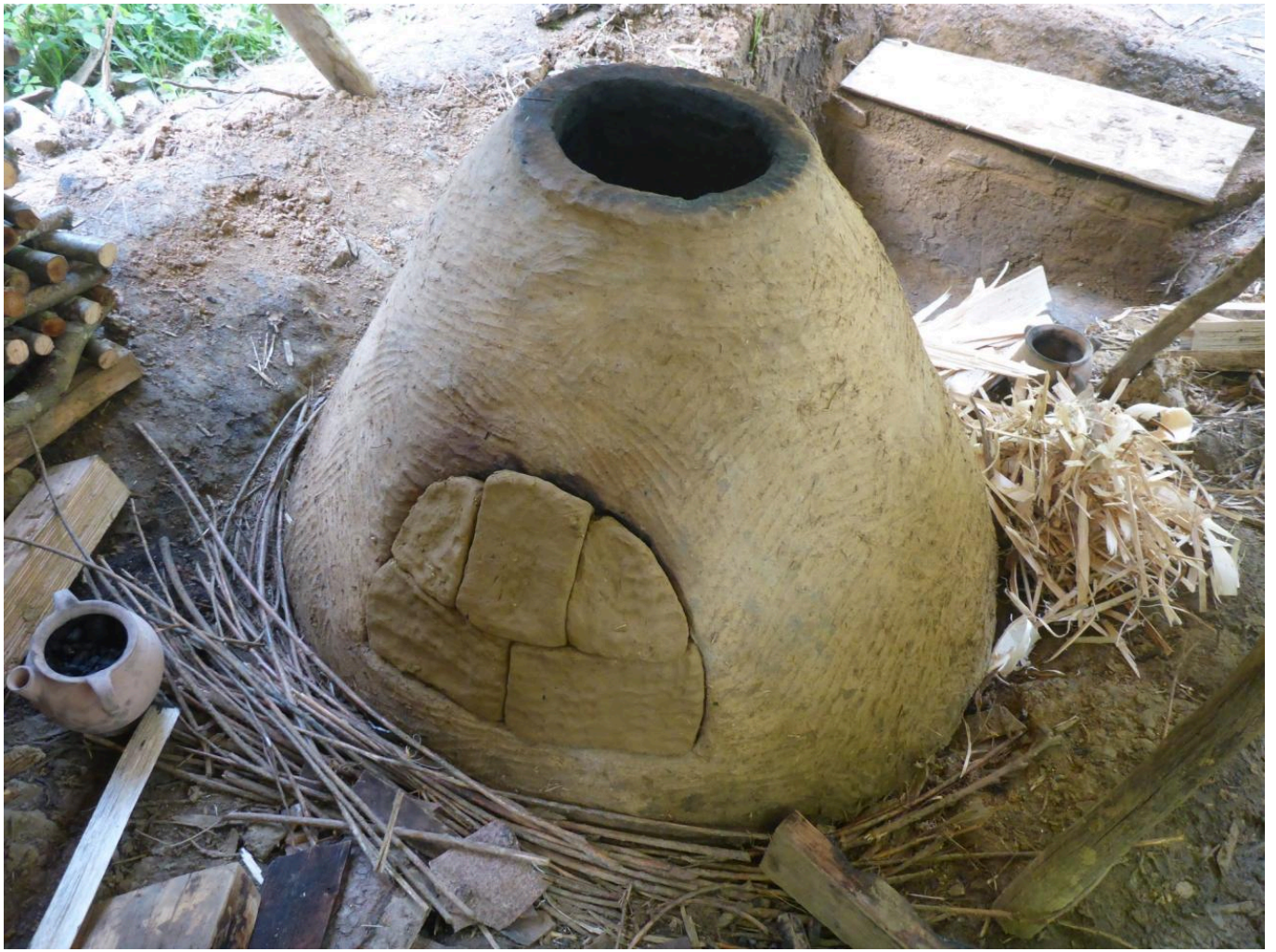
FIG 25. DOOR IN THE DOMED FIRING CHAMBER TO LOAD THE KILN WITH VESSELS, CLOSED WITH COB BRICKS.
