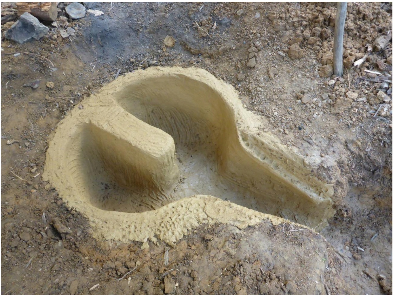
FIG 20. COMBUSTION CHAMBER WITH A RADIAL WALL AS A SUPPORT FOR THE RAISED FLOOR, AND FIRING TUNNEL, DURING THE CONSTRUCTION OF THE KILN.
