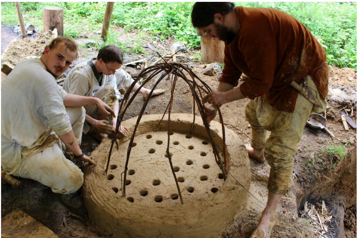
FIG 24. WEAVING WILLOW BRANCHES TO A SUPPORT CONSTRUCTION FOR THE DOMED FIRING CHAMBER.
