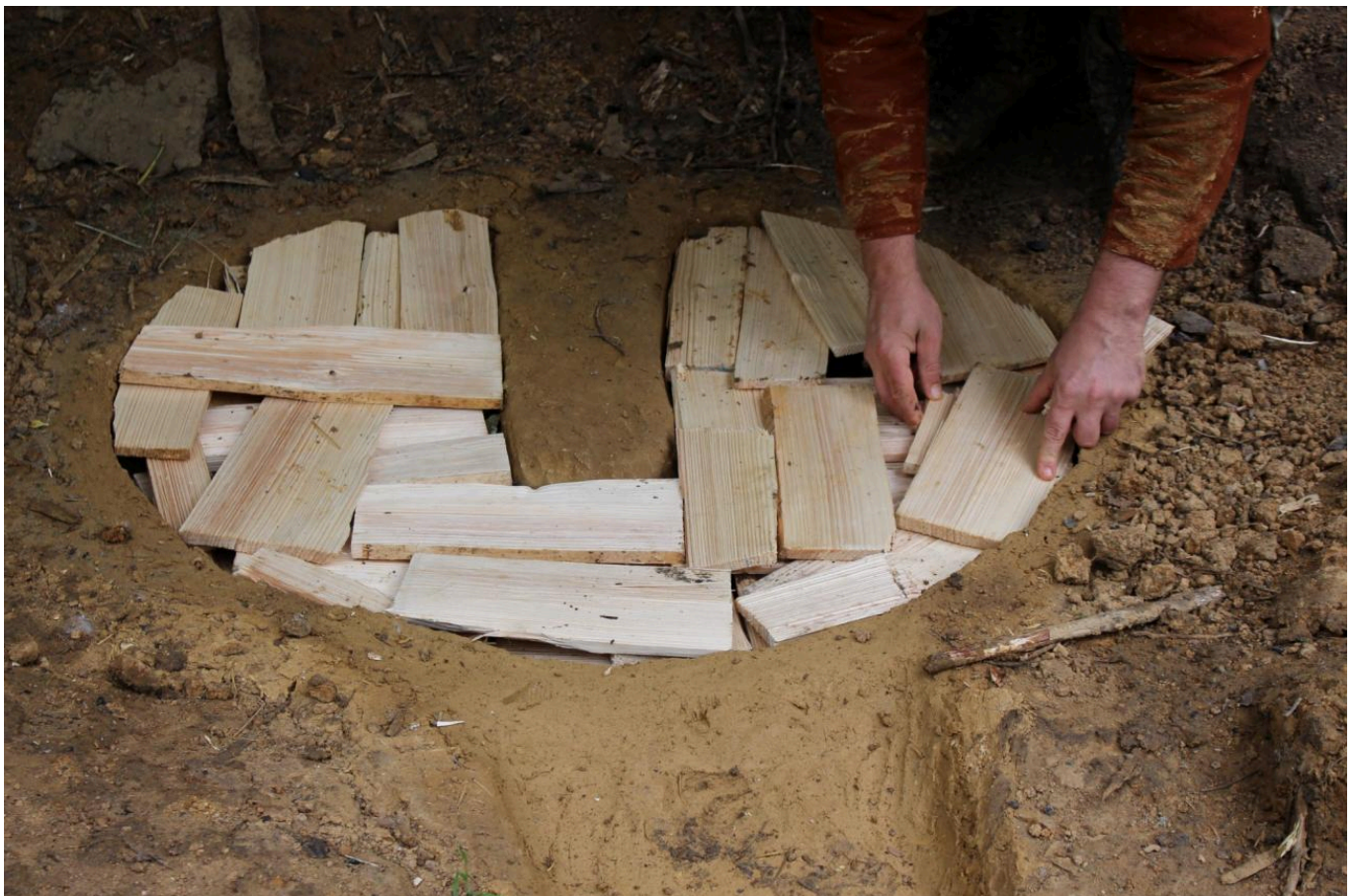
FIG 20. COMBUSTION CHAMBER WITH A RADIAL WALL AS A SUPPORT FOR THE RAISED FLOOR, AND FIRING TUNNEL, DURING THE CONSTRUCTION OF THE KILN.
