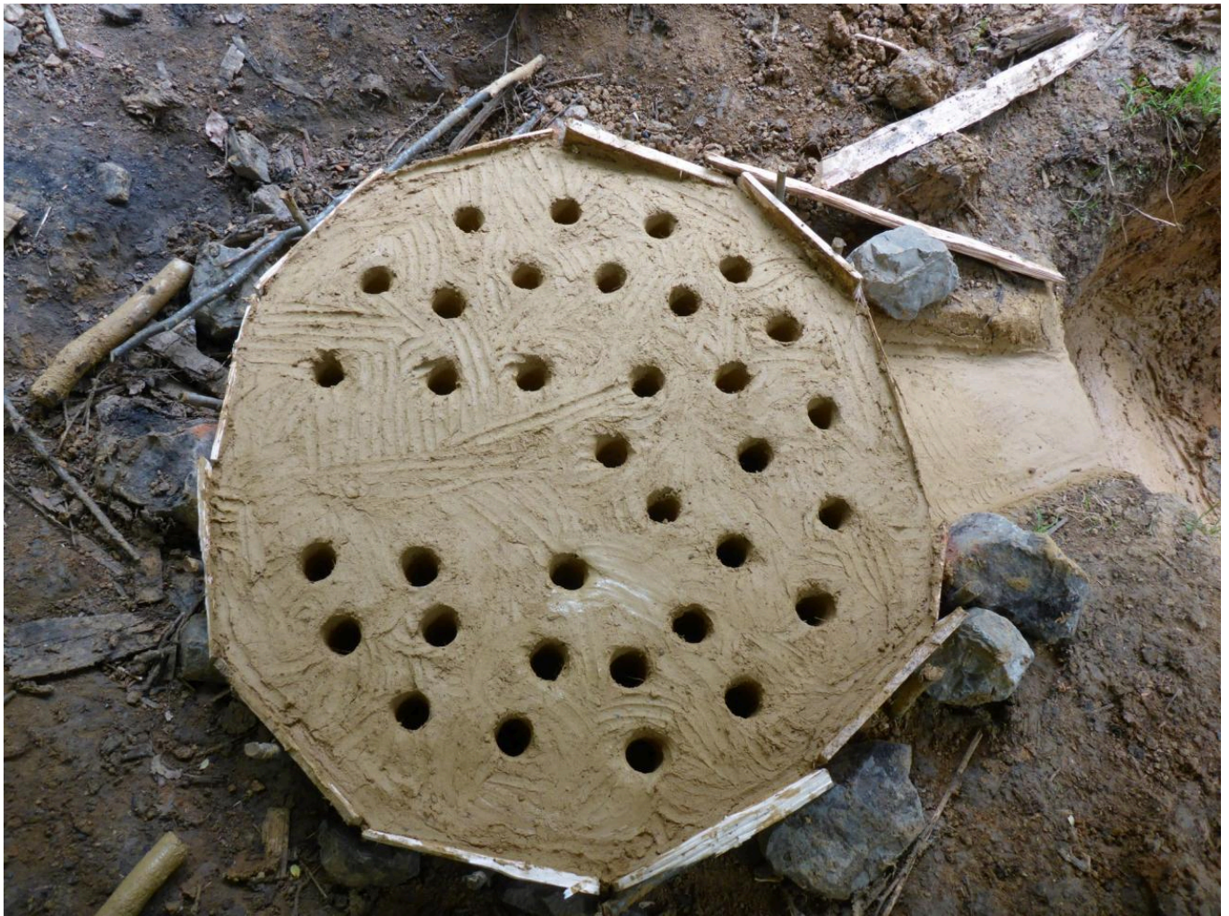
FIG 23. RAISED KILN FLOOR MADE OF COB, PERFORATED WITH VENTS, DURING THE CONSTRUCTION.
