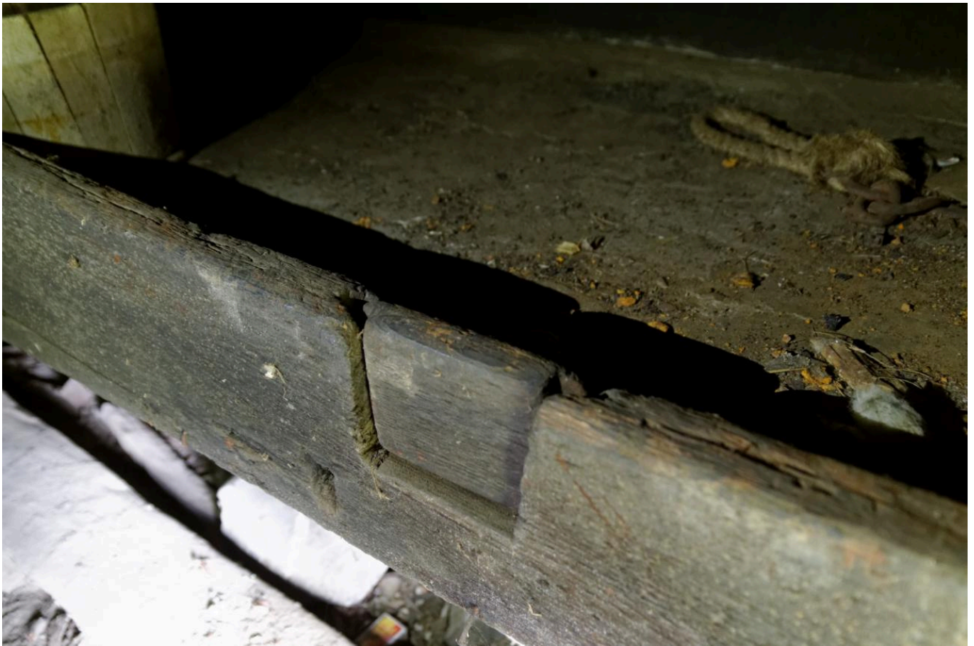
FIG 15. LITTLE 'GATE' FOR SCOOPING OUT THE MALT FROM THE SHELF. COPYRIGHTS BY LARS MARIUS GARSHOL. FOR MORE DETAILS SEE LARSBLOG HTTPS://WWW.GARSHOL.PRIV.NO
