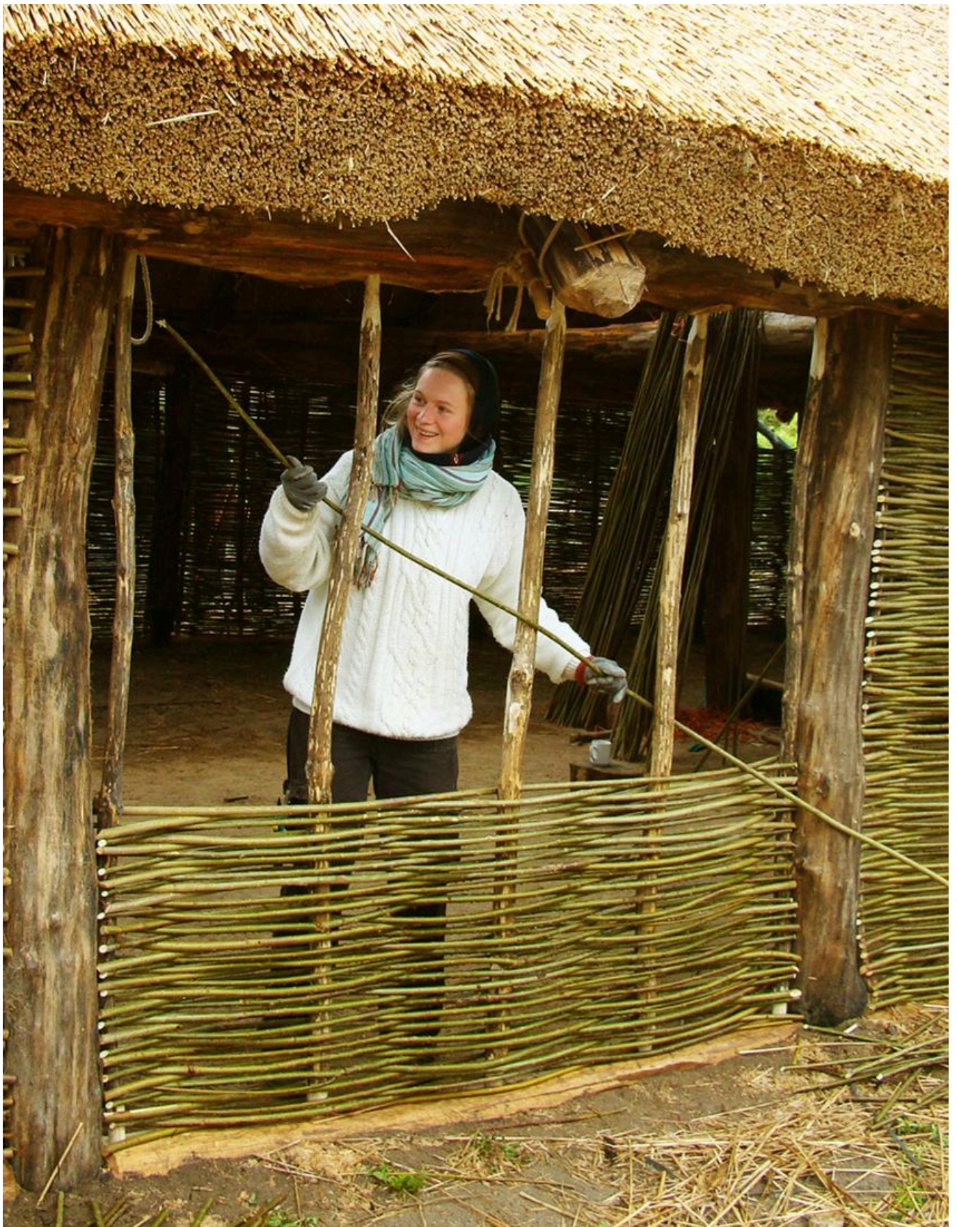
FIG 12. IN THE MIDDLE PART OF THE HOUSE THE WALL INFILLS WERE WOVEN WITH WILLOW RODS IN WATTLE AND DAUB STYLE. COPYRIGHT: WOLFGANG LOBISSER
