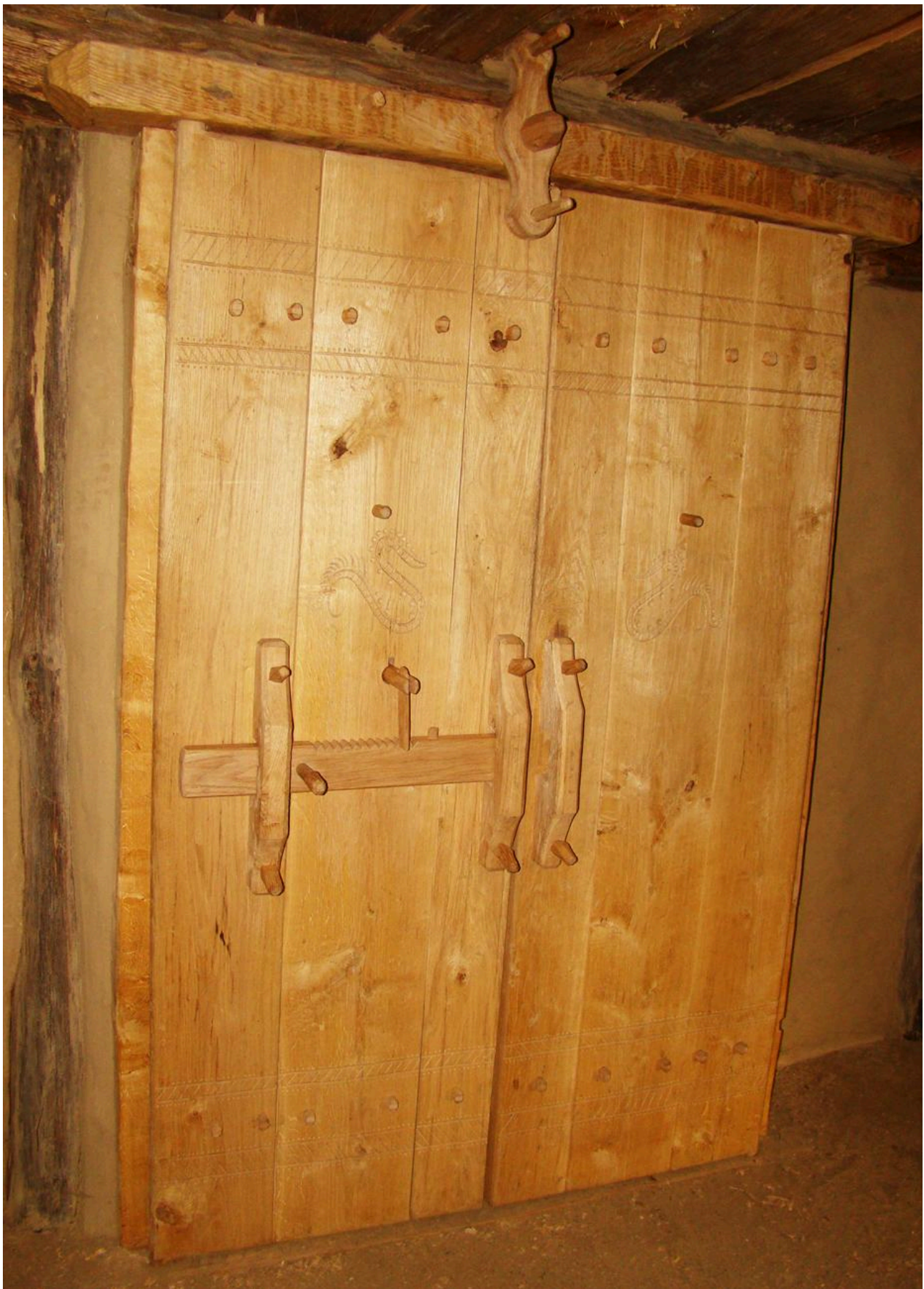
FIG 14. THE TWO LEAVES OF THE DOOR ARE MOUNTED IN A DOOR FRAME AND CAN BE LOCKED WITH A WOODEN BOLT MECHANISM. COPYRIGHT: WOLFGANG LOBISSER
