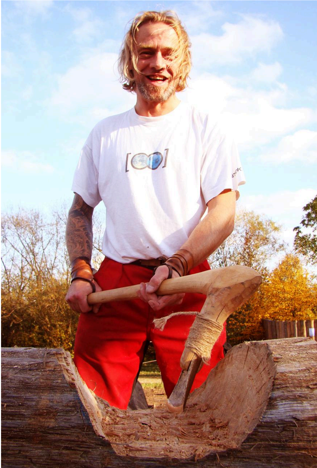
FIG 6. THE STRENGTHENING TRANSVERSAL ANCHOR BEAMS WERE FIXED ON THE EAVES BEAMS WITH SO CALLED SINGLE NOTCHED JOINTS; THE HALF ROUND RECESSES WERE HEWN OUT WITH HEAVY BRONZE AXES. COPYRIGHT: WOLFGANG LOBISSER
