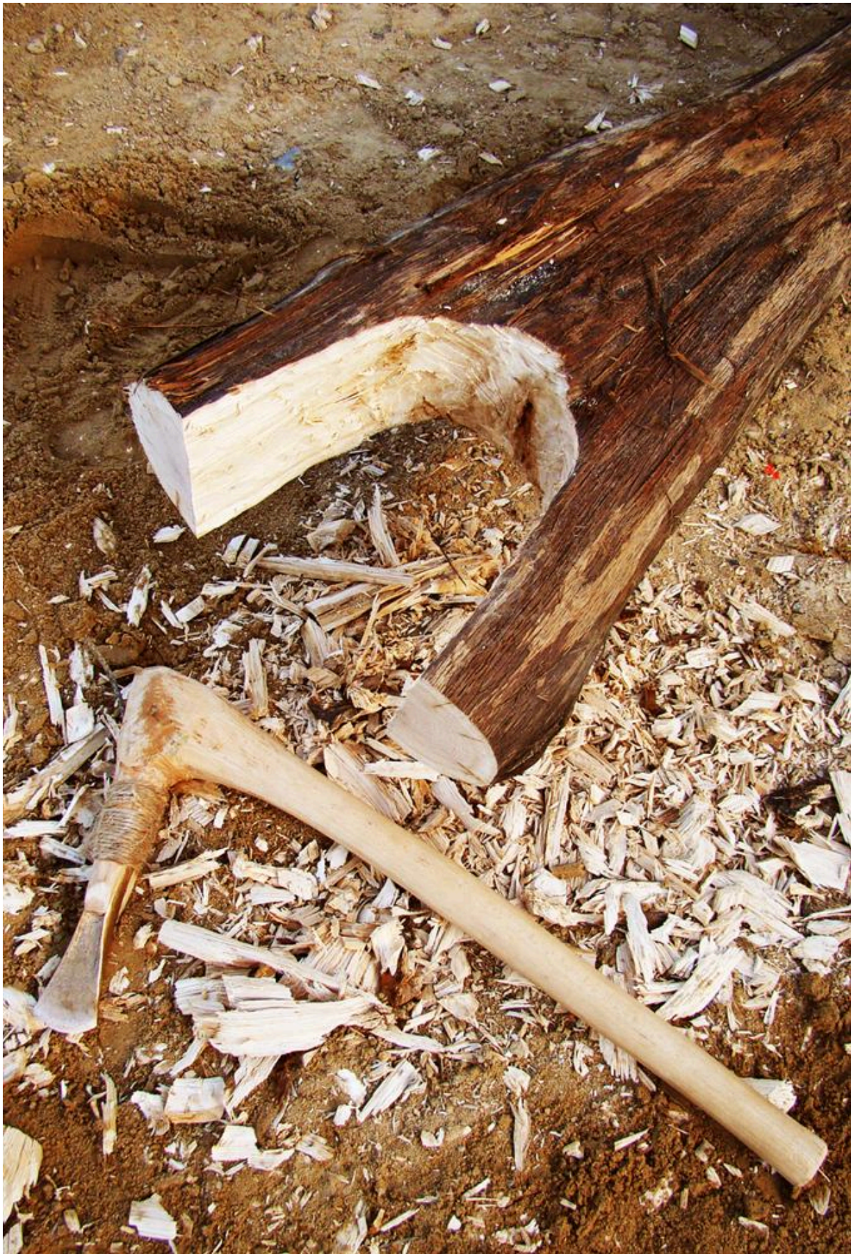
FIG 3. THE FORKED GROWN TAP ENDS OF THE EARTH FAST RIDGE POSTS WERE ADAPTED TO THE FORM OF THE PURLINS WITH BRONZE AGE AXES ATTACHED TO THE ANGLED HANDLES. COPYRIGHT: WOLFGANG LOBISSE
