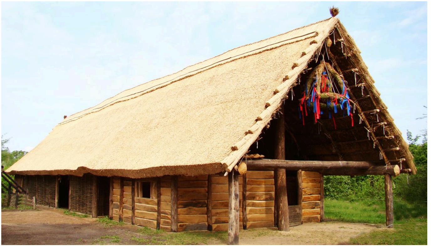
FIG 18. THE LONGHOUSE WITH THE ROOF FINISHED; IN THE EAST THERE IS AN OPEN BUT ROOFED ACTIVITY AREA; PLEASE NOTICE OUR SUGGESTION FOR A WINDOW IN THE OAK PLANK WALL. COPYRIGHT: WOLFGANG LOBISSER
