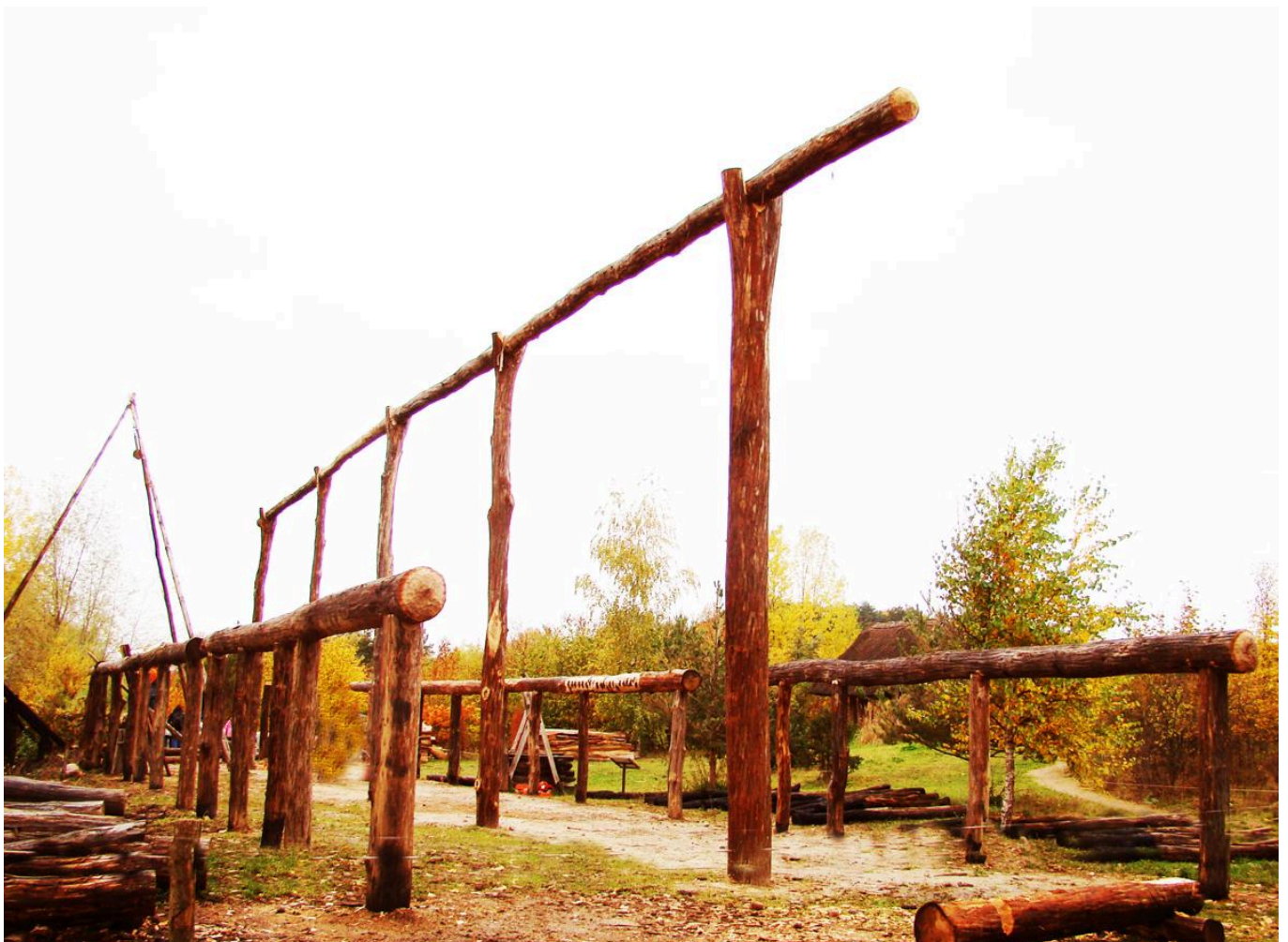
FIG 4. BRONZE CHISELS WERE WELL SUITED TO CARVE RECTANGULAR TENONS ON THE UPPER ENDS OF THE EXTERNAL WALL POSTS WHICH ALLOWED US TO PUT ON THE EAVES BEAMS. COPYRIGHT: WOLFGANG LOBISSE
