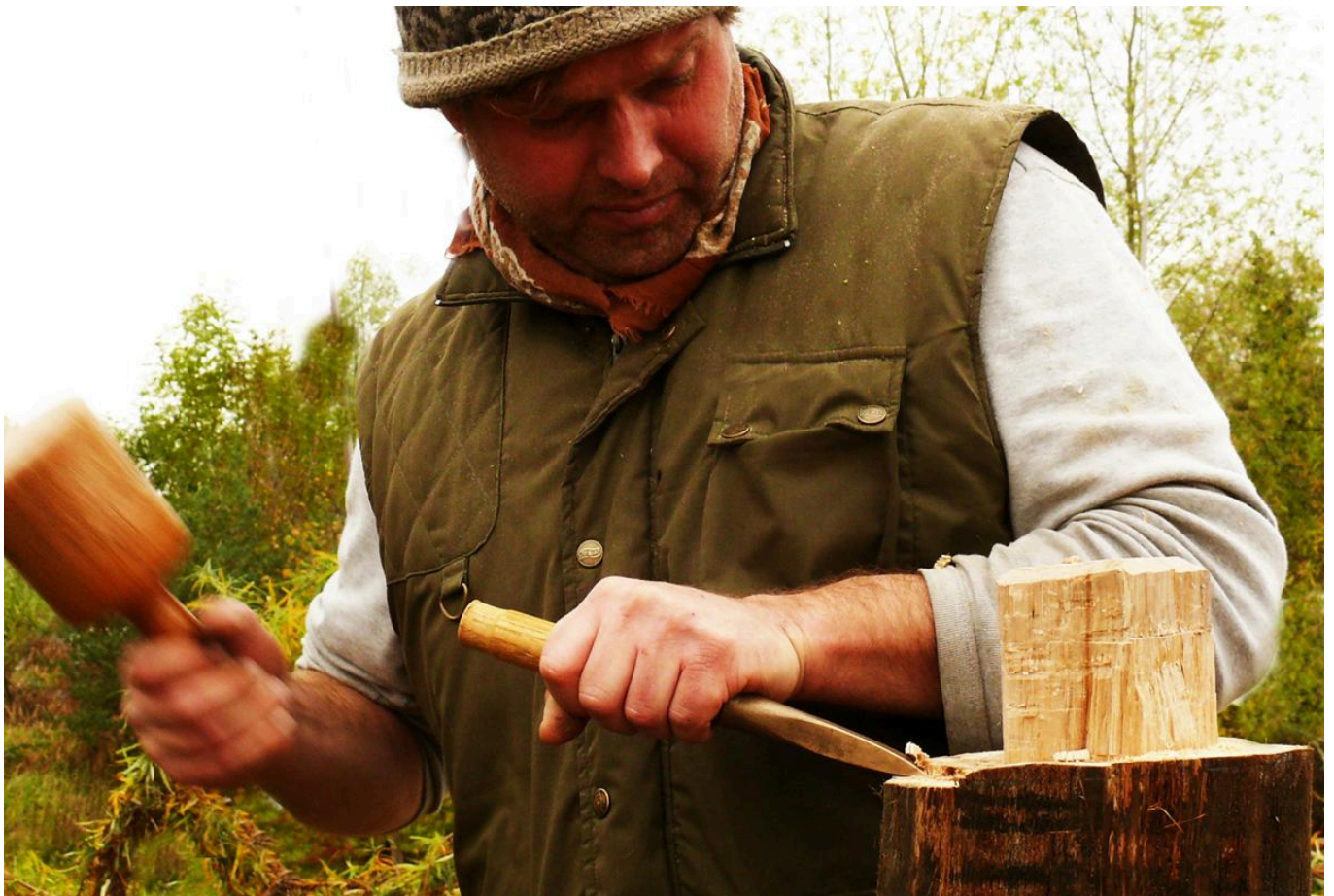
FIG 4. BRONZE CHISELS WERE WELL SUITED TO CARVE RECTANGULAR TENONS ON THE UPPER ENDS OF THE EXTERNAL WALL POSTS WHICH ALLOWED US TO PUT ON THE EAVES BEAMS. COPYRIGHT: WOLFGANG LOBISSE
