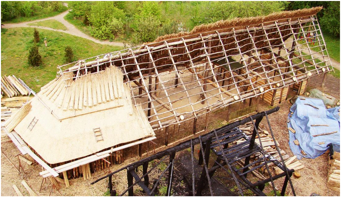
FIG 15. A BIRD'S-EYE VIEW DURING THE WORK ON THE REED ROOF. COPYRIGHT: WOLFGANG LOBISSER
