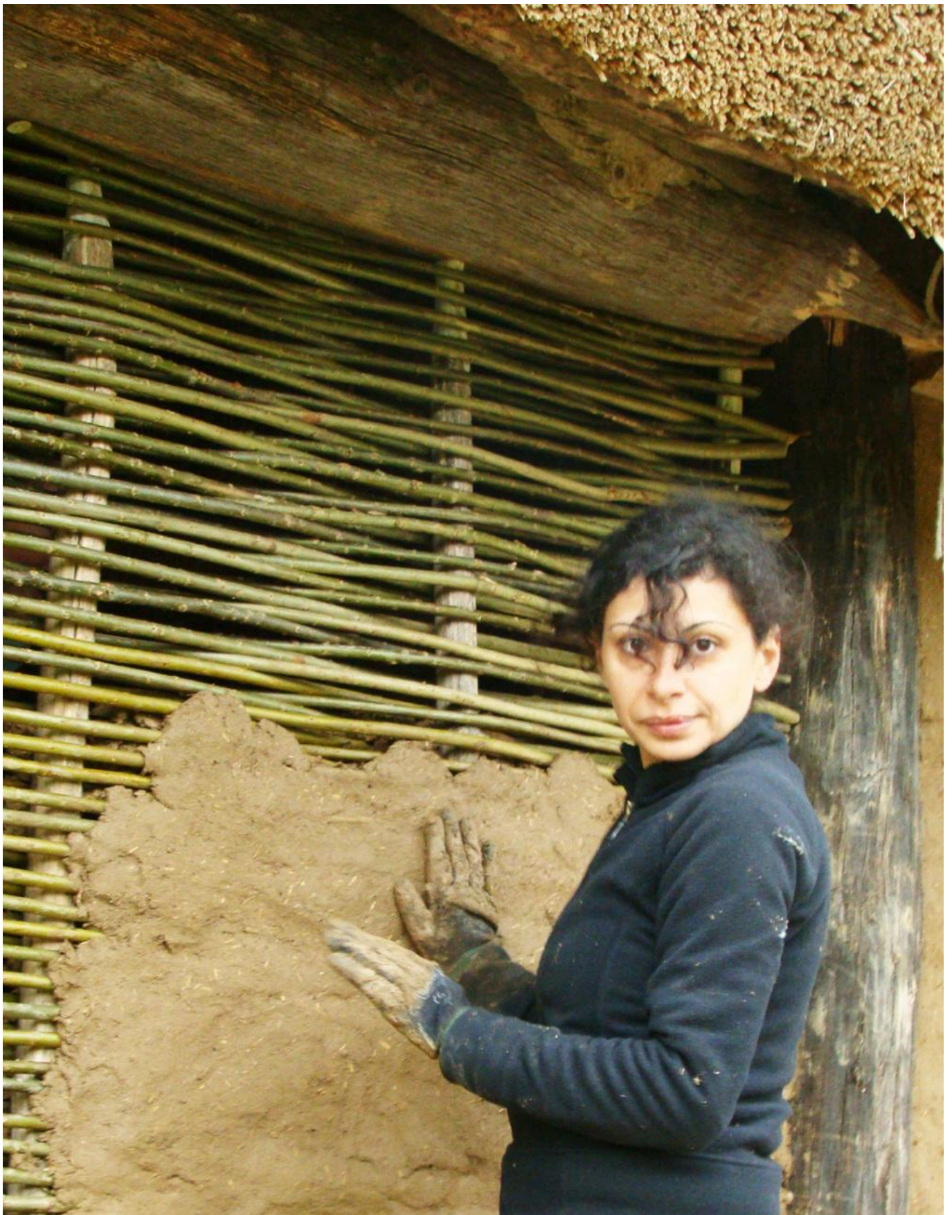
FIG 16. CONCERNING THE LOAM PLASTER WE USED DIFFERENT COMPOSITIONS OF CLAY AND DIFFERENT TECHNIQUES OF BRINGING UP THE LOAM TO THE WICKER WORK WALLS. COPYRIGHT: WOLFGANG LOBISSER
