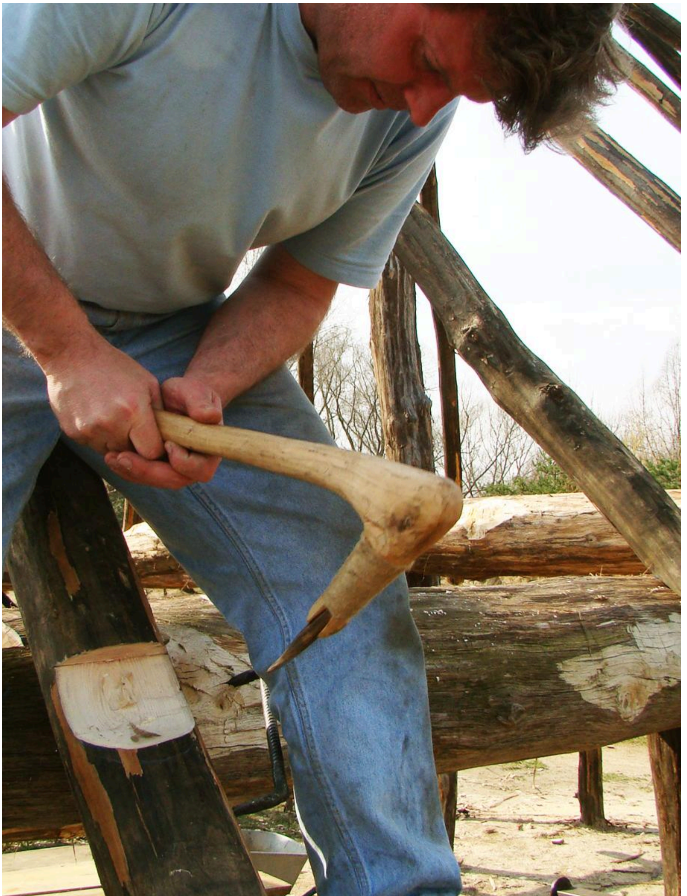
FIG 8. THE RAFTERS WERE FIXED ON THE EAVES BEAMS WITH SO CALLED BIRDSMOUTHED JOINTS, WHICH WERE WORKED OUT WITH BRONZE BLADES HAFTED AS ADZES. COPYRIGHT: WOLFGANG LOBISSER
