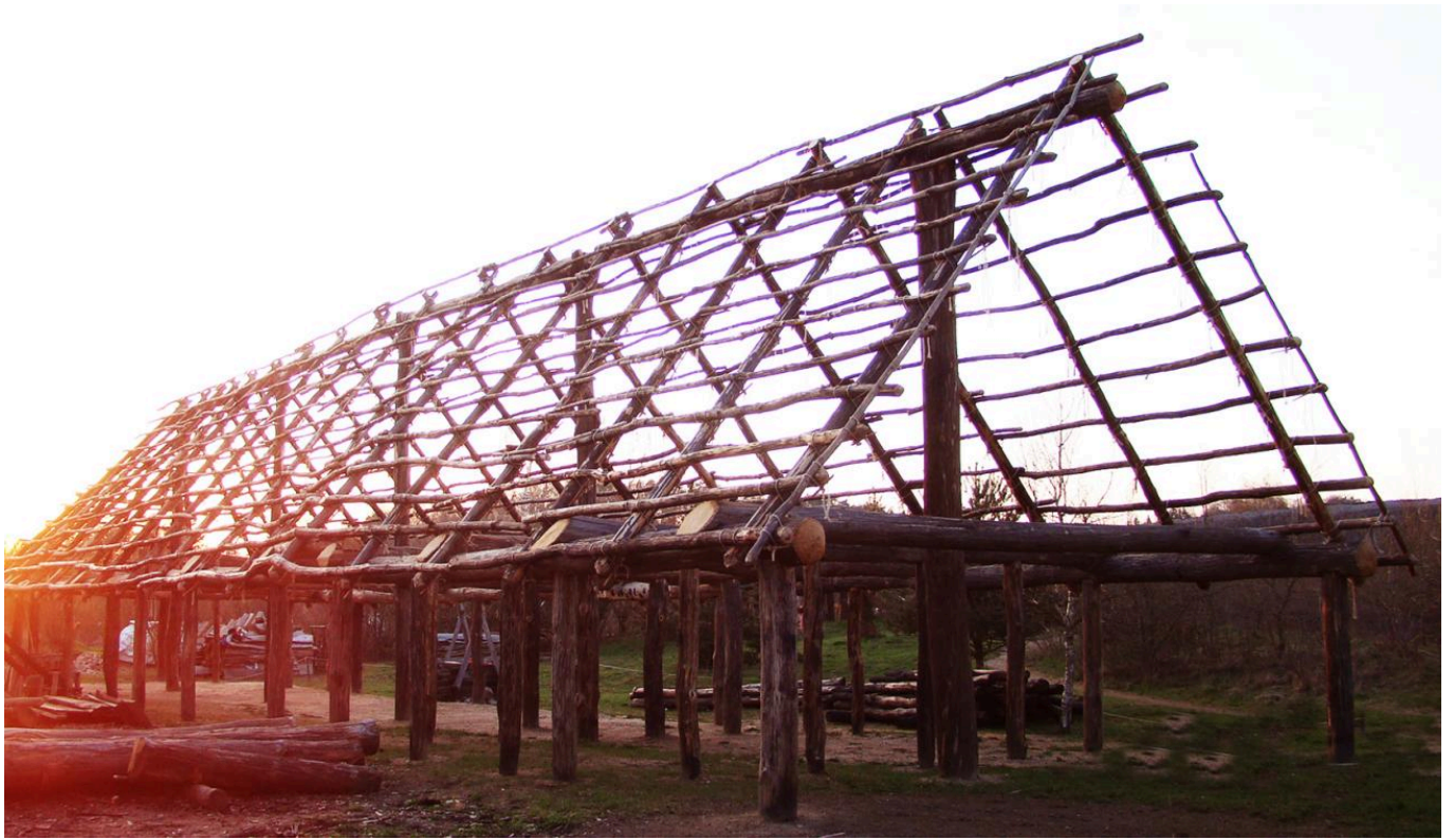
FIG 9. THE BATTENS WERE BOUND ON THE RAFTERS USING ROPE BINDINGS. COPYRIGHT: WOLFGANG LOBISSER
