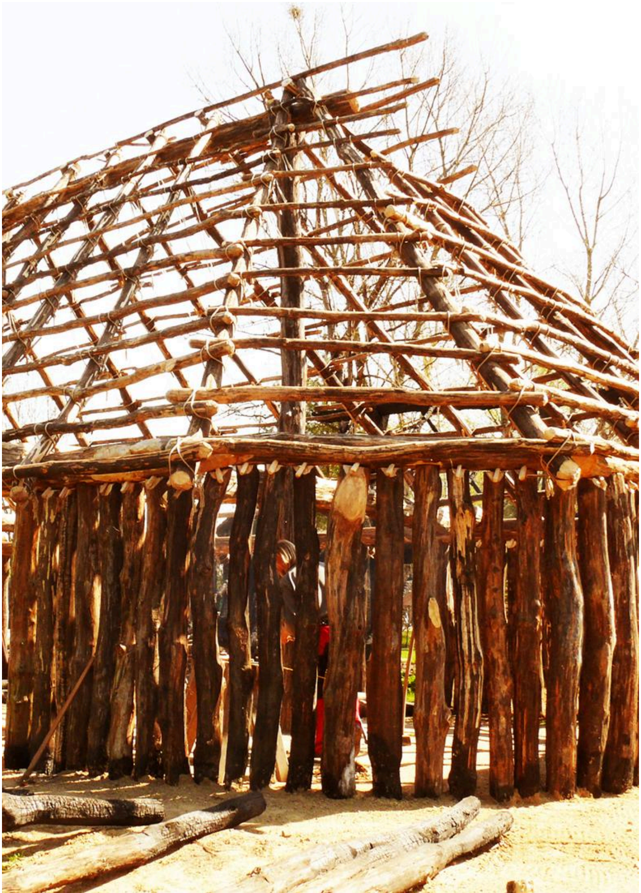
FIG 10. ACCORDING TO EXCAVATION DATA THE WALL AT THE WESTERN END OF THE HOUSE WAS CONSTRUCTED WITH VERTICAL ROUND LOGS; THE GAPS WERE FILLED WITH CLAY. COPYRIGHT: WOLFGANG LOBISSER
