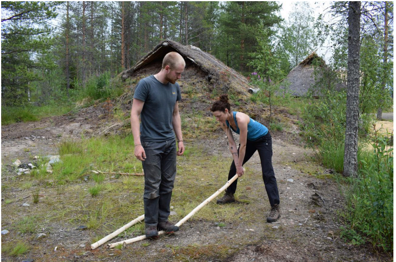
FIG 4B. SNAPPING THE TREE LENGTHS AT THE WEAK POINT. PHOTO BY JAMES FINDLAY
