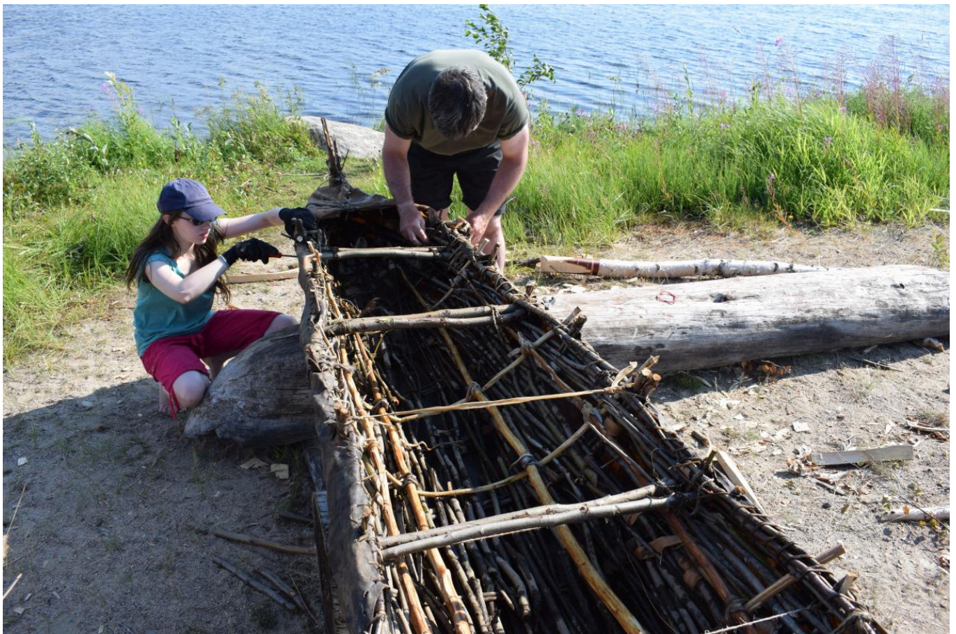
FIG 6. THE HIDES AT THE STERN BEING DOUBLE STITCHED TOGETHER USING THIN RAWHIDE LACING. PHOTOGRAPH JAMES FINDLAY.
