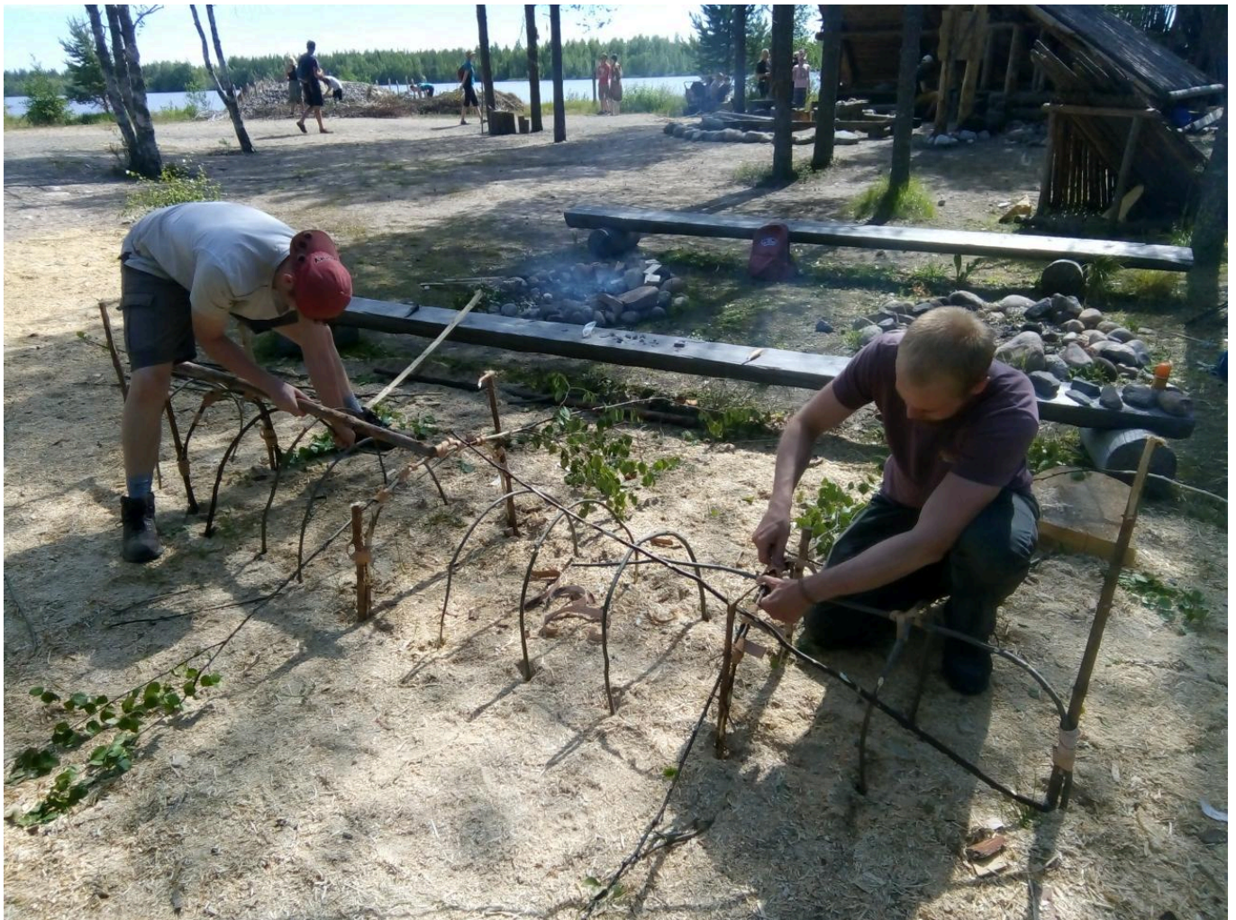
FIG 1. THE FIRST RIBS (HOOPS) OF THE CANOE BEING LASHED WITH BIRCH BARK. PHOTOGRAPH JAMES FINDLAY.
