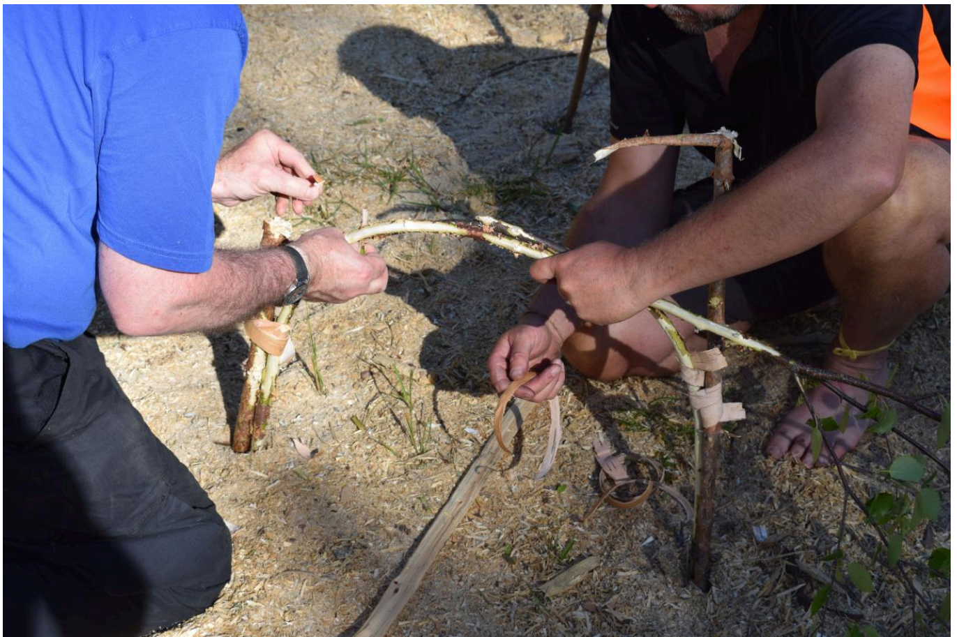
FIG 1. THE FIRST RIBS (HOOPS) OF THE CANOE BEING LASHED WITH BIRCH BARK. PHOTOGRAPH JAMES FINDLAY.
