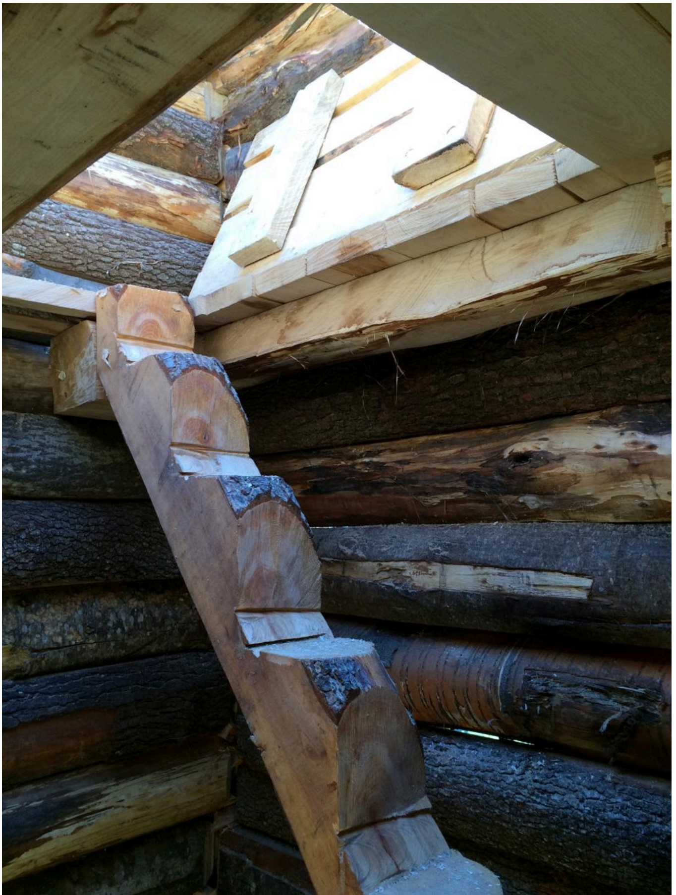
FIG 17. THE STEPLADDER MADE IN A TRUNK
