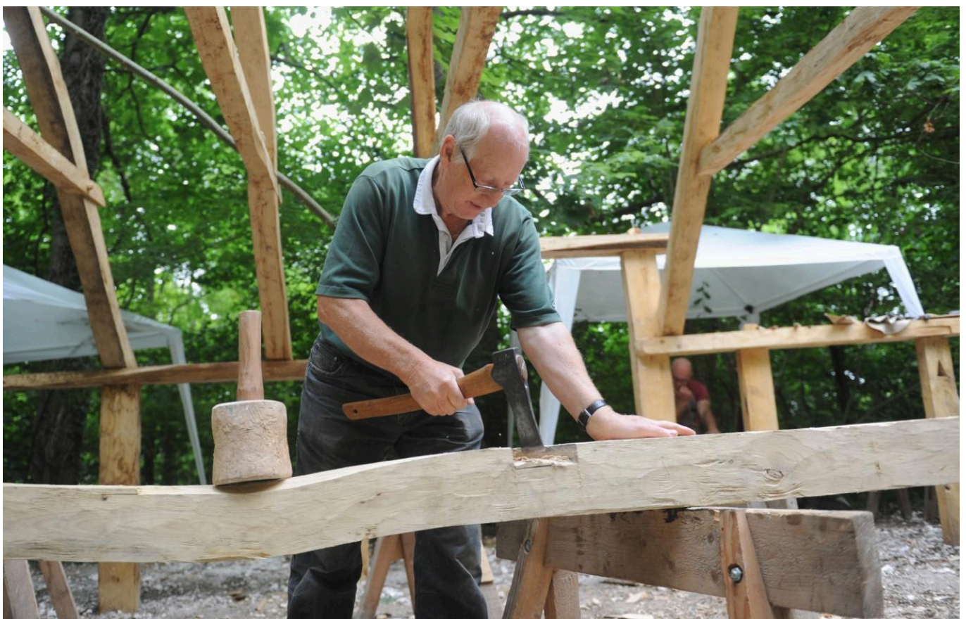
FIG 8. PHOTOGRAPH OF SOME OF THE TOOLS USED ON THE FRAME. PHOTO BY LOUISE ADAMS FOR WDLM
