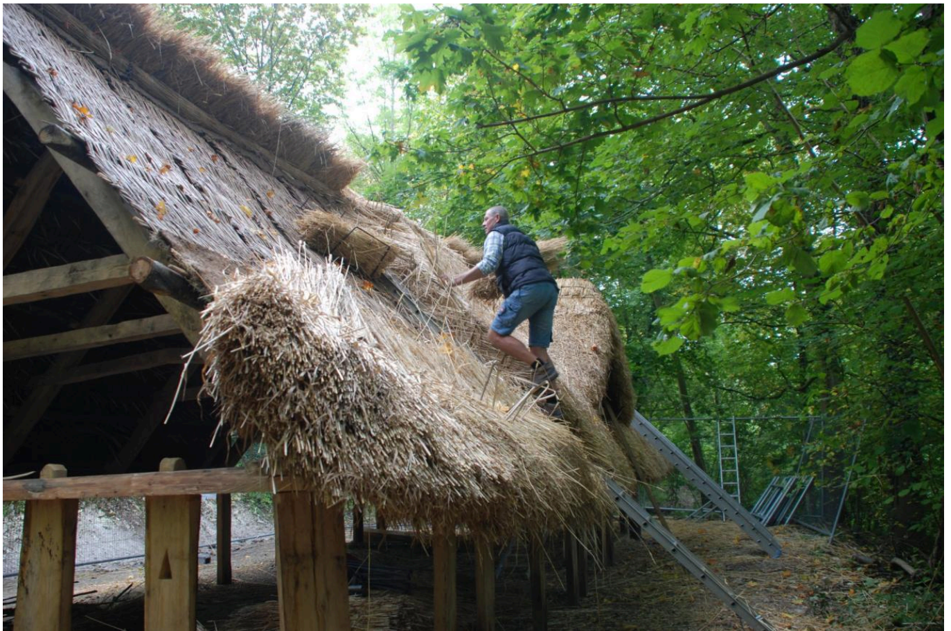
FIG 10. PHOTOGRAPH OF THATCHING OF THE SAXON HALL. COPYRIGHTS BY WDLM
