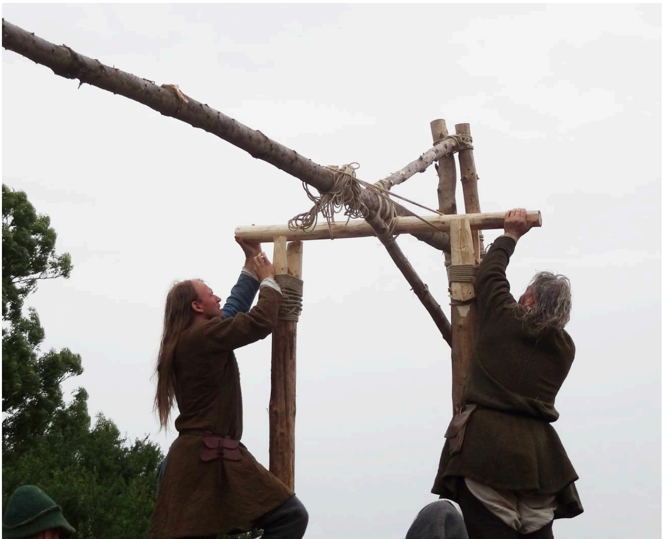
FIG 4. TEST PLACEMENT OF ARM TO CHECK ANGLES. ROPING HAS NOT BEEN COMPLETED. MIDDELALDERCENTERET NYKØBING FALSTER 2017
