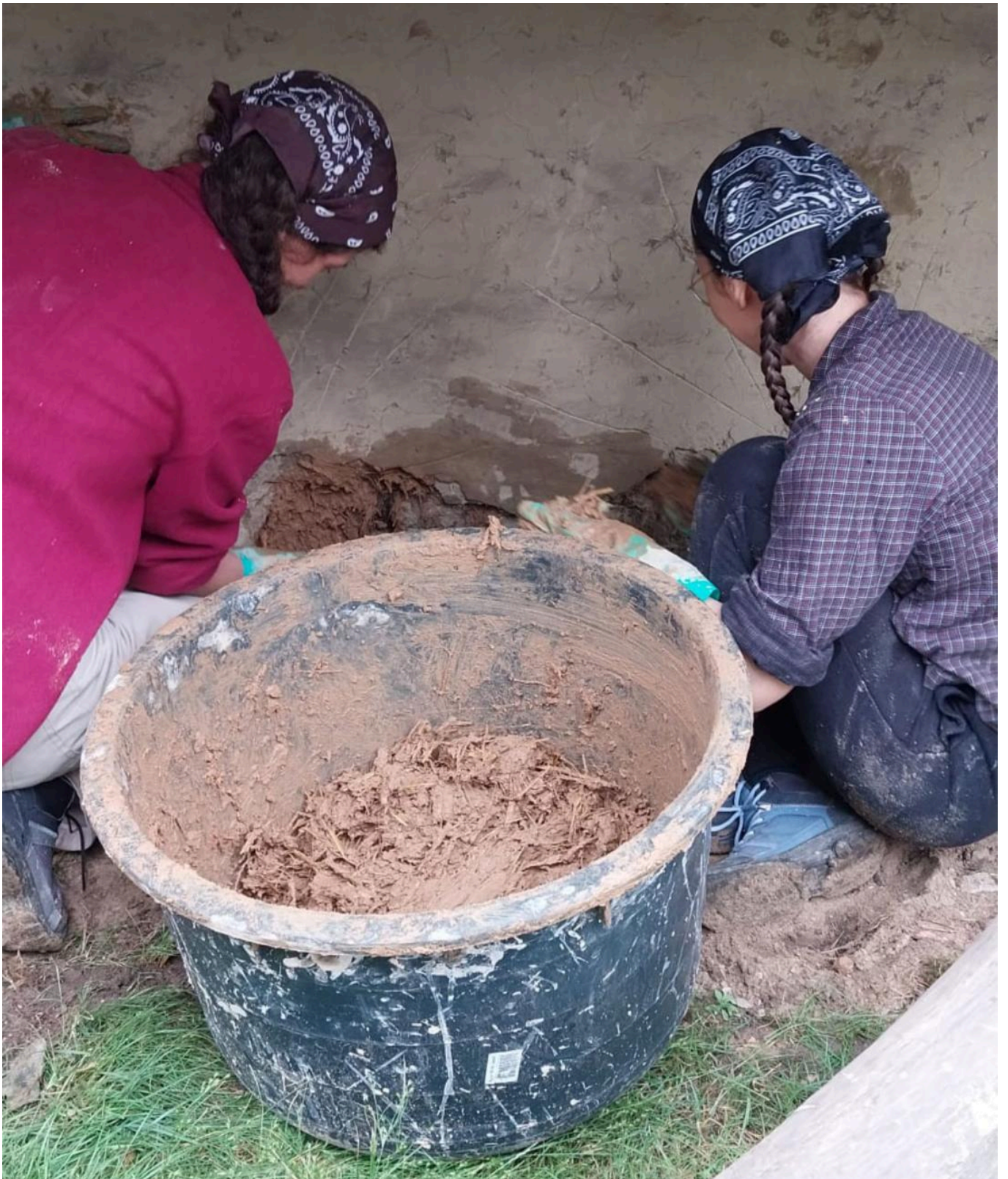
FIG 5. WORK IN PROGRESS. PHOTO BY AUTHORS
