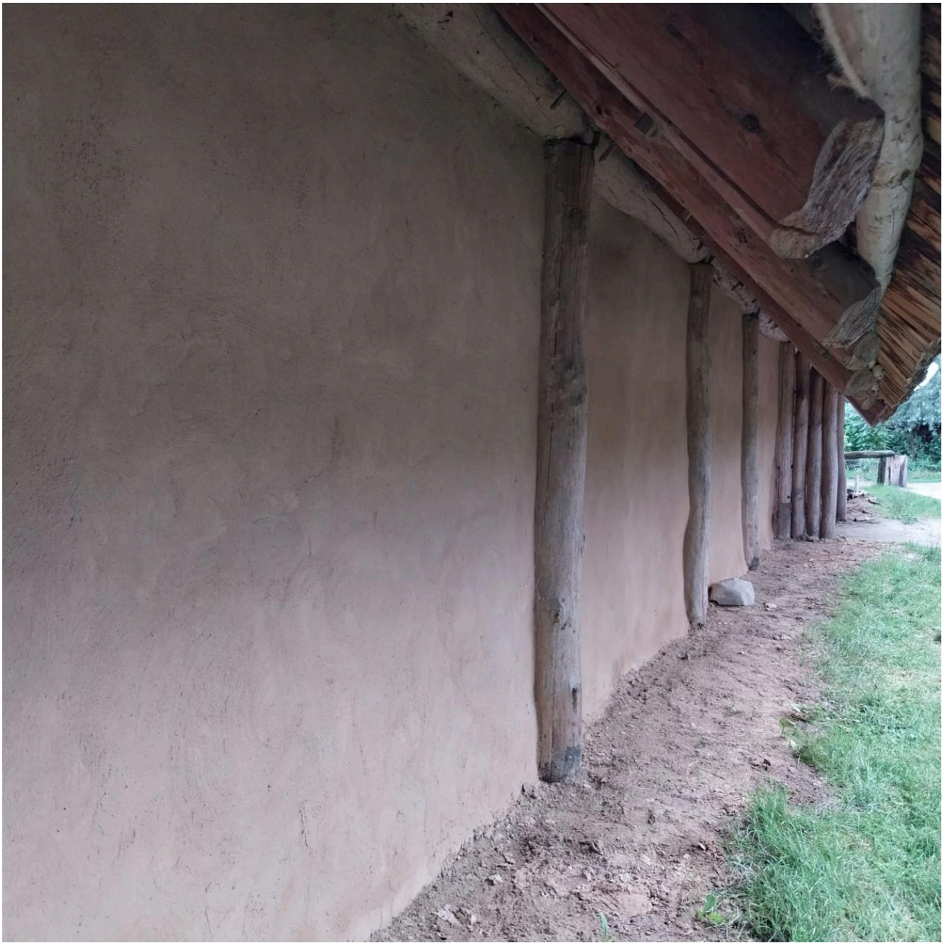
FIG 8. WALL OF THE ROMAN BUILDING AFTER THE "THE CLAY GIRLS". PHOTO BY AUTHORS
