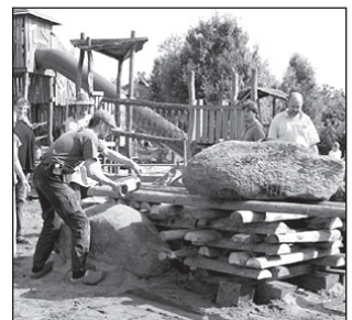
■ Picture D Greasing the rails before final placement
