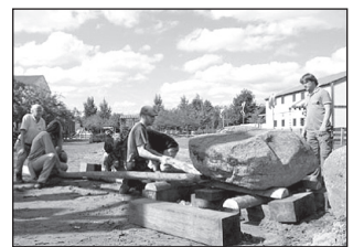
■ Picture C Lifting the stone with levers to put wooden logs under it
